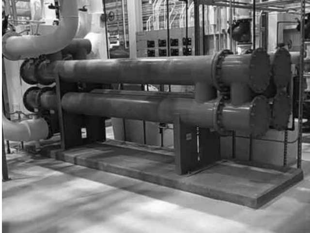
FIGURE 14.1 Typical shell-and-tube heat exchanger. (Courtesy of the Baltimore Aircoil Company, Baltimore, MD.)
