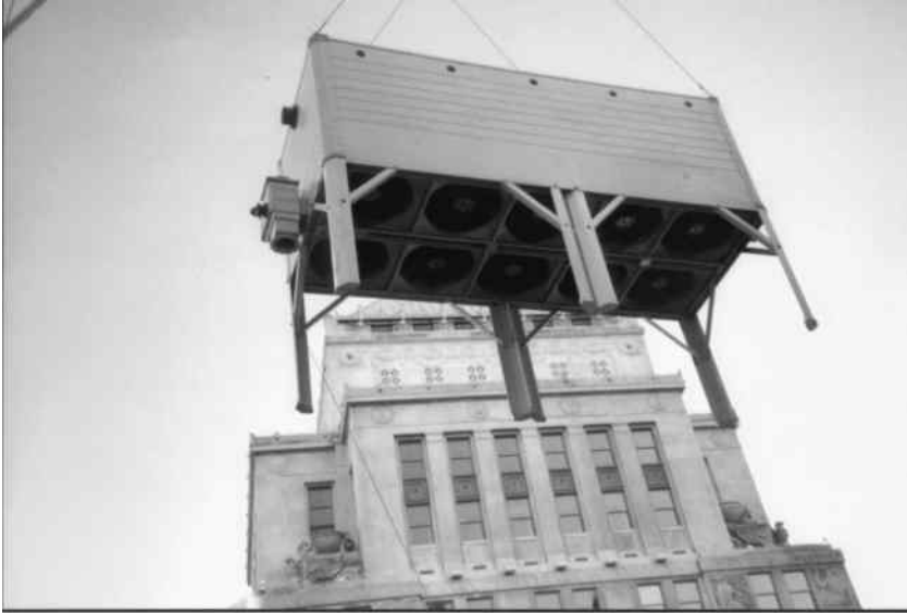
FIGURE 11.3 Typical forced draft counterflow cooling tower. (Courtesy of Tower Tech, Inc., Oklahoma City, OK.)
