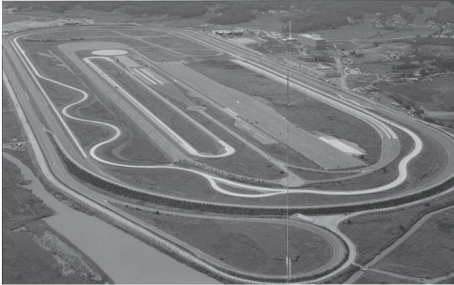
Figure 15.9 View of Hyundai Research Centre at Namyang
