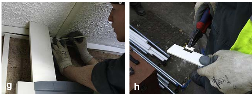
(g) The trunking lid is marked out for cutting. (h) After screwing the trunking in position, the lid is cut to suit. In this case a notch needs to be removed to clear an existing trunking run. The lid is notched using a saw and pliers used to remove the notch.
