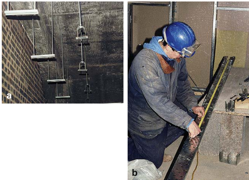
(a) Supports appropriate for the installation are first fitted. Here ceiling supports to carry cable tray and trunking above a suspended ceiling can be seen. (b) The length of tray required is measured and marked off, ready for cutting.
