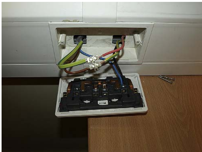
FIGURE 16.1 The test for continuity involves using a bridging strap connected between the line conductor and the relevant earth connection related to the particular circuit, here conveniently applied at a socket outlet.
