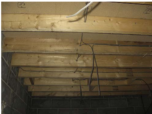
FIGURE 13.5 During building construction, it is possible to gain access to joists from either above or below. Here the upper floor has been laid but access for wiring is still possible from below. Joists have been bored and cable runs made prior to the ceiling being fitted (NBK Electrical).
