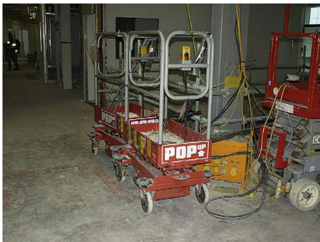
FIGURE 1.3 Battery powered re-chargeable working platforms in use in a new building greatly help in carrying out installation work at heights. The units are stable on level ground, have protection devices fitted and can easily be set by the operator to the most convenient working height (M.W. Cripwell Ltd).
