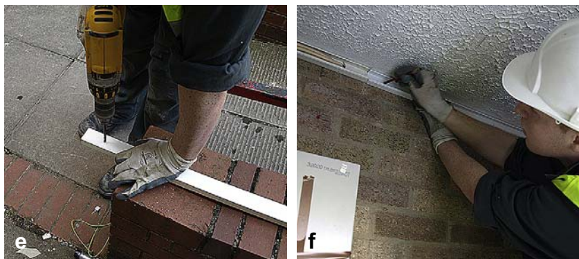
(e) Fixing holes are required and these are next drilled at suitable positions. (f) After drilling the conduit, the wall is correspondingly marked out and drilled for wall plugs.
