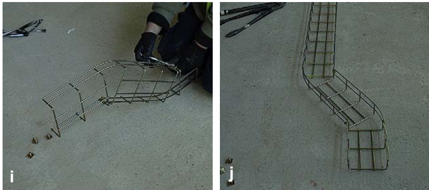
(i) Once the side and bottom elements have been cut, the bend can be made and secured with the bolted clips. (j) The completed offset, ready for erection overhead into the third basket run.
