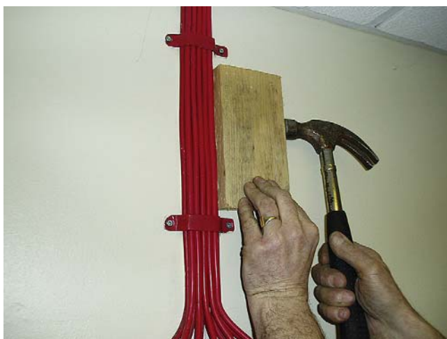
FIGURE 14.2 Straightening up multiple runs of MI cable using a block of wood and hammer (Wrexham Mineral Cables).
