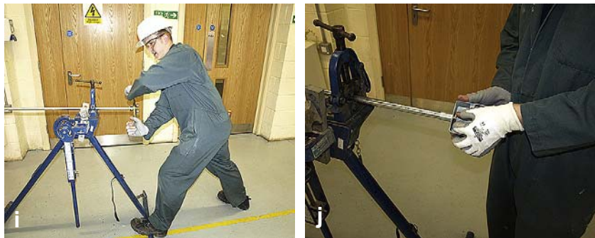
(i) Using a set of dies and a die holder, the conduit is threaded ready of the outlet bush. Application of a thread cutting lubricant aids this process. (j) After the coupler is secured, the outlet box is attached using a brass bush.
