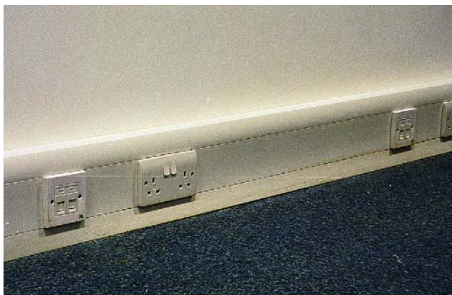
FIGURE 10.4 Multi-compartment skirting trunking allows the segregation of different types of circuit. In this example 13 A ring main socket outlets and telecommunications circuits are provided (W.T. Parker Ltd).
