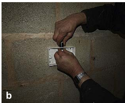
(a) The conduit can easily be cut to length with the special cutters obtainable for the purpose. (b) A range of fittings is available including boxes, bends, saddles and bushes. Here a bush is being secured using a threaded ring.
