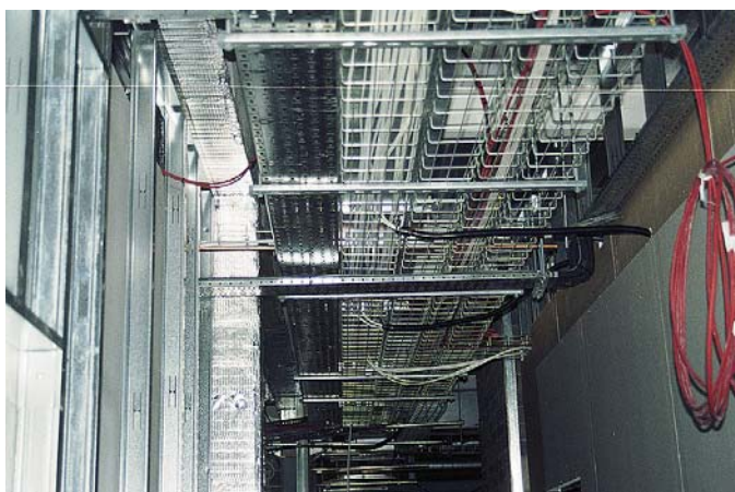
FIGURE 8.4 A high-level cable route in an industrial building is illustrated in this view. Cable ladder is provided to carry distribution cables feeding switchboards remote from the site sub-station. Cable basket, which in this case has three separate compartments, is to be used for data cabling and cable tray is provided for final circuits feeding lighting and machinery (W.T. Parker Ltd).
