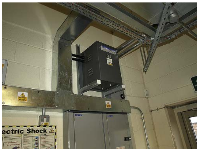
FIGURE 2.5 An isolating transformer supplying extra-low voltage socket outlets for use of portable tools in an industrial installation.
