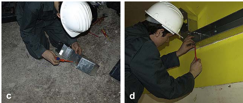
(c) Fitting the components of the offset together using set screws inserted into the pre-tapped holes in the angle pieces. (d) Having fitted the long runs of 100×100mm conduit to the wall, the offset is assembled in position.
