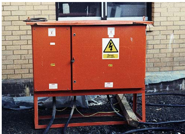
FIGURE 7.2 Load centre for a temporary installation on a construction site (William Steward & Co).
