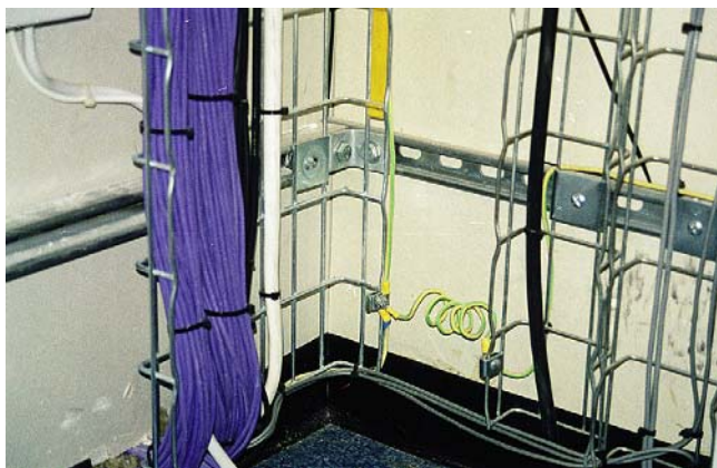
FIGURE 4.5 A commercial location where a cable riser is constructed from cable basket and carries cables for different types of circuits. Note the equipotential bonding conductors (W.T. Parker Ltd).
