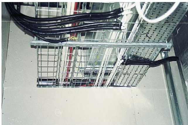
FIGURE 12.2 Cable runs fitted in the roof space above a suspended ceiling. Multi-compartment cable basket is provided, as well as cable tray for different circuit categories. Note the copex flexible conduits which carry feeds to specific locations (W.T. Parker Ltd).
