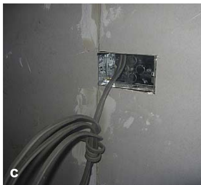
(c) After the wall surface is complete, the cables can be stripped and socket outlets, spur boxes and other accessories fitted to complete the installation (all NBK Electrical).
