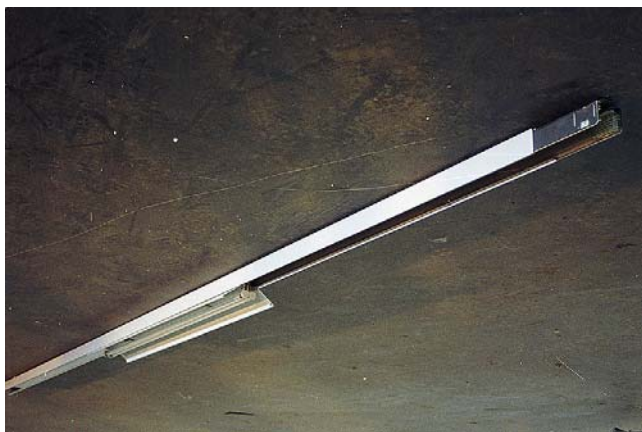
FIGURE 11.1 This type of lighting trunking has integral busbars carrying conductors for the supply to the luminaires. The 54-W twin fittings are available with either wide angle or semi-specular narrow beam characteristics, enabling effective lighting from different heights. The trunking can be suspended from the building frame and, with the narrow beam reflectors, is suitable for high-bay illumination. The clip-in fittings can be arranged to pick up from different phases and the whole assembly can be carried out without the use of tools, a particular advantage when working at heights (W.T. Parker Ltd).
