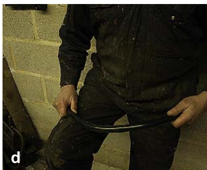
(c) Jointing is carried out by the use of solvent adhesives, and care must be taken in their application to avoid blocking small-sized conduits. (d) Bending can be by hand and a bending spring is used to retain the shape of the bore. In cold conditions, the conduit should be warmed before being bent through an angle slightly greater than that required. It is then returned to the right angle generally needed for bends.
