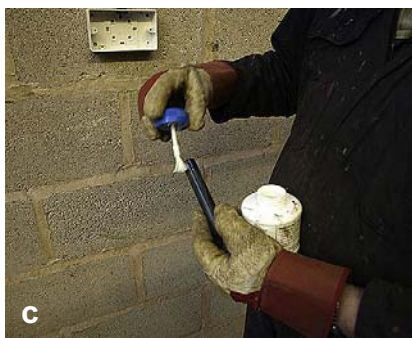
(c) Jointing is carried out by the use of solvent adhesives, and care must be taken in their application to avoid blocking small-sized conduits. (d) Bending can be by hand and a bending spring is used to retain the shape of the bore. In cold conditions, the conduit should be warmed before being bent through an angle slightly greater than that required. It is then returned to the right angle generally needed for bends.
