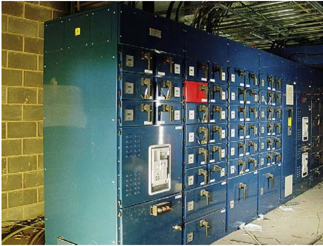
FIGURE 5.3 A switchboard for use in an industrial premises. The board incorporates over 60 outgoing switches as well as main ACBs, bus-section switches and metering facilities (Pandelco Ltd).
