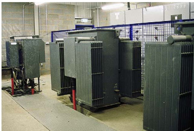
FIGURE 5.1 Main transformers in a factory building. Incoming supplies are from an 11kV ring main and feed two 800kVA, 11kV to 415V transformers. The distribution board in the sub-station use four-pole 1600A ACBs set at 1200A and a four-pole bus coupler rated at 2000A (W.T. Parker Ltd).
