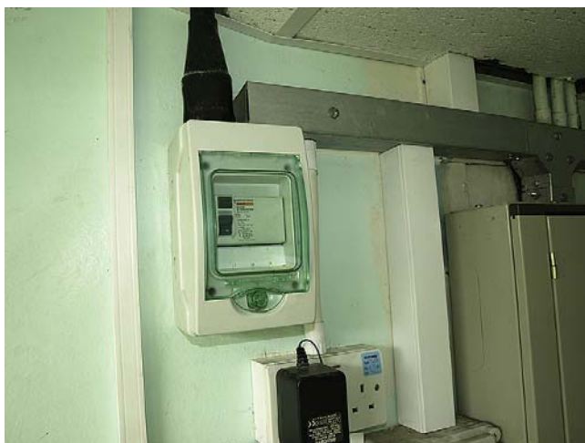
FIGURE 5.10 A 63-A RCCB with a 30-mA tripping current is fitted in a school and protects specific parts of the installation.
