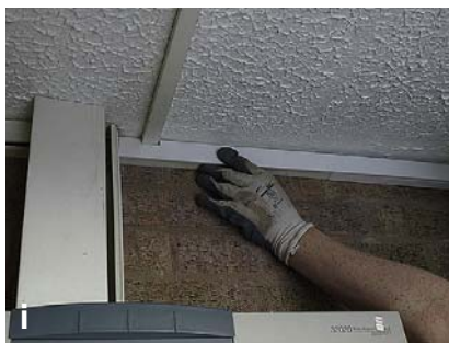
(i) The lid is fitted, the completed trunking gives a neat and workmanlike appearance (all M.W. Cripwell Ltd).
