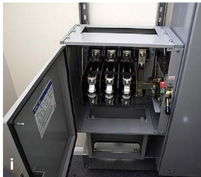
FIGURE 12.1 cont'd. Installation of main incoming switch.
