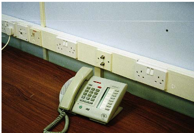
FIGURE 10.5 A typical office installation where data, telecommunication and power circuits are required (W.T. Parker Ltd).
