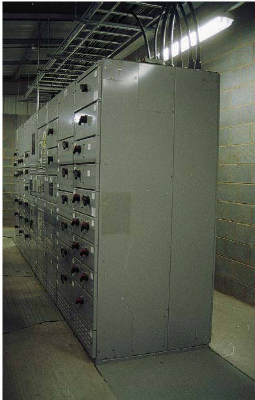
FIGURE 2.6 IEE Regulation 513 requires that every item of equipment be arranged so as to facilitate its operation, inspection and maintenance. This switchboard is installed in a room provided for the purpose, with access space both in front and behind the equipment. This situation will allow access for proper maintenance (W.T. Parker Ltd).
