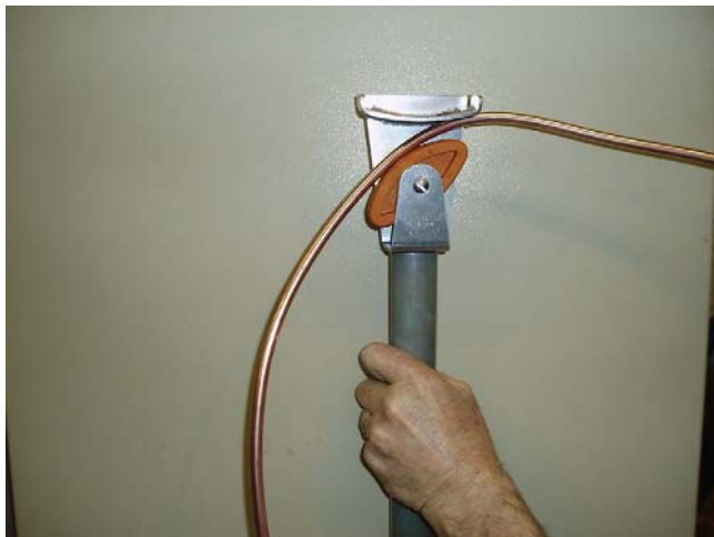
FIGURE 14.3 Bending and setting of MI cable. These operations can be more easily done by means of the simple tool illustrated (Wrexham Mineral Cables).
