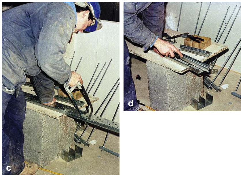
(c) The cable tray is cut using a hacksaw. (d) Using a file, burrs are removed to prevent damage to cables.
