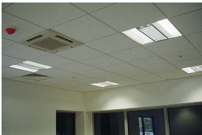
FIGURE 15.4 Suspended ceilings are regularly encountered in commercial premises. The matrix is designed to accept air conditioning, fire detection and lighting fittings, as seen in this view. The luminaires are Dextra compact fluorescent fittings with reflectors which give indirect as well as direct illumination (W.T. Parker Ltd).
