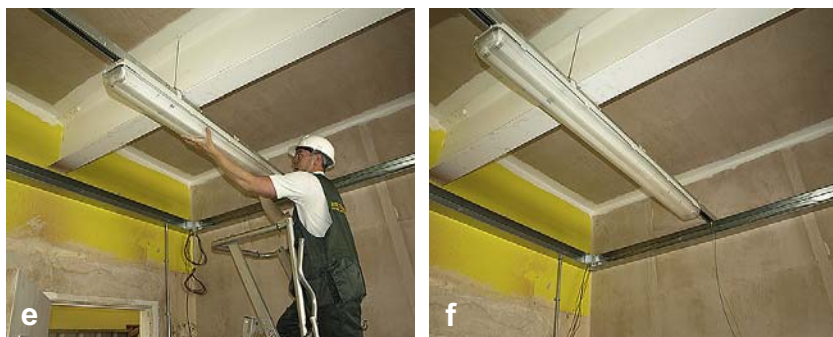
FIGURE 15.3 Installing a fluorescent lighting fitting.
