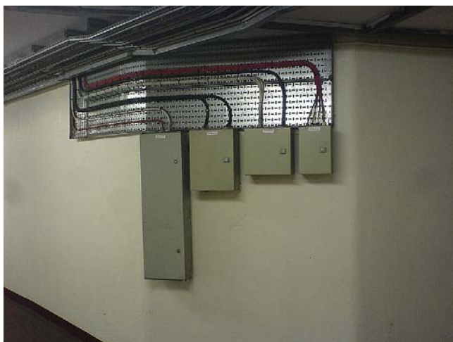
FIGURE 8.3 This neat installation shows cable tray with PVC and FP cable systems used to good advantage in a distribution area.
