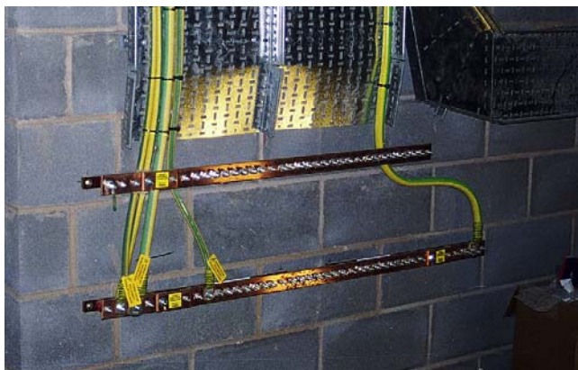
FIGURE 4.7 The main earth terminal in an industrial earthing location. The connections are located where inspection can readily be checked (W.T. Parker Ltd).
