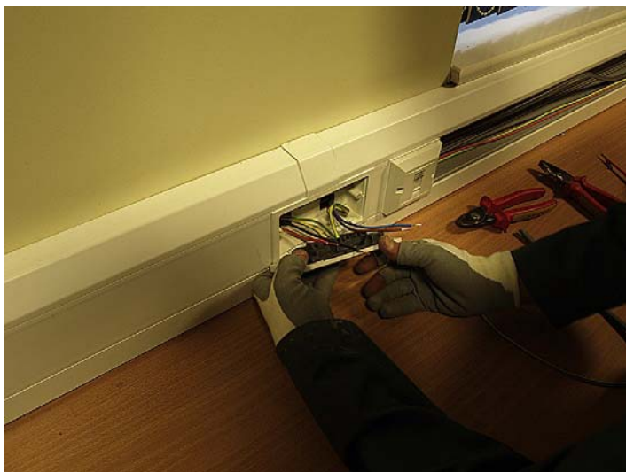
FIGURE 8.7 An extension to this installation will result in a mixture of colours from the old and current standards. A warning notice will need to be displayed (M.W. Cripwell Ltd).
