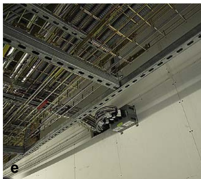
(e) The junction box and cable basket enable a neat installation to be made and one where fault finding and alterations are easily accommodated at a later date. (f) Modular units installed in a wall partition. Sufficient spare cable is arranged to enable the fitting of switch and socket units and to carry out changes should these be needed at a later date (all M.W. Cripwell Ltd).
