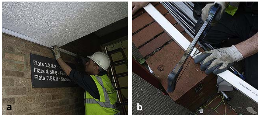
(a) The mini-trunking is offered up on site and marked to indicate the location of the bend. (b) Using a fine-tooth hacksaw, the conduit is cut at the back and on one side to suit the angle of bend required.
