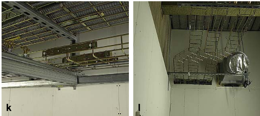
(k) In-line joints may be bolted or clipped. In this view, the clipped joining strips are seen. (l) The completed set of three parallel runs of cable basket, with suitable openings cut in the partition and offset to allow for the later erection of the ventilation ducting.
