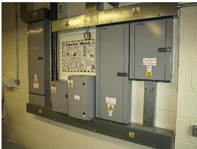
FIGURE 5.8 A distribution board in use in a college premises. The board incorporates three MCB distribution panels and associated switches. The installation is neatly wired in steel trunking and on cable tray.
