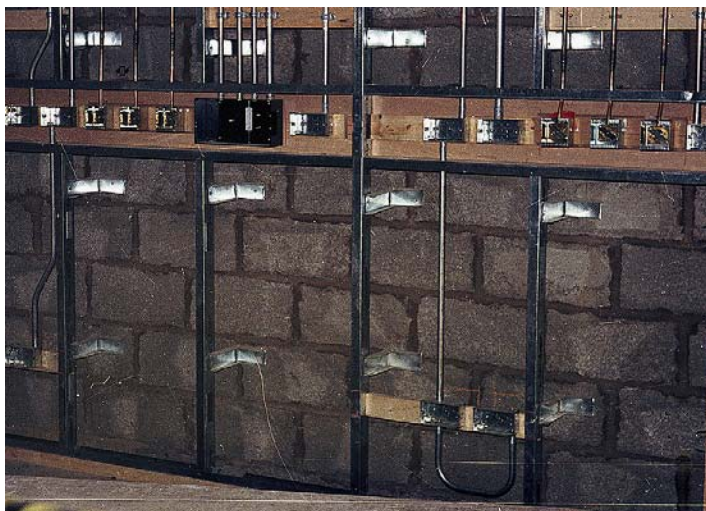
FIGURE 9.21 A neat completed conduit installation, ready for wiring to be installed (William Steward & Co. Ltd).
