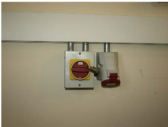
FIGURE 1.2 To comply with the Electricity at Work and IEE Regulations, it is necessary, in appropriate circumstances, to provide means to 'prevent any equipment from being inadvertently or unintentionally energised'. Isolators with provision for padlocking in the isolated position are available to meet this requirement (M.W. Cripwell Ltd).
