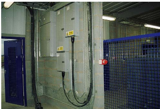
FIGURE 12.5 A neat installation of cable tray in a sub-station carrying feeds to individual distribution boards (W.T. Parker Ltd).
