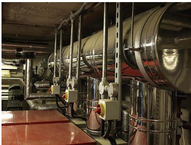
FIGURE 8.5 Wiring systems in use in a boiler house. The main wiring is in steel conduit and short lengths of heat-resisting cable in flexible conduit are used for the connections in the vicinity of the boiler where the temperatures are high (M.W. Cripwell Ltd).
