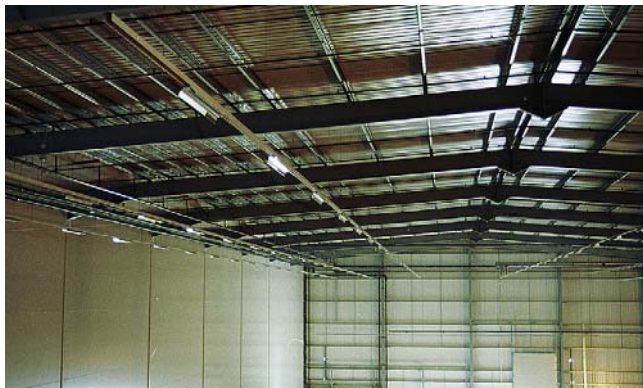
FIGURE 11.2 The busbar lighting units installed in a high-bay storage building. The lighting units have been installed and the installation is ready for the lids to be clipped on (W.T. Parker Ltd).
