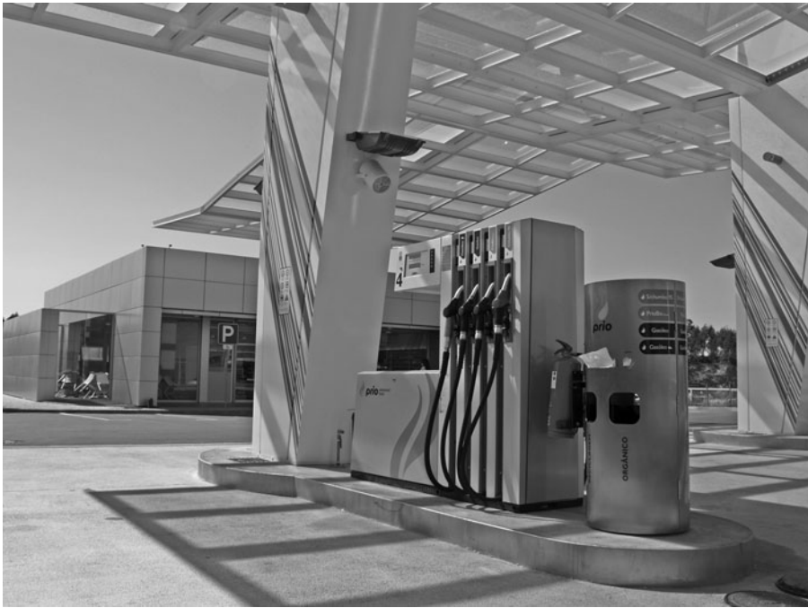
Figure 12.14 Biofuel filling station. Courtesy of MARTIFER.
