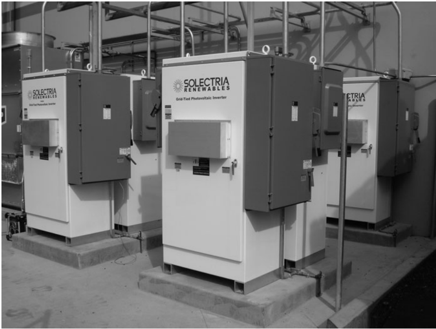
Figure 3.14 External view of inverter electronics. Photo courtesy of Solectria Renewables.
