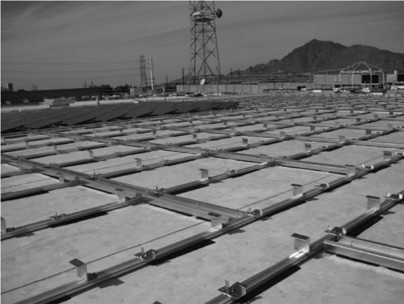
Figure B.16 Nonpenetrating-type roof-mount solar power support railing. Photo courtesy of DWP Solar.
