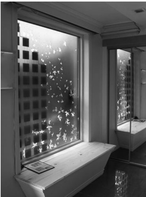
Figure 3.27 BIPV modules in a window glazing. Photo courtesy of Atlantis Energy Systems.
