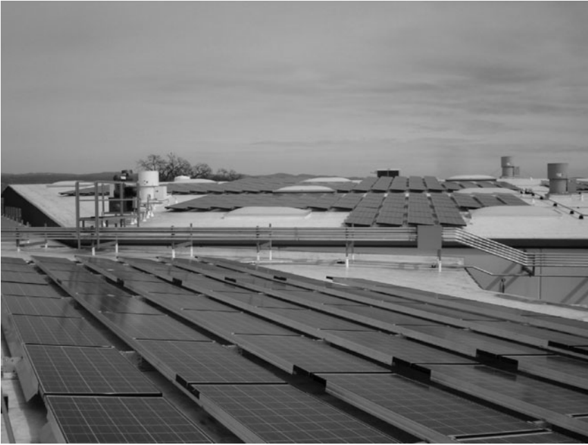
Figure B.6 Roof-mount adjustable solar power racking. Photo courtesy of DWP Solar.
