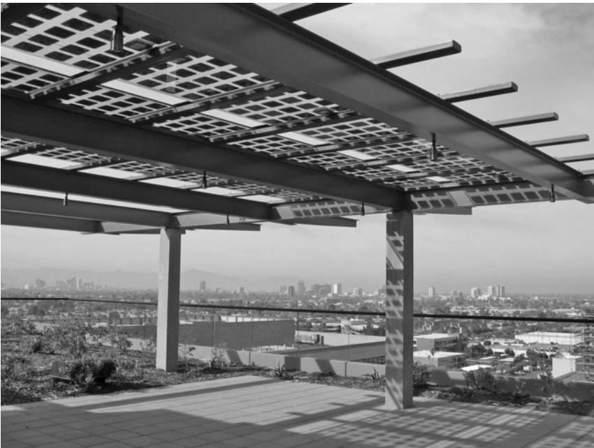
Figure B.7 Building-integrated solar power canopy. Photo courtesy of Atlantis Energy.
