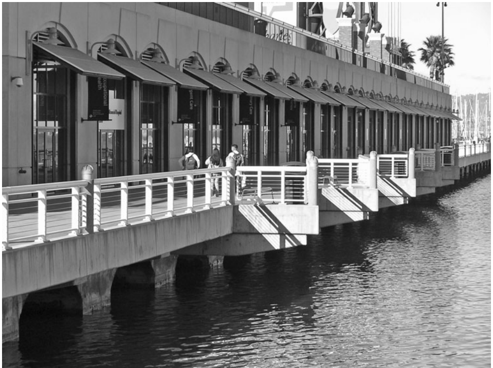
Figure 3.32 Application of a solar PV system in window shading. Photo courtesy of AT&T Ballpark.
