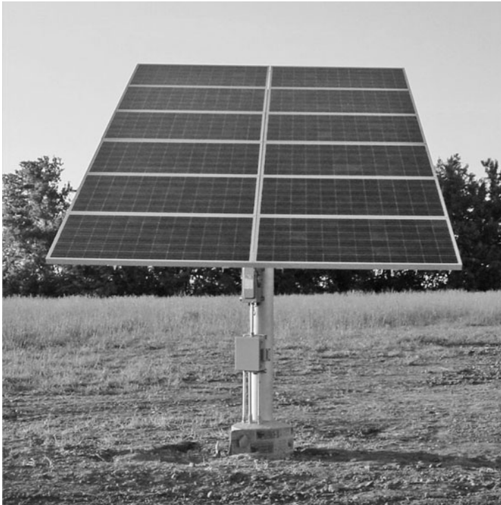
Figure 3.46 Typical ground-mounted solar power system installation. Photo courtesy of DPW Solar.
