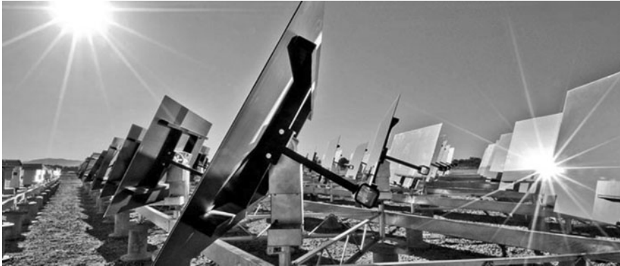
Figure 6.14 Heliostat reflecting mirrors of an eSolar power plant. Courtesy of IdeaLab.
