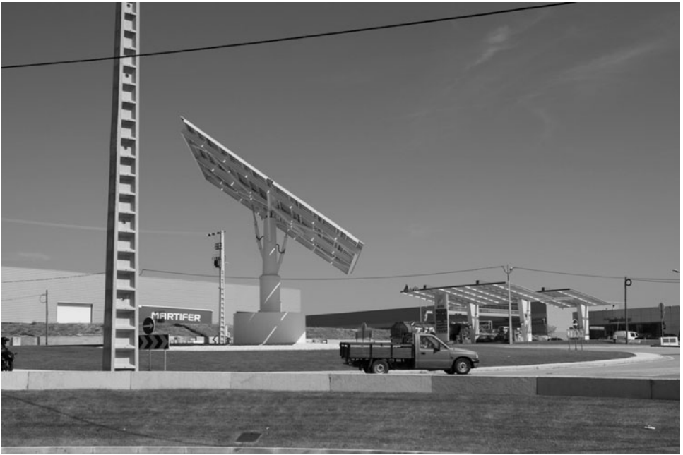
Figure 3.23 A MARTIFER two-axis sun tracker. Photo courtesy of MARTIFER.
