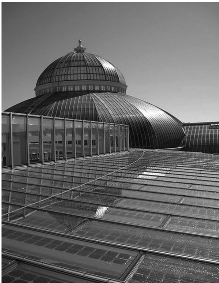
Figure 3.29 An Atlantis Energy Systems custom-designed BIPV. Photo courtesy of Atlantis Energy Systems.
