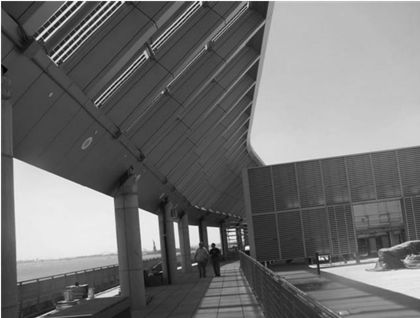
Figure B.1 Building-integrated solar power (BIPV) structure, New York. Photo courtesy of Atlantis Energy.
