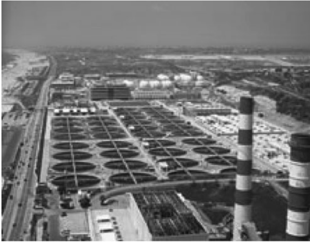
Figure 14.2 View of sedimentation basins at the Hyperion Sewage Treatment Plant, Los Angeles, California.
