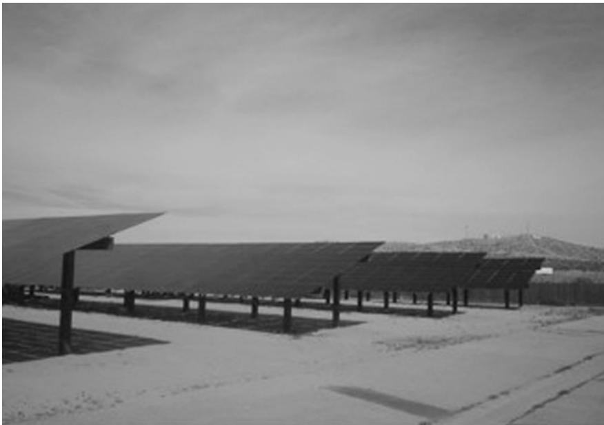
Figure 3.66 Boron solar PV farm. Photo courtesy of Grant Electric.
