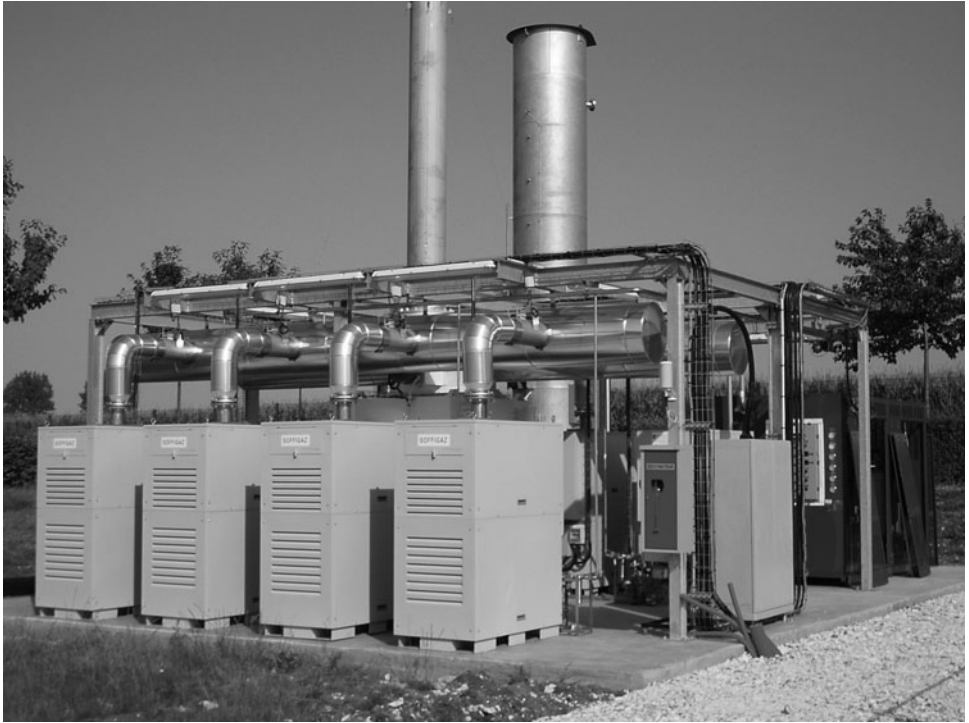
Figure 12.8 Microturbine in a landfill installation. Courtesy of Capstone Microturbine.
