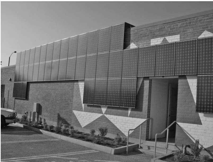
Figure B.15 Wall-mount solar power. Photo courtesy of DWP Solar.
