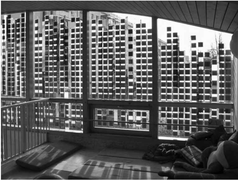
Figure B.10 Building-integrated solar power used as decorative curtain wall. Photo courtesy of Atlantis Energy.
