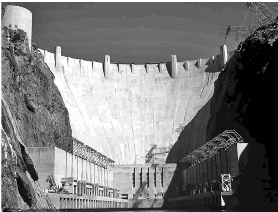
Figure 10.5 Hoover Dam and its hydroelectric power-generating station.
