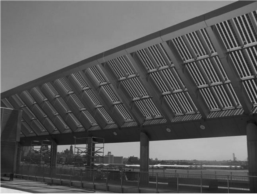
Figure B.2 Building-integrated solar power (BIPV) structure, New York. Photo courtesy of Atlantis Energy. (Continued)
