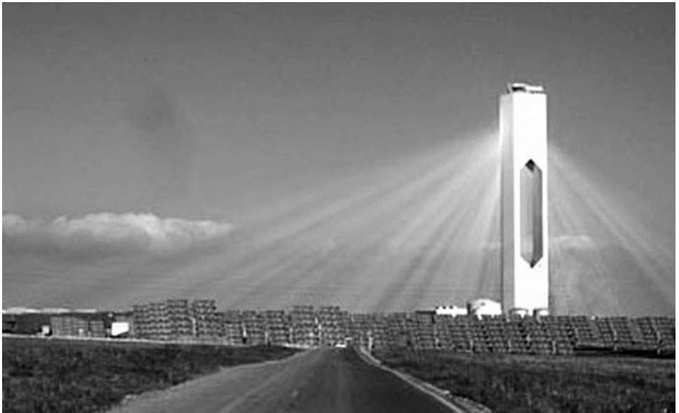
Figure 6.10 A passive solar tower concentrator. Courtesy of Solar Reserve.
