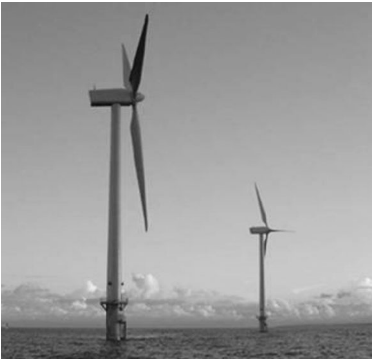
Figure 8.6 Offshore wind turbine installation. Courtesy of AWEMA.
