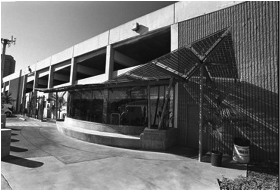
Figure B.9 Building-integrated solar power entrance canopy. Photo courtesy of Atlantis Energy.
