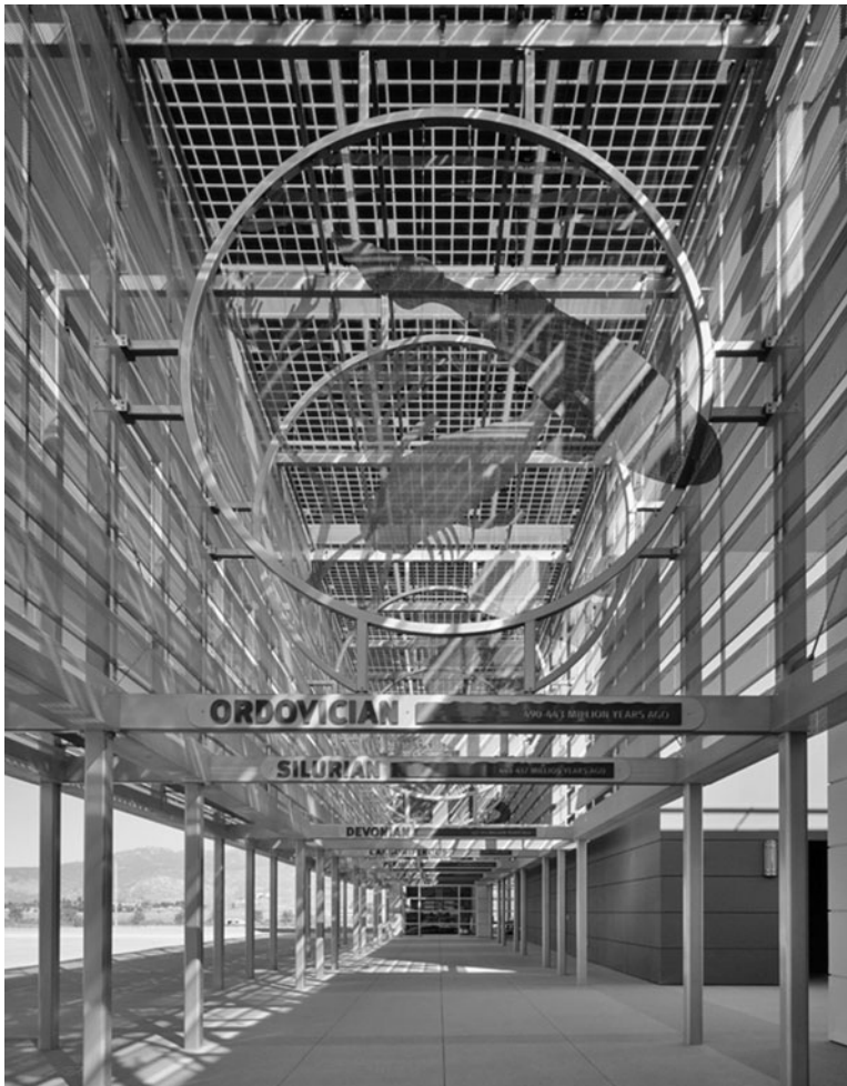
Figure 5.12 Paleontology Museum building integrated photovoltaic (BIPV) solar power system. Photo courtesy of Lehrer+Gangi architects.
