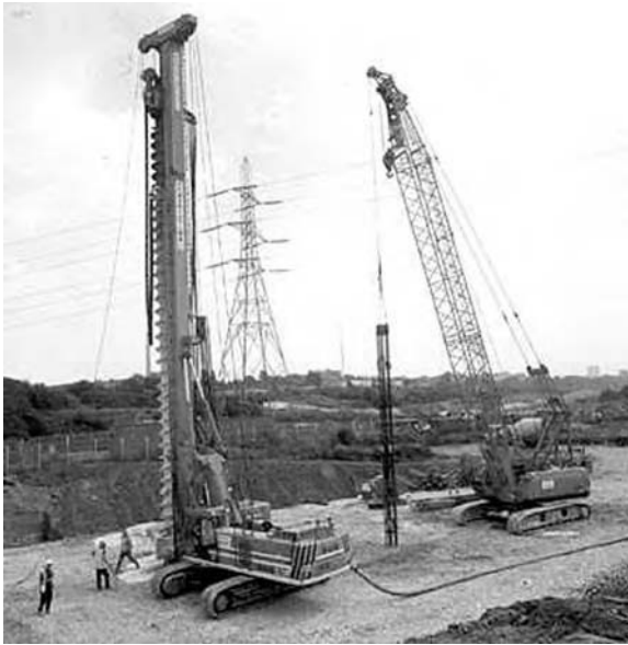
Figure 3.33 Installation of CFA piles in chalk with crane handling reinforcement cage (courtesy Cementation Foundations Skanska).
