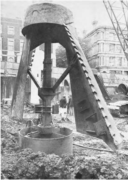
Figure 3.30 Top-hinged under-reaming bucket.
