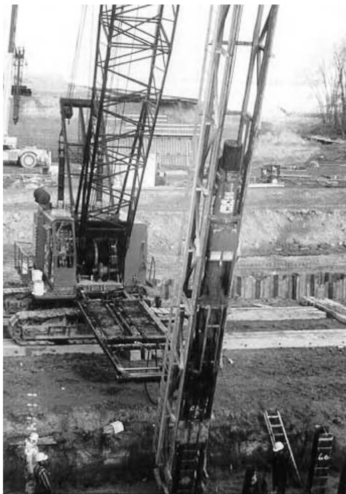
Figure 3.15 Delmag D30–20 diesel hammer on American style leaders with helmet for driving steel H-piles.
