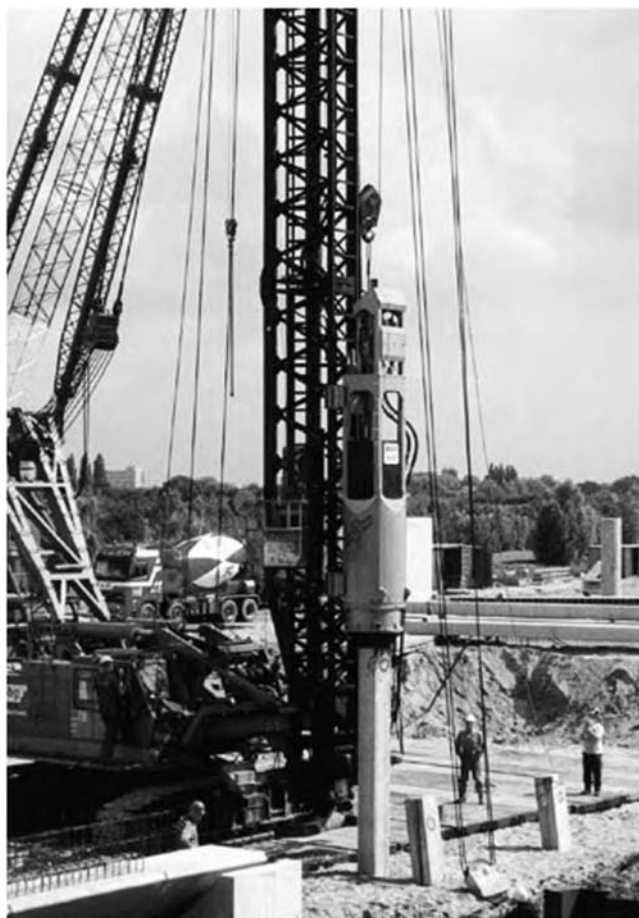
Figure 3.14 BSP CX110 hydraulic piling hammer on Hitachi crane-mounted leader (courtesy BSP International Foundations Ltd).
