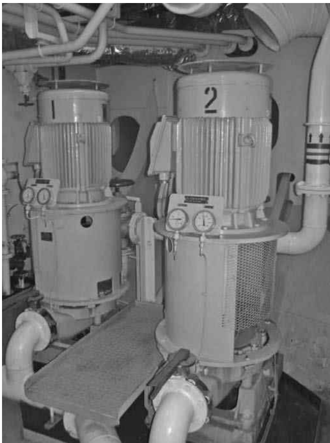
FIGURE 5.2 Vertical shaft motor saves footprints in ships. (From Raul Osigian, U.S. Merchant Marine Academy.)
