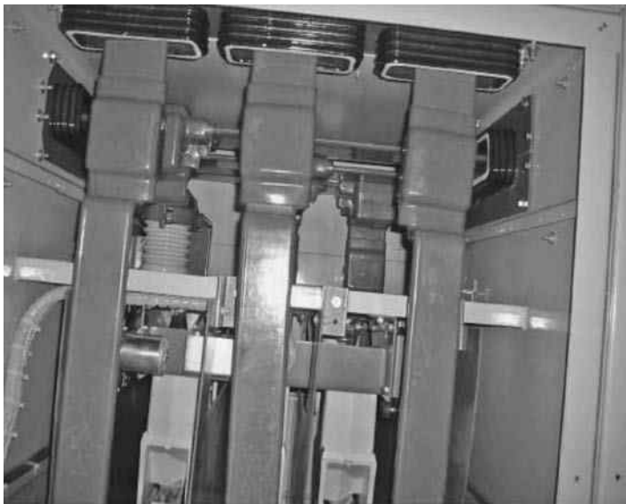
FIGURE 8.9 High voltage bus bars in switchgear through porcelain bus ducts: cast epoxy insulated with joints covered by removable boots (with permission from Myers Power Products, Inc.).
