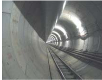
Figure ap.7.11.3 The excavated tunnel.
