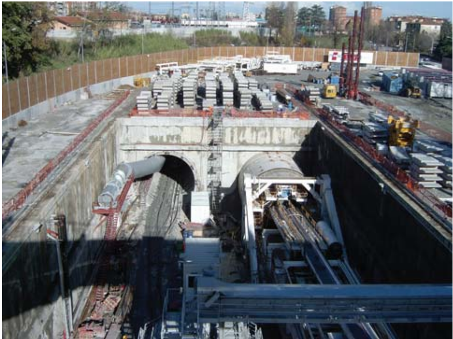
Figure 8.55 The second Lovat TBM ready to start.
