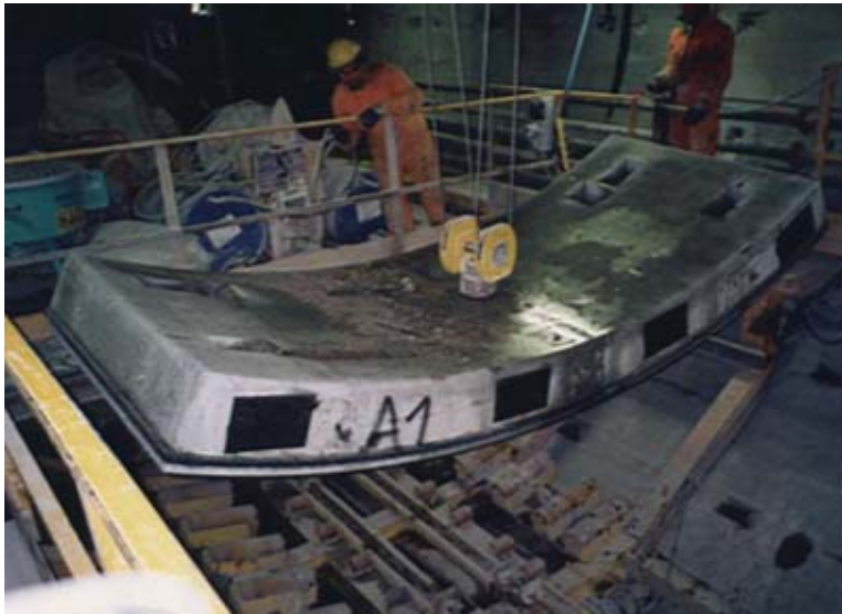
Figure 5.52 A segment with load distributing pads.
