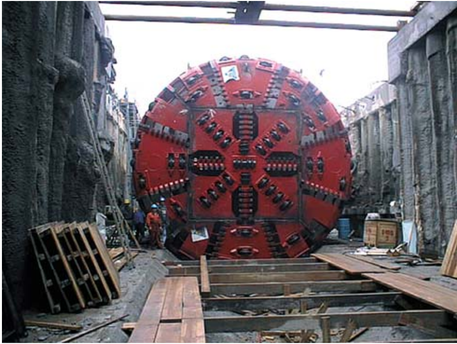
Figure 1.3 One of the Earth Pressure Balance Shields operating in the Porto Metro; the 8.7-m - diameter Herrenknecht TBM.
