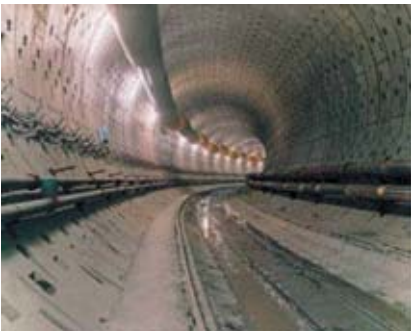
Figure ap.7.7.2 The excavated tunnel.
