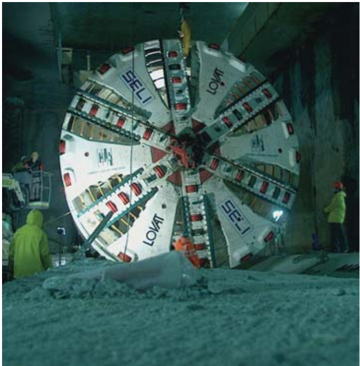
Figure 7.3 Winter assembly of a TBM at the bottom of a shaft.
