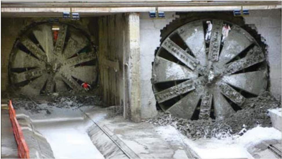
Figure an.3.1 Nodo di Bologna: the final breakthrough of the two TBMs.
