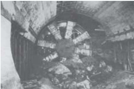
Figure ap.7.1.1 The TBM excavating the Line A tunnel.
