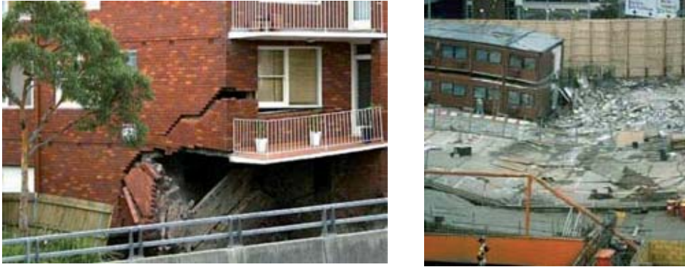
Figure 3.10 Damage to existing structures during tunnel excavation in an urban area (Left: Lane Cove Tunnel, Sydney; Right: Heathrow Express, London).
