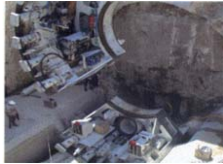
Figure ap.7.10.5 Picture during assembling operation.
