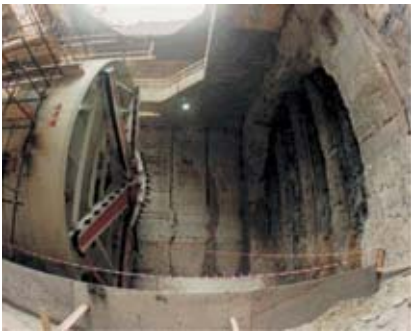
Figure ap.7.7.1 The TBM approaching the tunnel.
