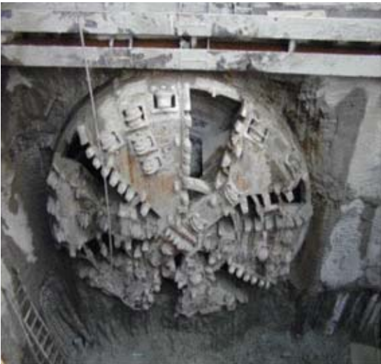
Figure ap.7.8.5 The TBM cutterhead.
