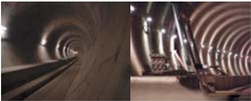
Figure ap.7.12.3 The excavated tunnel.
