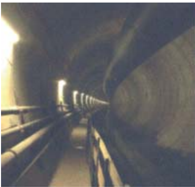
Figure ap.7.10.4 A picture of the tunnel.
