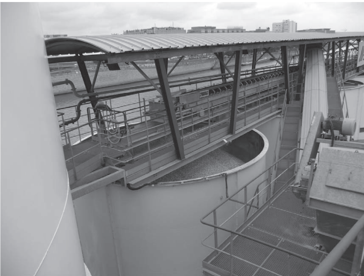
Figure 17.8 Coarse aggregate storage; Cemex plant at Ivry.
