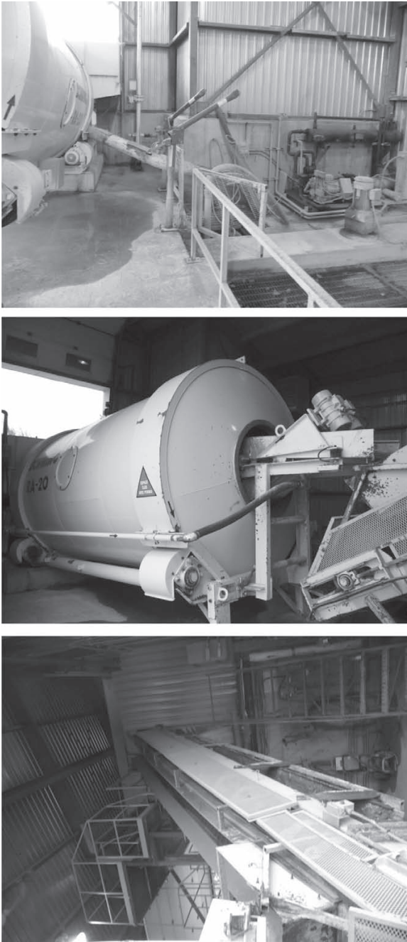
Figure 17.19 Recovery of the aggregates from the unused fresh concrete; Demix Béton plant.
