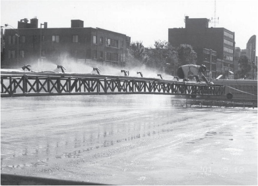
Figure 13.1 Fogging to prevent plastic shrinkage.
