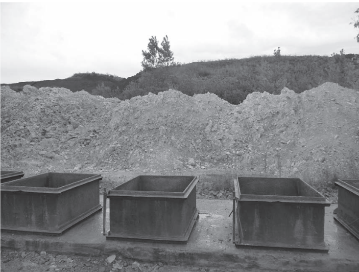
Figure 17.18 Forms for making concrete blocks; Demix Béton plant.
