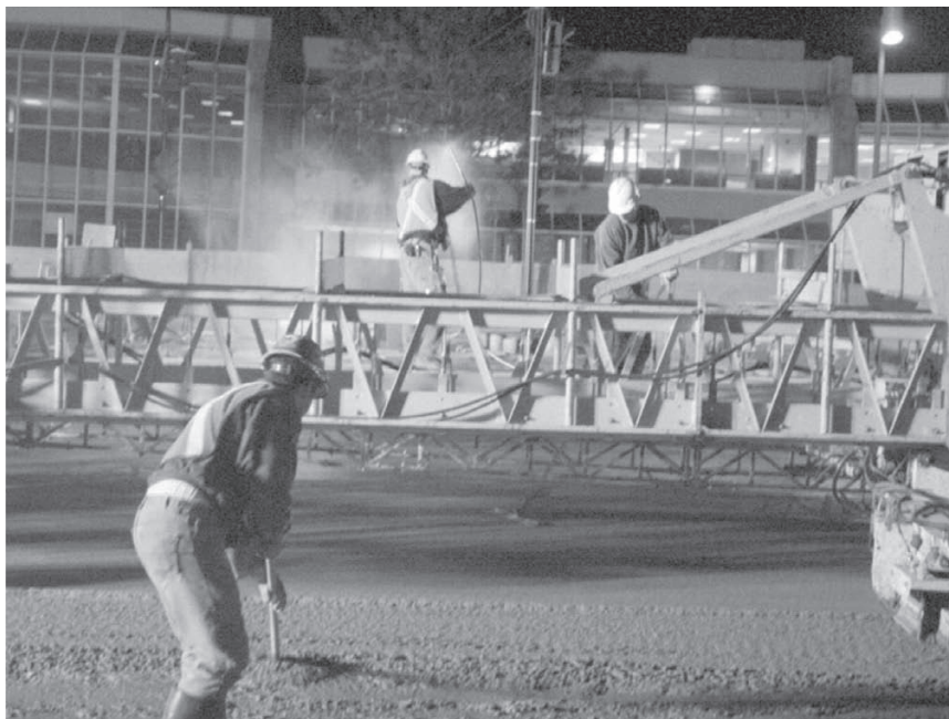
Figure 13.2 Application of a curing membrane just after concrete casting.
