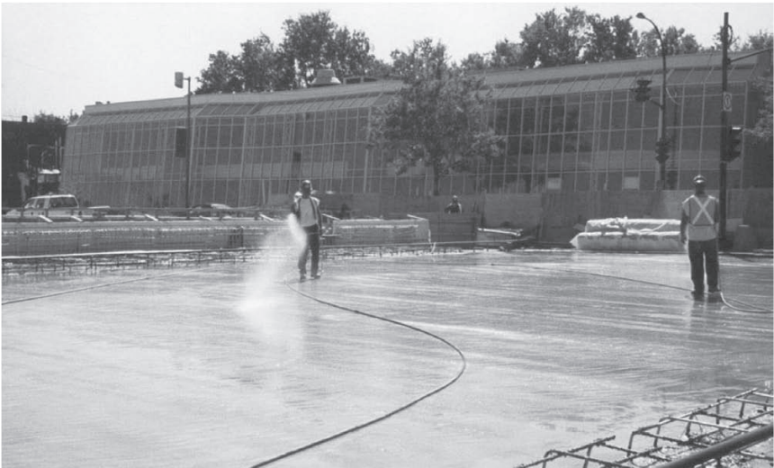
Figure 13.3 Yes, they are paid to water-cure concrete and they do it diligently.
