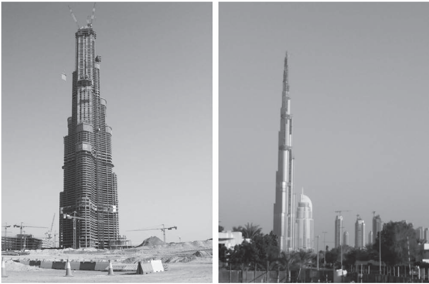
Figure 3.6 The Burj Khalifa Tower in Dubai.
