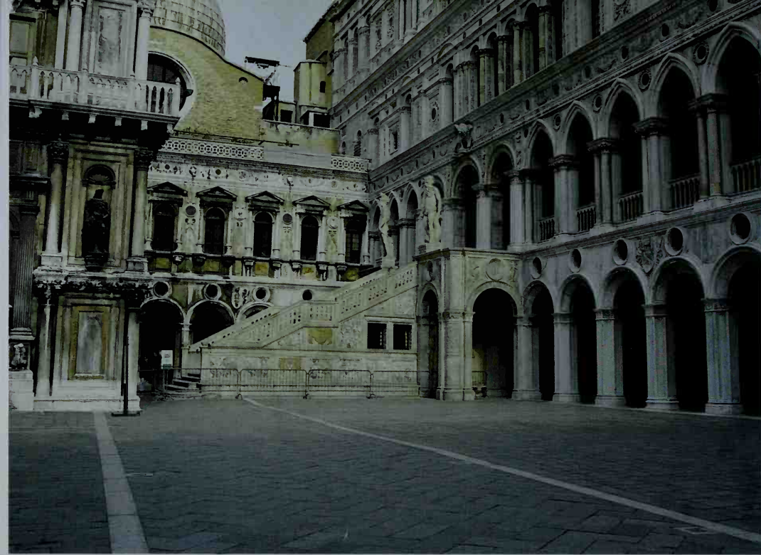
70 Palazzo Ducale, courtyard, towards the Arco Foscari, mid-fifteenth century; east wing (on the right) begun after fire of 1483
