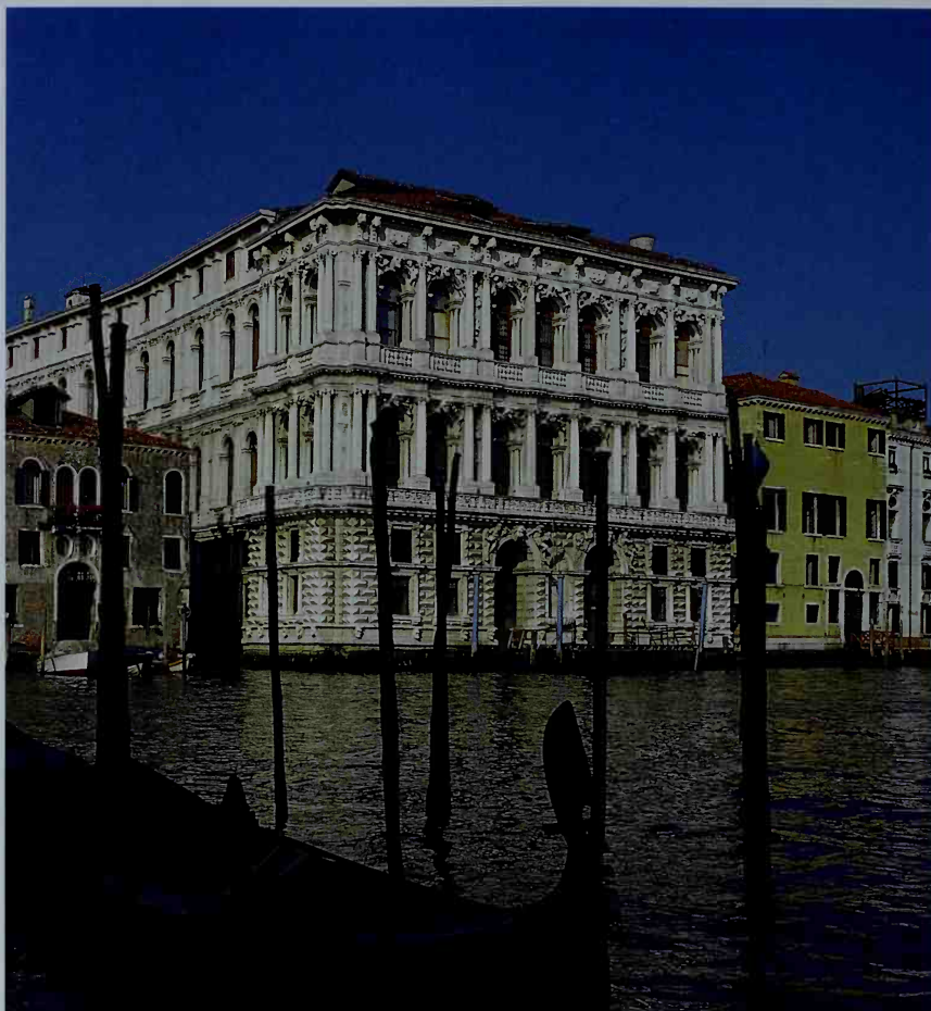
130 Ca' Pesaro, by Longhena, begun c.1652; completed by Antonio Gaspari
