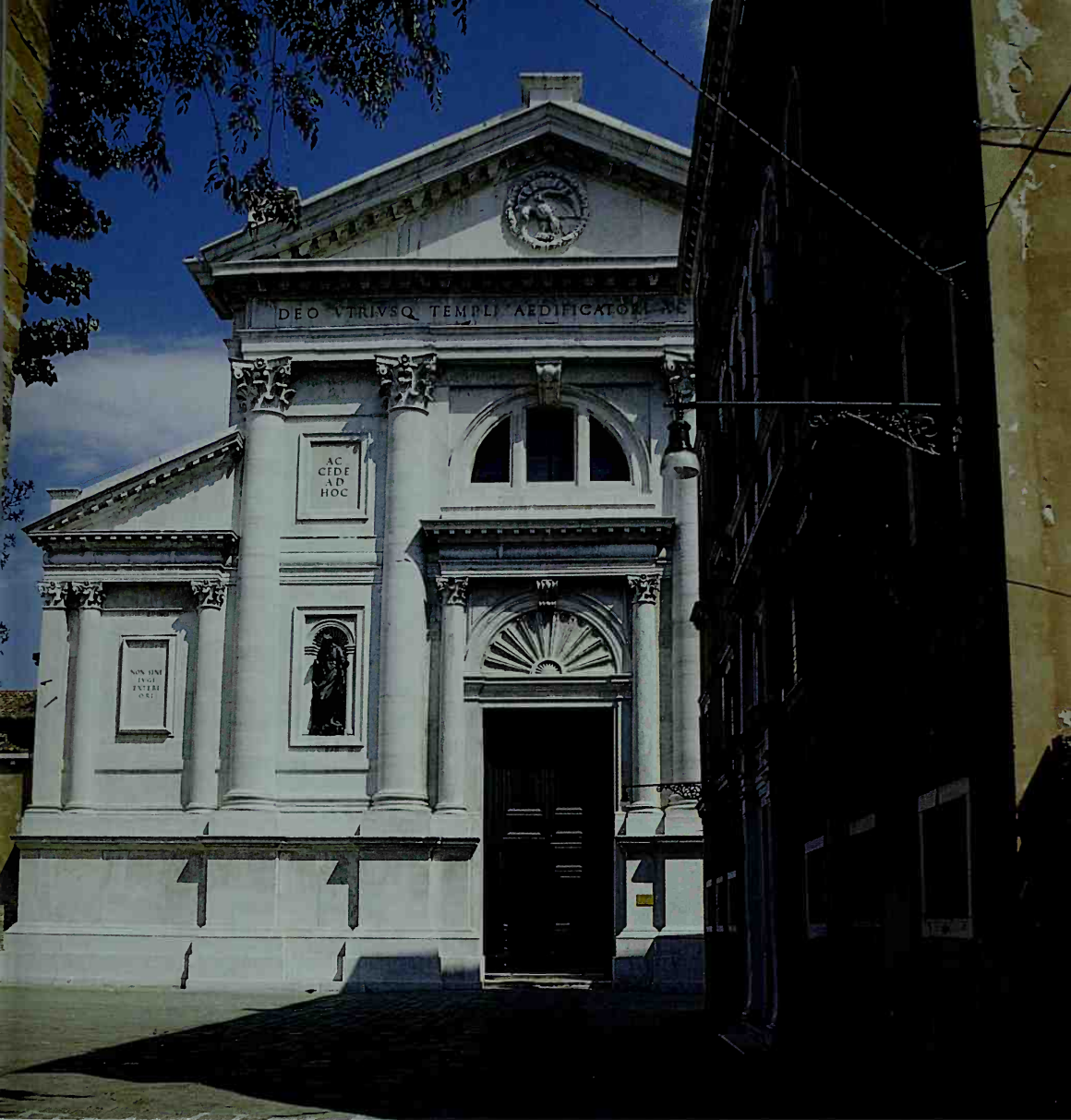
117 San Francesco della Vigna, façade by Palladio, begun c.1562
