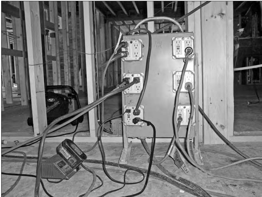
Figure 2-4: A freestanding panel inside the work site gives your crew more flexibility.
