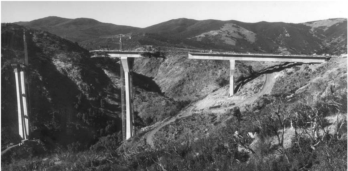
Fig. 17.54 Segmental cast-in-place concrete construction in progress for the Pine Valley Bridge, California. (California Department of Transportation.)
