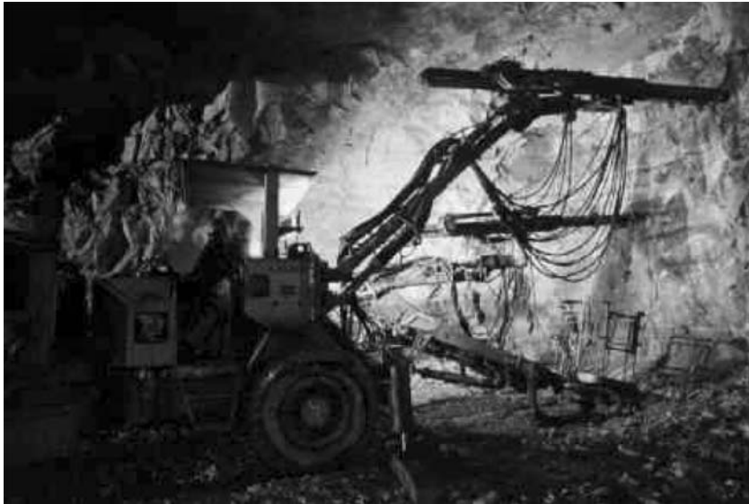
Fig. 20.10 Drill and Blast (TARP).
