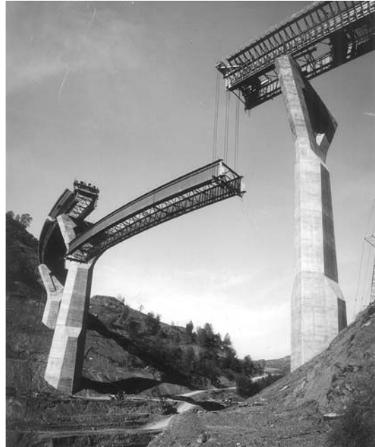
Fig. 17.33 Curved girders of Tuolumne River Bridge, California, were erected in pairs with their cross frames connected between them. (California Department of Transportation.)
