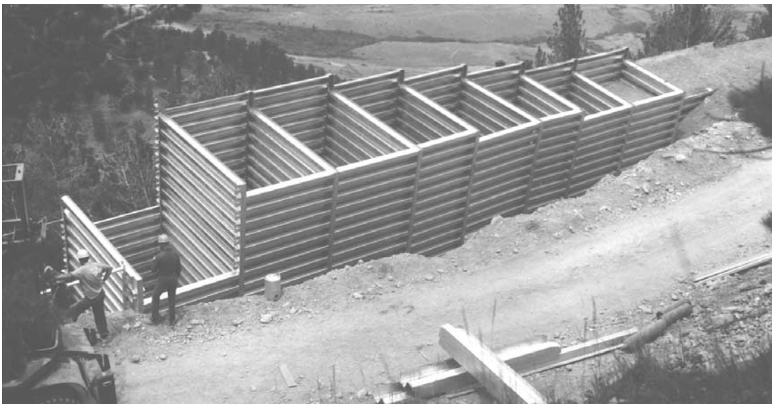
Fig. 10.26 Bin-type retaining wall of cold-formed steel.
