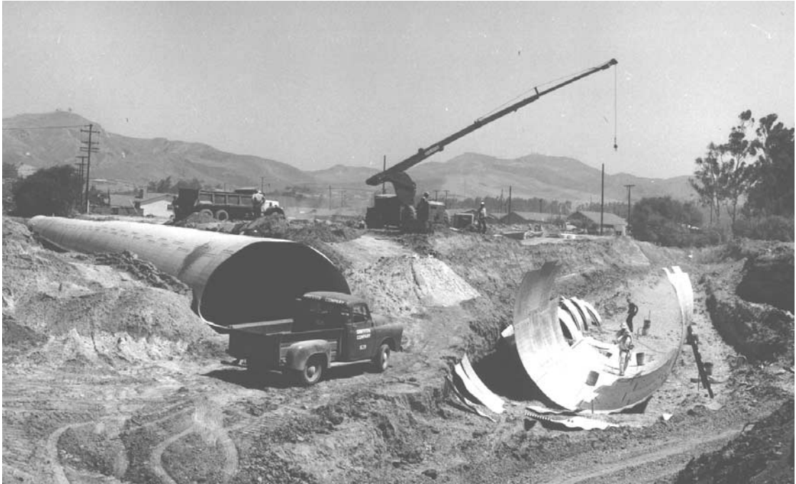
Fig. 10.21 Structural-plate pipe is shown being bolted together at right. Completely assembled structural-plate pipe arch is shown at left.
