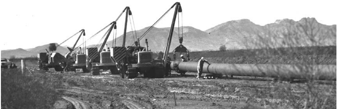
Fig. 13.11 Pipelayers. ( Caterpillar Tractor Co. )
