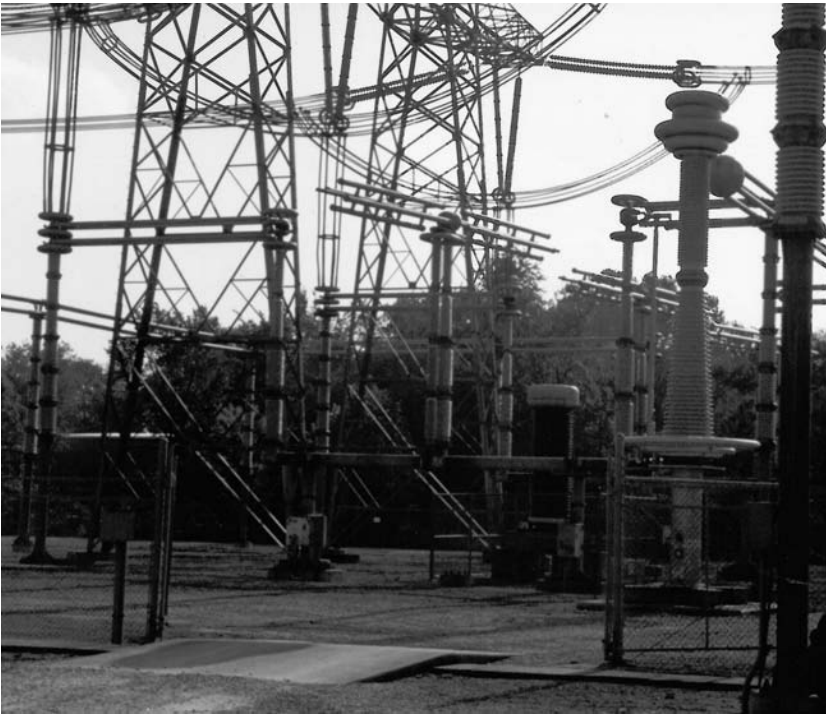
FIGURE 6.11 A 800-kV disconnect switch on the ac side at the same converter station.
