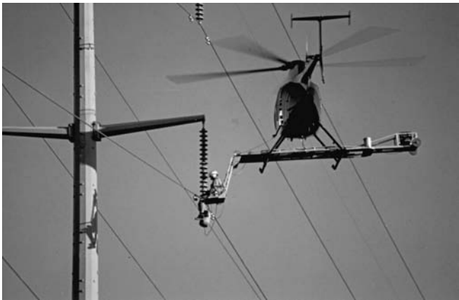
FIGURE 2.15 A lineman working from a helicopter platform.
