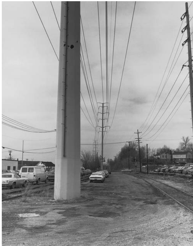
FIGURE 2.6 A double circuit 138-kV line built by using steel poles, having two 138-kV circuits underbuild. (Union Electric Company.)
