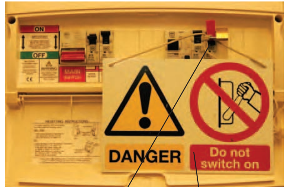
Isolate and lock off
