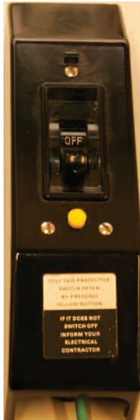
A typical voltage – operated earth leakage current breaker (ELCB) – now obsolete
