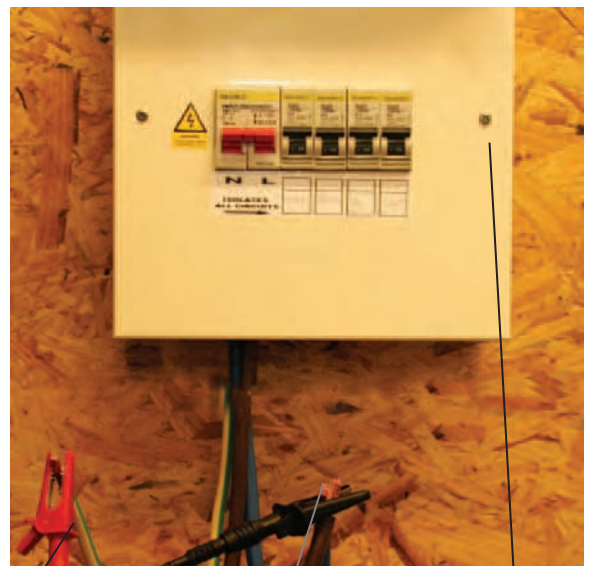
Earthing conductor
