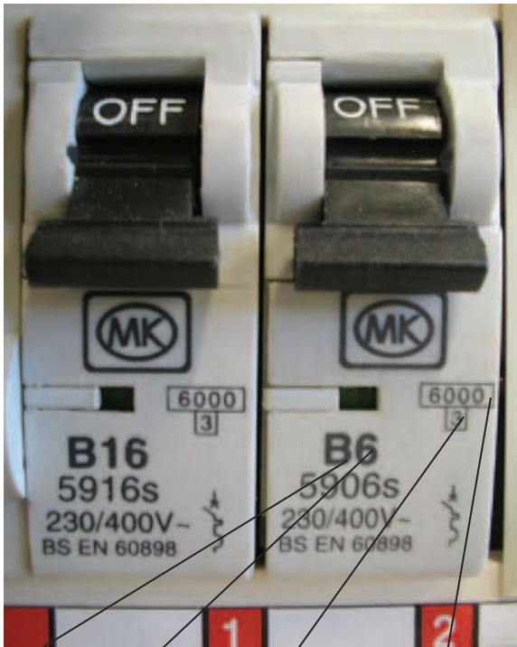
Type In rating Ics rating Icn rating
