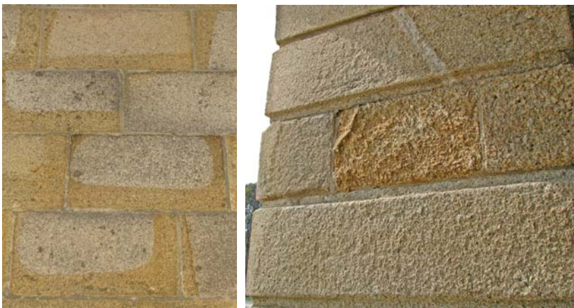
Figure 9. Different tonalities (discolouration) in applied granite stones related to previous weathering of rock masses (a, b). It is frequently observed that granite stones with different discolouration tonalities (representing different previous weathering intensity) present different decay intensity (b).
