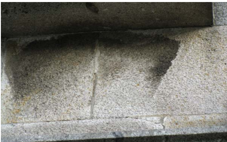
Figure 7. Decay patterns apparently related to bedding.
