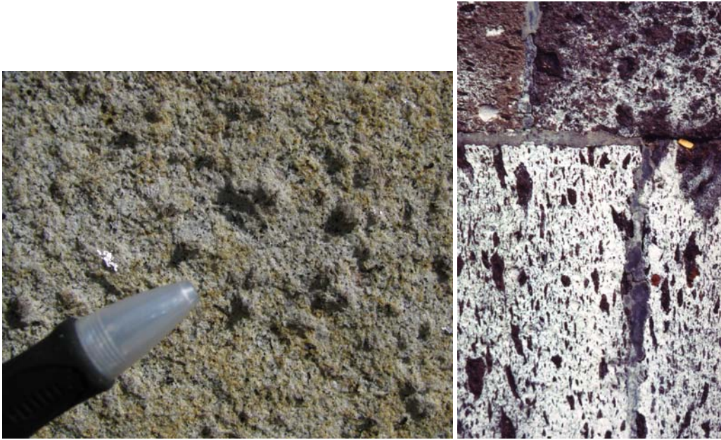
Figure 5. Differential relief in granite stones (a) and differences in patterns of efflorescences in volcanic stones (b) related to rock heterogeneity.
