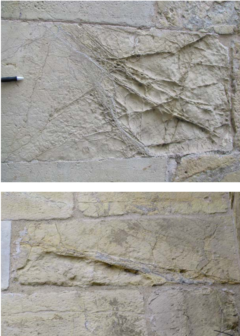
Figure 12. Differential erosion features in limestones related to heterogeneity (a, b).
