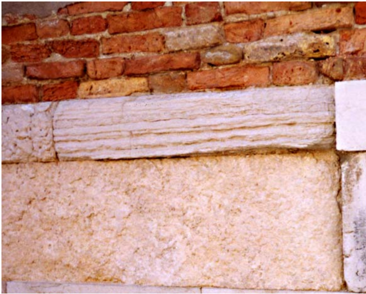
Figure 7. Decay patterns apparently related to bedding.
