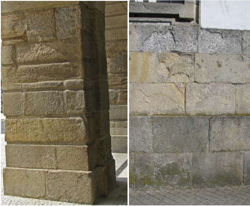
Figure 4. Distribution of decay features suggestion capillary rising of salt solutions on granites (a, b).
