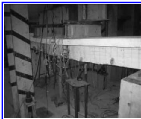
Figure 5. Overall deformation of SCB-1.
