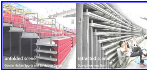
Figure 9. Retractable seating in the site.
