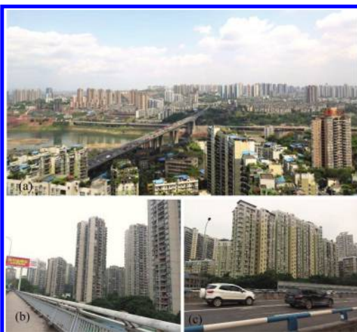
Figure 1. Photographs of case study areas; (a) panoramic view, (b) road-side buildings of Housing estate A, (c) road-side buildings of Housing estate B.
