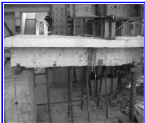
Figure 6. Crack distribution of SCB-1.
