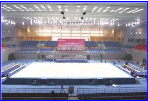
Figure 3. Interior scene in Beijing Forestry University gymnasium with roof optical pipes.
