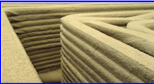
Figure 1. 3D printed concrete by Chinese company WinSun.
