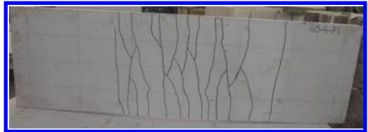
Figure 4. Flexural cracks in specimen 40-4-F1.
