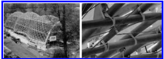
Figure 9. Construction process and node of Japan pavilion of Hanover expo (Tong 2013).
