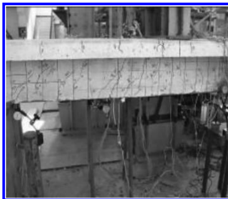
Figure 8. Crack distribution of SCB-2.
