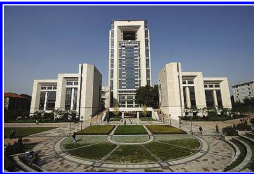
Figure 1. Main administrative and teaching building external view (Source: self-take).
