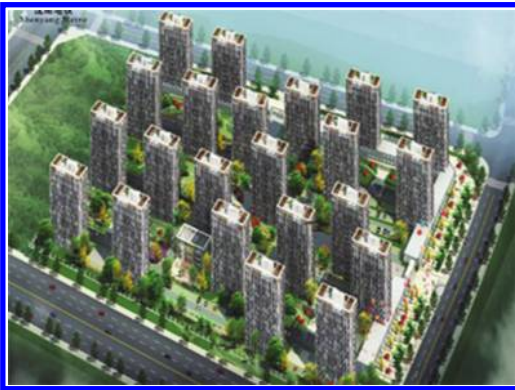
Figure 4. The aerial view of Shenyang Metro Huimin Town projects.
