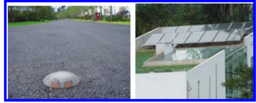
Figure 5. Solar energy ground lights and solar heat-collecting panel on the roof (Jiang 2007).
