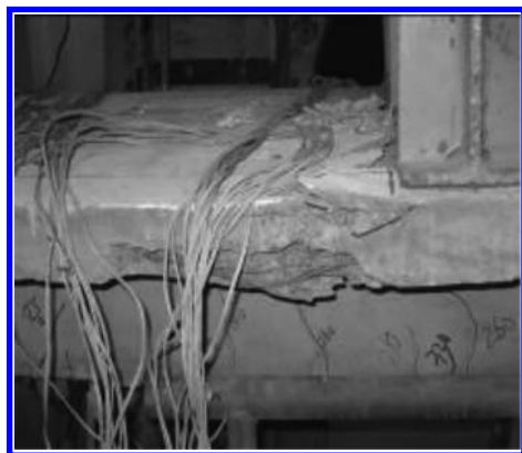
Figure 4. Crushing of the concrete flange.
