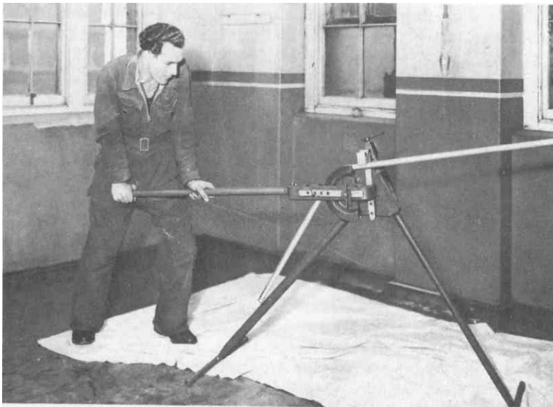
Fig. 8.16. Bending machine for medium sized conduit
