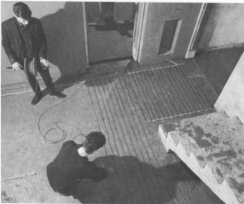
Fig. 6.14. Installing a floor warming cable. The cable is laid onto concrete and plastic spacer bars (above) are used to make the turns at the end of each run (BICC)
