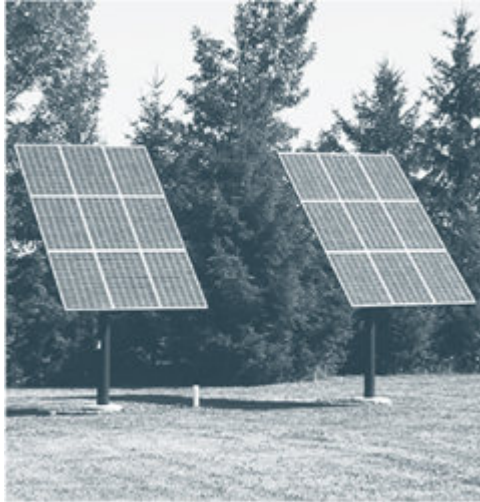
Figure 8.7. Pole-Mounted Array. Each array is mounted on a pole anchored to the ground and is installed at the optimum angle for its location. Pole-mounted arrays provide some flexibility in placing an array on a lot. Credit: Anthony Powell.
