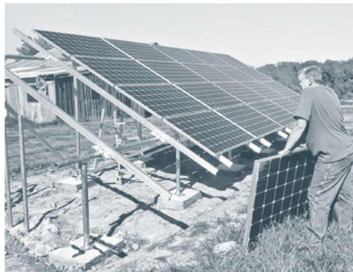
Figure 3.5. Monocrystalline Module. Even from a distance you can tell that these solar modules are made from monocrystalline solar cells. Credit: Dan Chiras.
