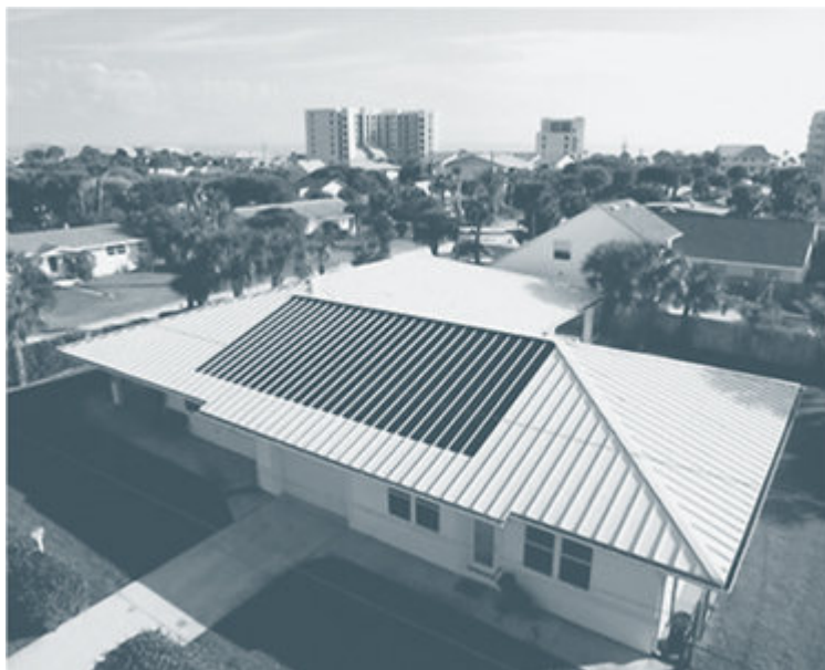
Figure 8.27. PV Laminate from Uni-Solar. PV laminate is applied directly to standing seam metal roof as shown here. Credit: National Renewable Energy Laboratory.
