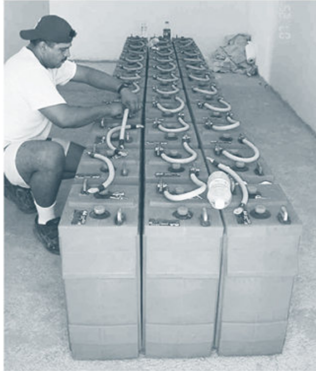
Figure 7.3. Lead-Acid Batteries for RE System. Lead-acid batteries are commonly used in renewable energy systems. Be sure to purchase deep-cycle batteries; keep them in a warm, safe place; recharge quickly after deep discharges; and equalize them periodically. Credit: Surrette Battery Company LTD.
