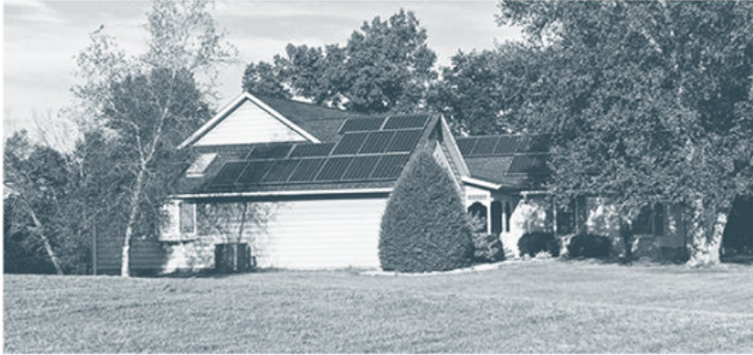
Figure 8.1. East-facing Array. Irresponsible and uninformed solar installers sometimes install PV arrays on east- and west-facing roofs (like the one shown here) under the misguided notion that this orientation will only reduce PV output by 15%. That's not true for steep roofs like this one. This array, which faces due east, is in the shade shortly after solar noon each day. There are also several large shade trees east of the array that block sun part of the year. And, making matters worse, the east-west oriented roof of this house shades the lower part of the array on winter days when the Sun is low in the sky. Don't make this egregious mistake. Credit: Dan Chiras.
