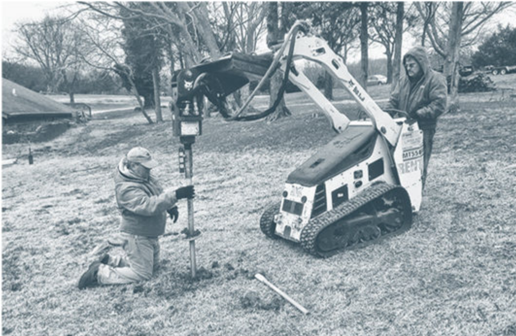
Figure 8.5. Steel Augers Being Installed. We use this machine or a skid steer equipped with an auger attachment to install augers to mount PV systems. One thing I like about this system is that it minimizes ground disturbance and makes for a much neater installation. Credit: Dan Chiras.
