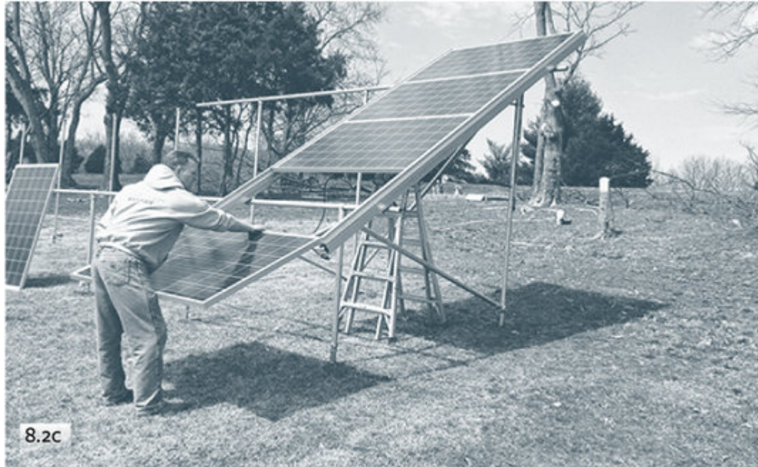
Figure 8.2a, b, and c. Several Types of Rails. Rails for mounting PV modules consist of a series of channels used to attach them to modules and mounting hardware, typically L-feet. (left) Most rails on the market look like this one from Renusol, and most modules are attached by midclamps and endclamps, (not shown). PV Racking makes a rail that I use a lot. As you can see, it has slots into which installers slide the modules. No WEEBs or ground lugs and ground wire are required. (right) A single worker can install the modules by himself. Credit: Dan Chiras.
