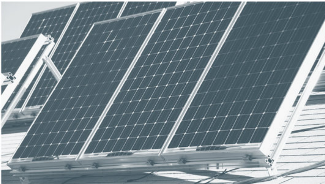
Figure 8.18. PV Array on Standard Rack. In early days of PV industry, modules were mounted on racks like the one shown here. They are designed to allow installers to mount modules at the proper tilt angle to maximize output, though they may not be the most attractive way to install a PV array. Credit: Dan Chiras.
