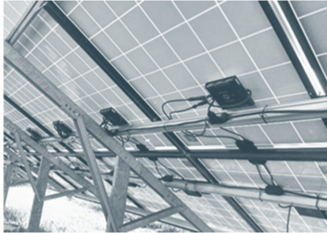
Figure 5.4. Microinverter on an Array. Microinverters like the one shown here are mounted either on the module frames or the rack system in close proximity to PV modules. They convert the DC electricity into 240 V AC electricity. Credit: Dan Chiras.
