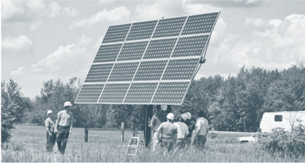
Figure 8.12. Tracking Array. This tracking array was installed by Dan and fellow students at a workshop in Minnesota sponsored by the Midwest Renewable Energy Association located in Custer, Wisconsin. Credit: Dan Chiras.
