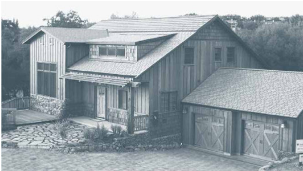
Figure 8.28. Sunslates from Atlantis Energy Systems. Sunslates from Atlantis Energy Systems are solar tiles that replace ordinary roof shingles. The top of this roof is fitted with solar tiles that generate electricity to help meet household demands. Credit: Atlantis Energy Systems.
