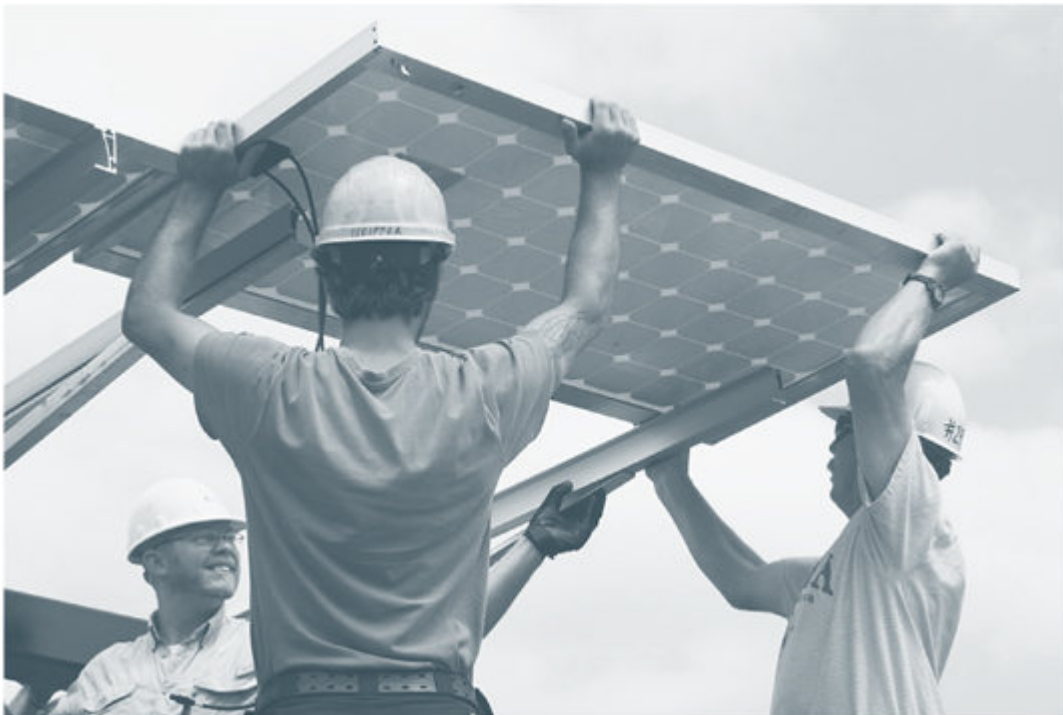
Figure 8.9. Module Being Inserted in Pole-Mount. Workers carefully slide PV modules into place on this dual-axis tracker at a Midwest Renewable Energy Association workshop in Minnesota. Credit: Dan
