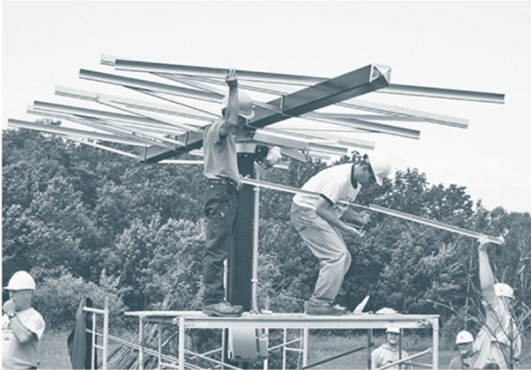
Figure 8.8. Pole-Mount Being Assembled. Students at MREA workshop installing rails on the strong back (center beam) on a pole-mount. Credit: Dan Chiras.
