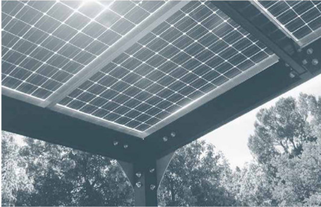
Figure 8.29. Solarscaping. PV modules can be used to create roofs of shade structures, a technique known as solarscaping. This photograph shows a portion of a carport made from PV modules by Lumos Solar. Credit: Lumos Solar.
