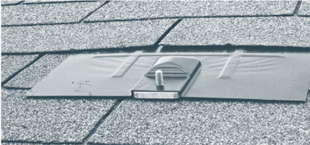
Figure 8.21. Mounting Kit with Flashing. We used this roof mount with flashing on a job on a steel company in Winfield, MO. Flashings such as this help reduce the chances of leakage, giving the homeowner and the installer a little more peace of mind. Credit: Dan Chiras.
