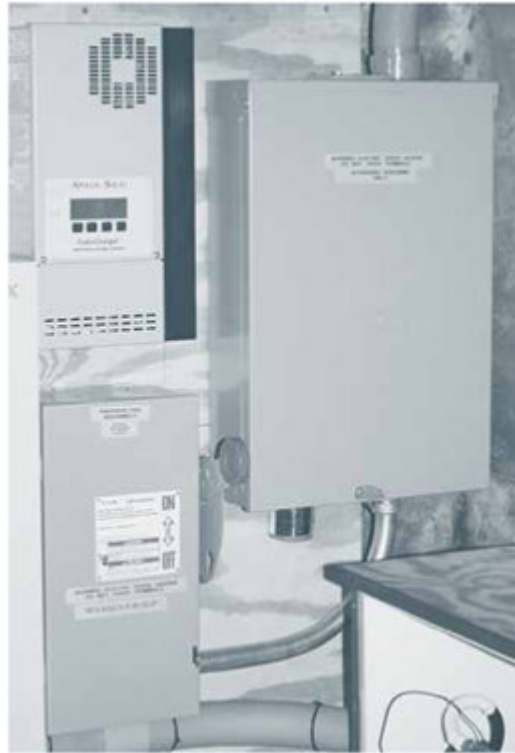
Figure 7.15. Charge Controller. Charge controllers like the one top left from Apollo Solar regulate the flow of electricity to the batteries in off-grid and grid-connected systems with battery backup. Some charge controllers contain maximum power point tracking circuitry to optimize array output and other features as well, like digital meters that display data on volts, amps, and electricity stored in battery banks. Credit: Apollo Solar.
