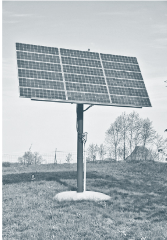
Figure 1.11. Ground-mounted solar arrays like this one accommodate numerous modules and can be oriented and angled to maximize production. Because they allow air to circulate freely around the modules, systems such as these stay cooler than many roof-mounted arrays and thus tend to have a higher output. Credit: Dan Chiras.
