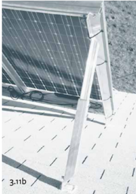
Figure 3.11. (a) Bifacial modules like those installed at the Midwest Renewable Energy Association harvest solar energy off both sides of the modules, although the front side shown here is by far the most productive source of electricity. (b) Sunlight reflecting off the light-colored roofing illuminates the back of the array, boosting its output. Credit: Dan Chiras.
