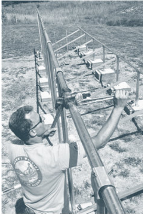
Figure 8.3. Note the cement blocks (ballast) that secure the array on the roof. Credit: Dan Chiras.
