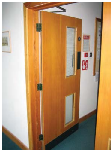
Figure 9.15 A typical fire resisting door
