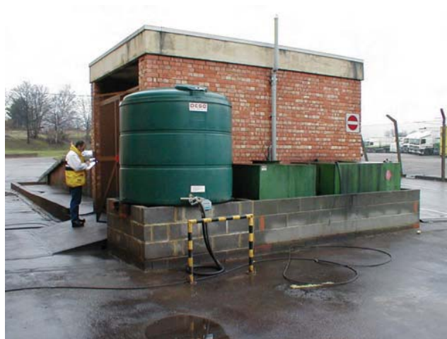
Figure 11.3 Fire safety hazards require active monitoring
