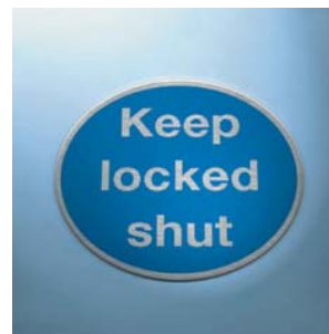
Figure 6.3 Typical fire door keep shut sign
