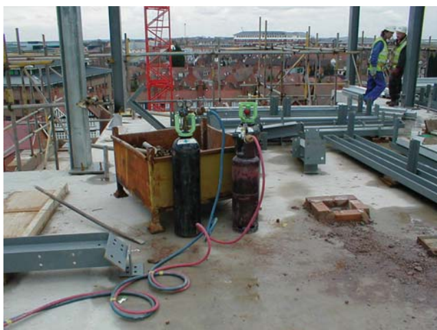
Figure 8.7 Oxy-fuel equipment on a construction site
