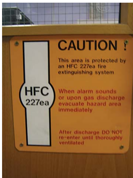
Figure 9.66 Typical warning sign to a computer room fitted with a flood system
