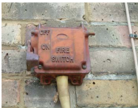
Figure 9.92 Fire fighters switch
