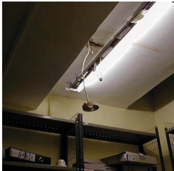
Figure 12.12 The result of contractors working on the fire alarm system – removal of detector head
