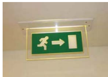
Figure 9.54 Maintained blade emergency light – double sided
