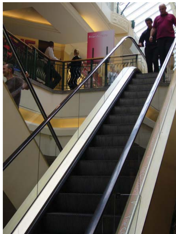
Figure 9.42 Escalators are generally unacceptable as a means of escape
