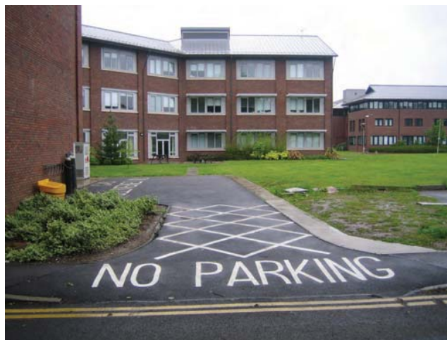
Figure 9.83 Fire service access road
