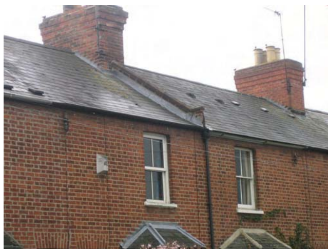
Figure 9.4 Party wall between terraced properties
