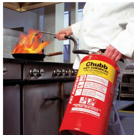
Figure 9.71 Wet chemical fire extinguisher
