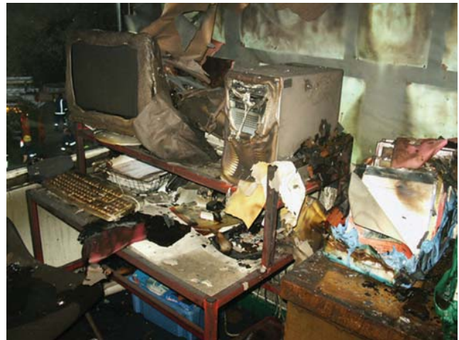
Figure 8.2 Electrical equipment involved in a school fire
