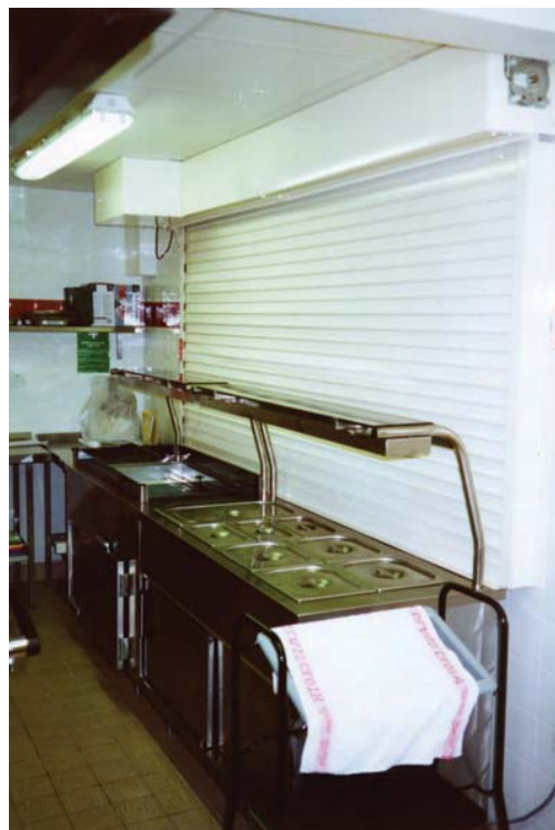
Figure 9.16 Fire shutter
