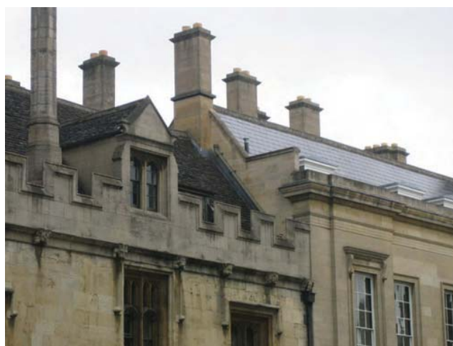
Figure 9.5 Party wall between two adjacent buildings
