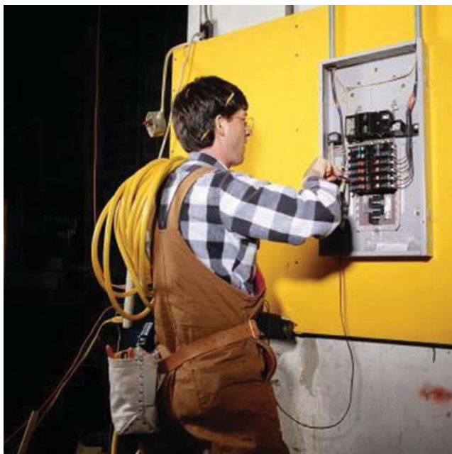
Figure 8.12 Electrical supply testing
