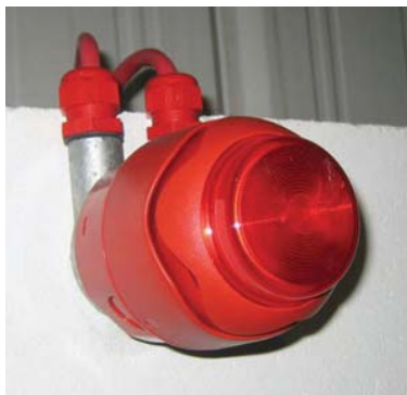
Figure 10.18 Visual alarm combined with an audible sounder
