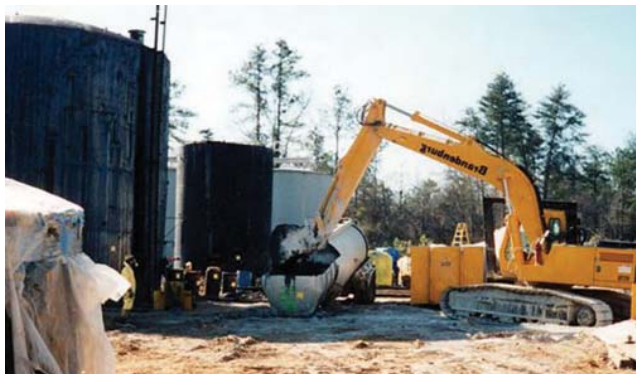
Figure 8.24 Purging tanks during decommissioning
