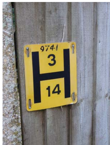
Figure 9.89 Fire hydrant indicator plate
