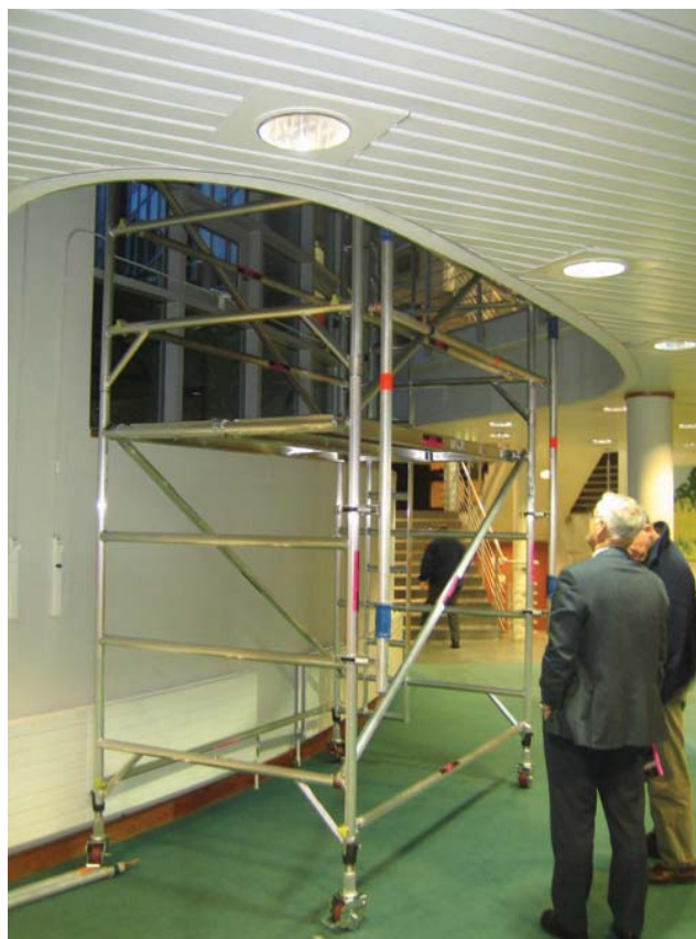
Figure 5.2 Inspecting contractors arrangements for working at height
