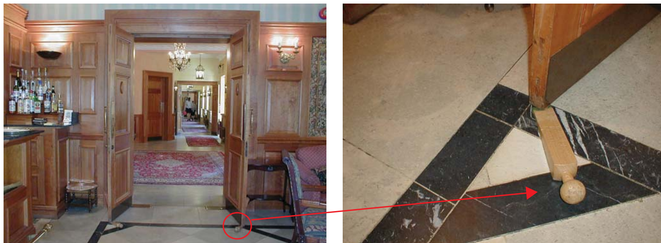
Figure 9.39 Example of abuse of fire compartmentation by the use of door wedges
