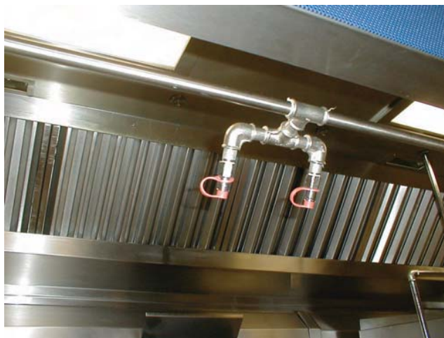
Figure 9.65 Detail of a fixed flooding system fitted to a kitchen range
