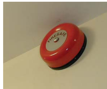
Figure 10.16 Audible warning devices
