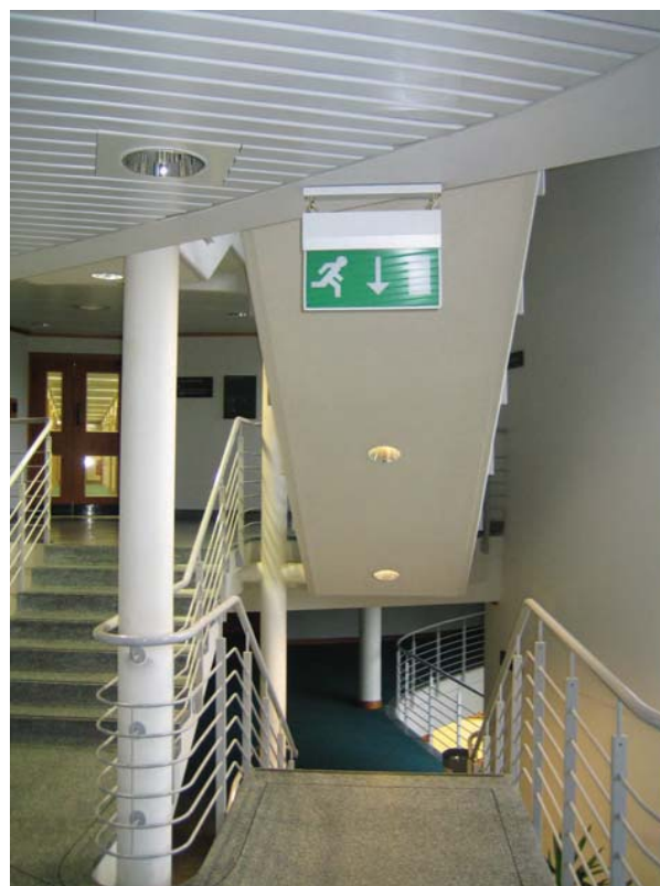
Figure 9.43 Typical modern escape stairway
