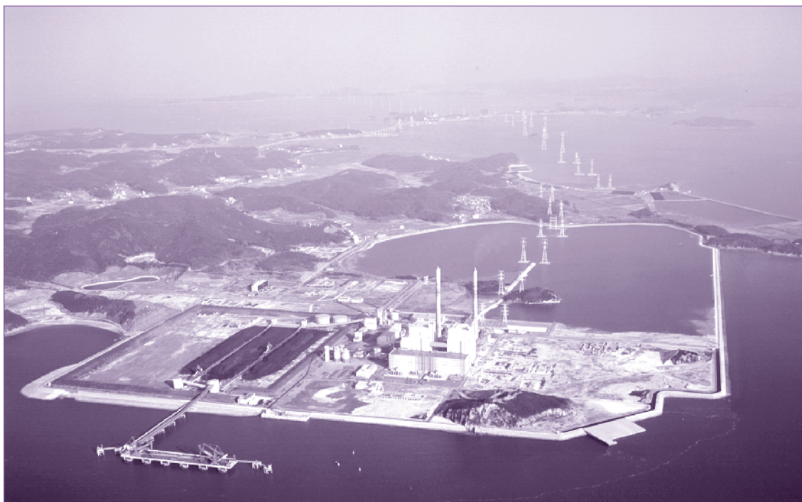
Figure 17 • Younghung Thermal Power Plant general view
