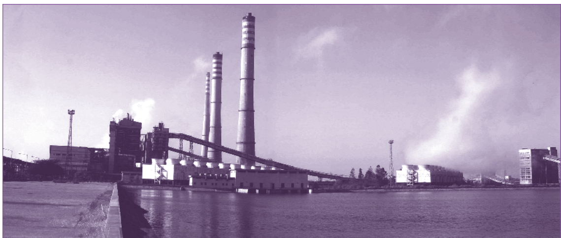
Figure 21 • Suratgarh plant general view
