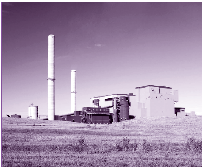
Figure 11 • Genesee 3 general view
