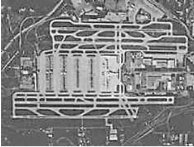
Figure 4-3. Atlanta's Hartsfield International Airport has two sets of parallel runways to accommodate high-volume large-aircraft operations. (Courtesy Hartsfield Atlanta International Airport)
