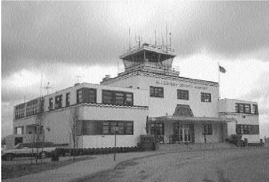
Figure 6-2. Allegheny County, Pennsylvania, historical unit terminal concept. (Photo courtesy Allegheny County Airport)
