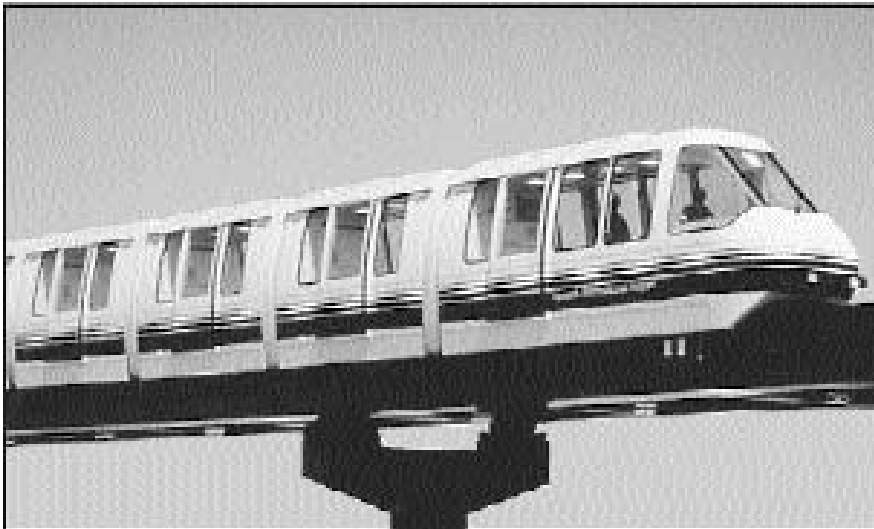
Figure 6-31. The APM system at Newark Liberty International Airport connects the airport terminal with parking and rental car facilities, as well as the regional rail transportation centers. (Picture courtesy Port Authority of New York/New Jersey)
