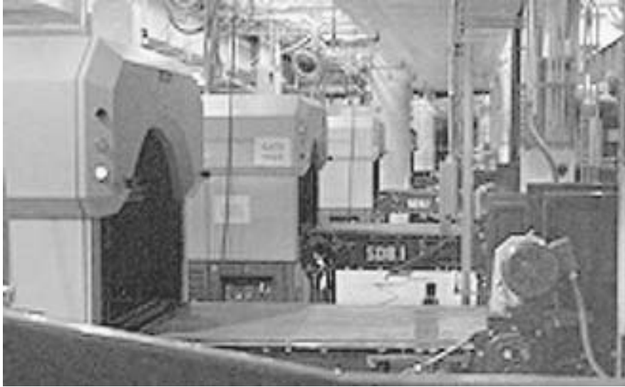
Figure 8-8. EDS machines located “in line” in baggage sorting areas.
