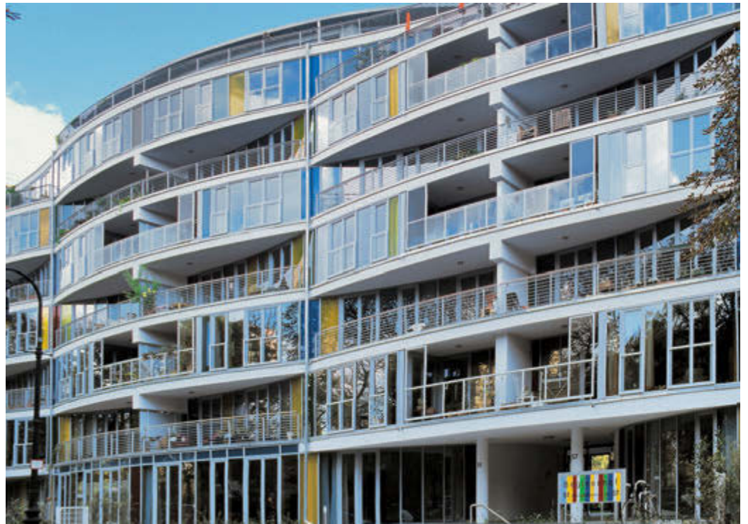
Street façade showing central entrance passageway | Full-height glazing in the interiors | Rooftop maisonette apartment | Gallery walkway facing the courtyard | Greened courtyard as private area for the residents | Plain courtyard elevation
