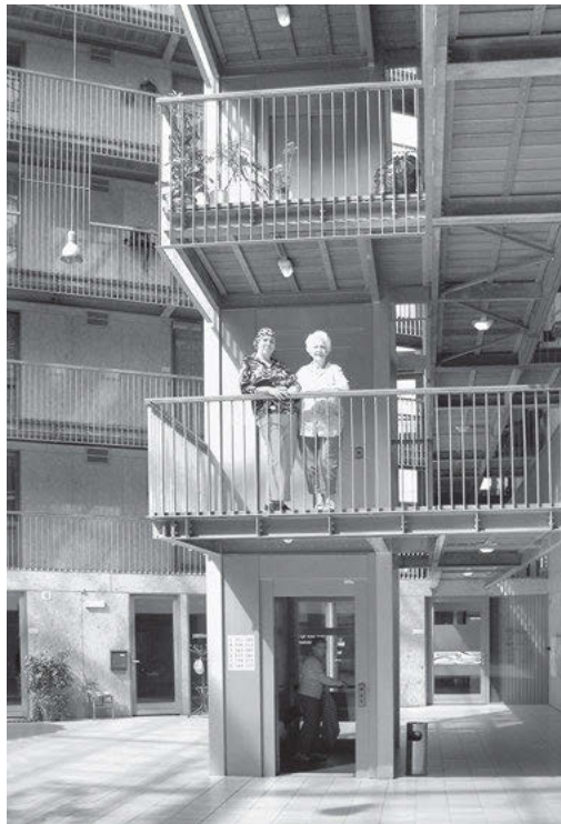
Exterior façade detail | Vertical access | The gallery walkways as semi-private areas | Central atrium covered by a glass roof | Urban context | Interior façades
