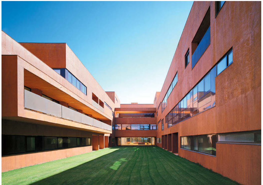
Façade detail | Two slightly-offset parallel buildings from an internal courtyard
