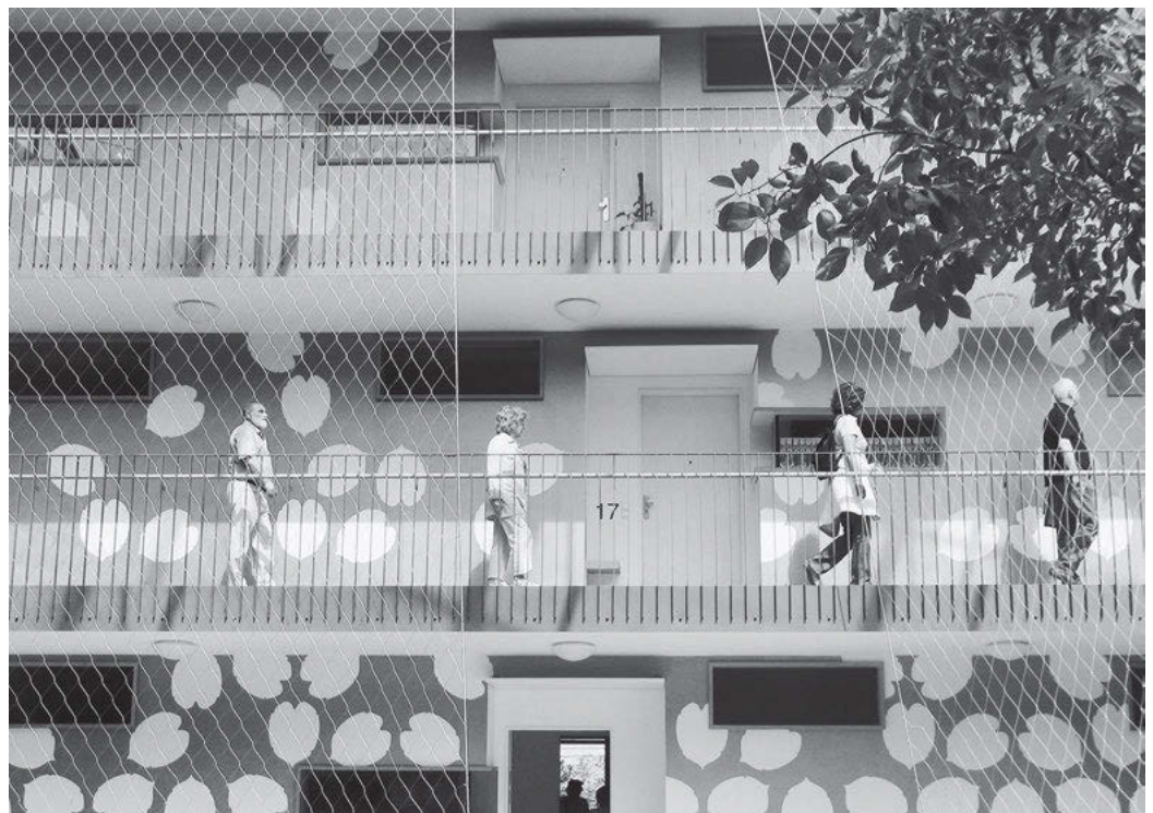
View from a communal terrace of the main landmark in the vicinity | Gallery walkways with personalisable entrances to the apartments
