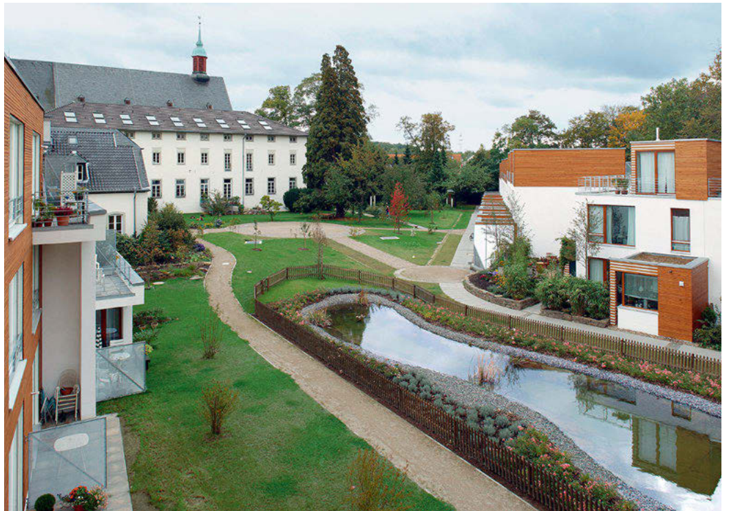
Courtyard in the existing monastery | View of the complex from the north
