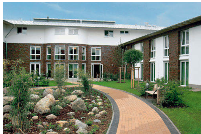
Senior care home in Neu Wulmstorf
