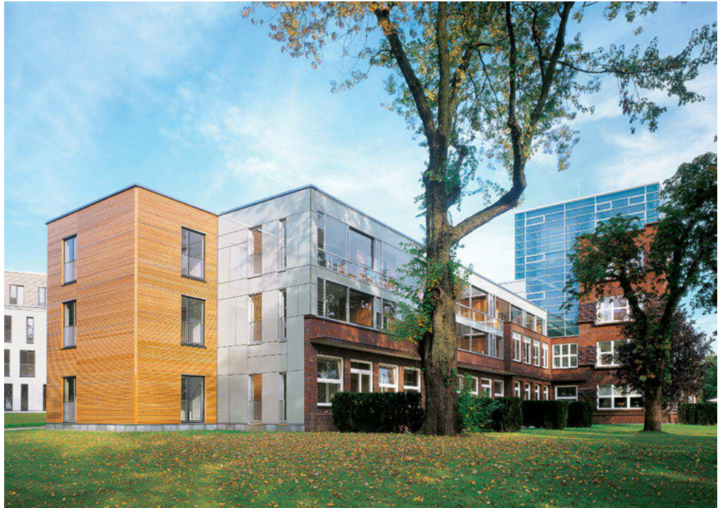
New residential buildings | Integration of the existing brick building in the new building with the landmark glass tower of the brewery in the background | Elevation of the new urban villa
