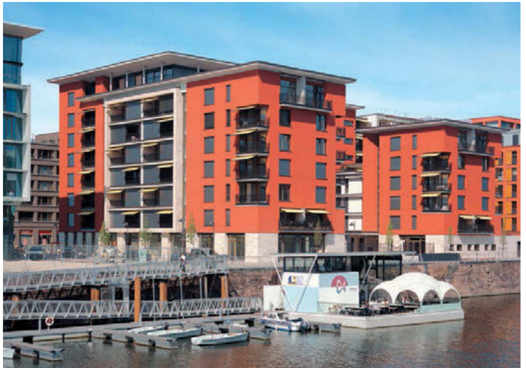
South elevation | East-west orientation of the building between the harbour and Speicherstraße | Central entrance hallway in the ground floor plinth level | Event room on the ground floor
