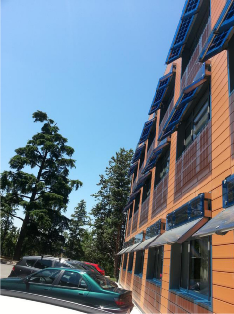
FIGURE 3.15 Low-energy building with overhangs made of PV panels, CIEMAT, Madrid, Spain.
