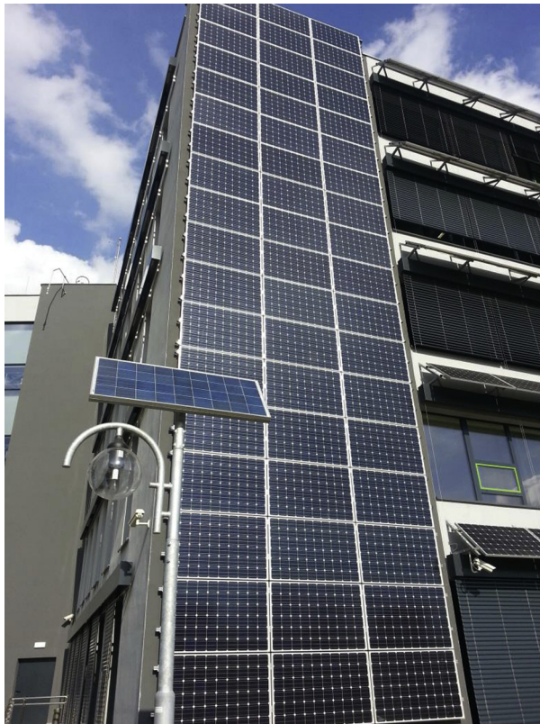
FIGURE 8.1 Passive and active solar building, Euro-Centrum, Katowice, Poland.
