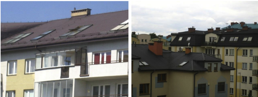
FIGURE 6.72 Examples of multifamily buildings with attics in Warsaw, Poland.
