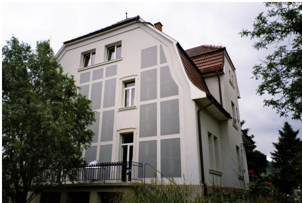
FIGURE 5.17 Villa Tanheim, headquarters of the International Solar Energy Society (ISES), Freiburg, Germany. Transparent insulations on the western façade.
