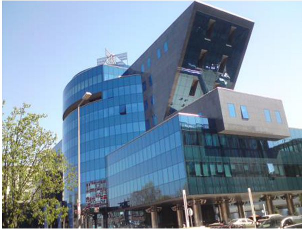
FIGURE 3.13 Example of an office building in Warsaw, with an upper part of “reversed facade.”
