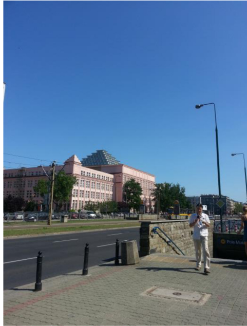
FIGURE 3.17 Glazed pyramid roof of the main building of the Warsaw School of Economics, Warsaw, Poland.
