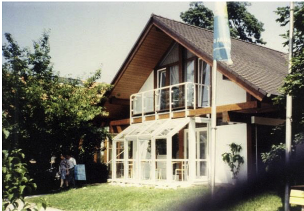
FIGURE 5.5 Typical example of a buffer space attached to a single-family house in form of a winter garden, Ulm, Germany.
