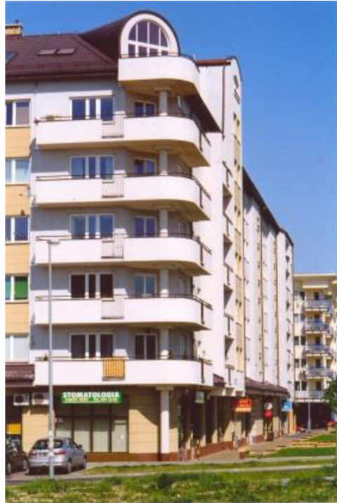
FIGURE 3.14 Window shading by balcony floors in a residential building in Warsaw, Poland.
