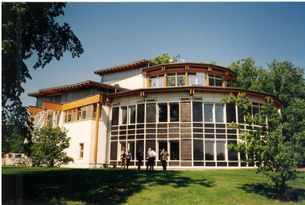
FIGURE 3.2 A low-energy building, Environment Center, Cottbus, Germany.
