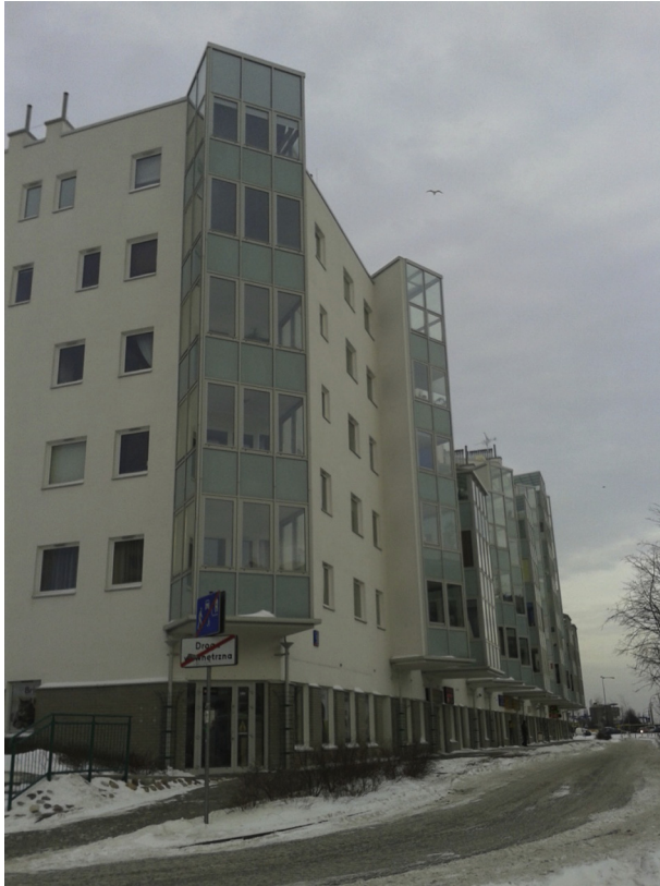
FIGURE 5.8 Example of a buffer space in form of a glazed loggia, Warsaw, Poland.
