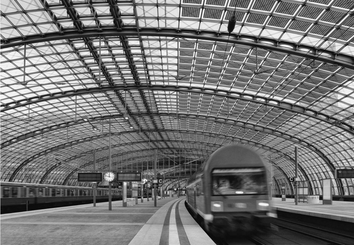
4.11 The platform roof spans up to 66m and the maximum depth of the compression members in the arch is only 13cm. von Gerkan, Marg und Partner and Schlaich Bergermann und Partner, Berlin, Germany, 2006.
