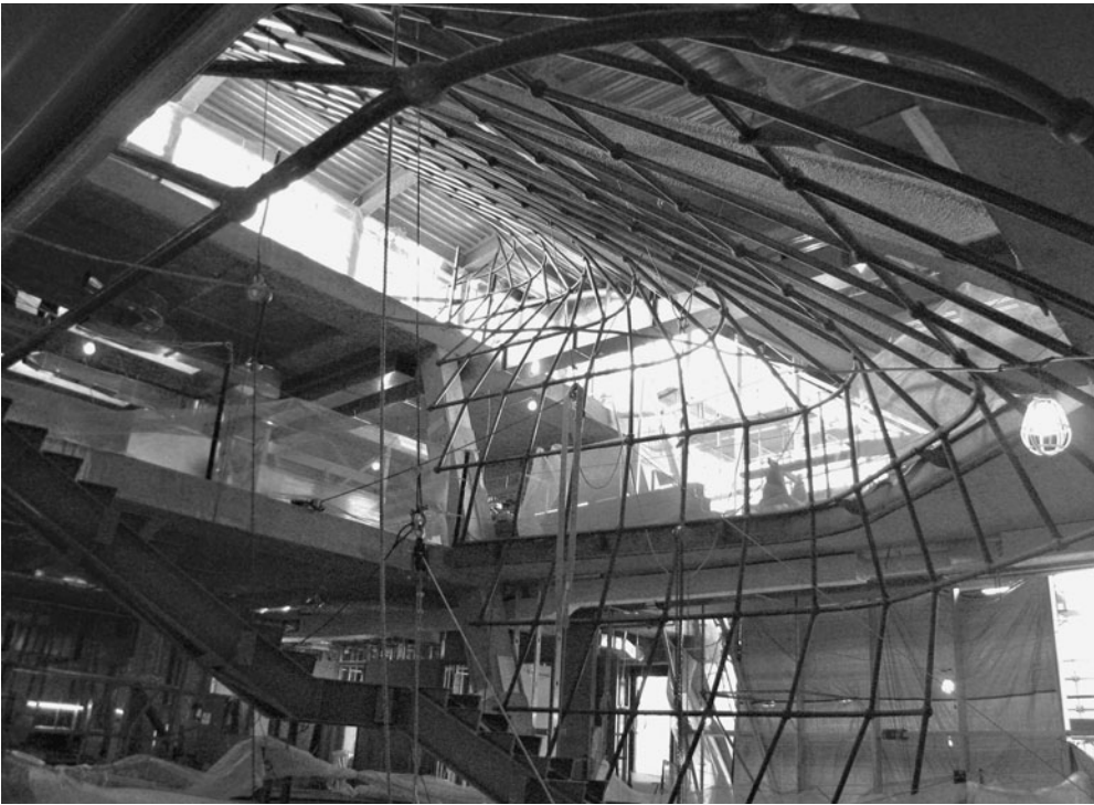
3.8 The atrium under construction. The slab edges, the connecting stairs and the installation of the steel lattice. Morphosis Architects, John A. Martin and IBE, 41 Cooper Square, New York, New York, 2009.
