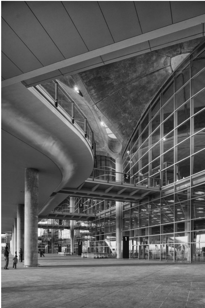
7.4 The mullions curve to reflect the domed roof. Foster + Partners, Buro Happold, Queen Alia International Airport, Amman, Jordan, 2013.
