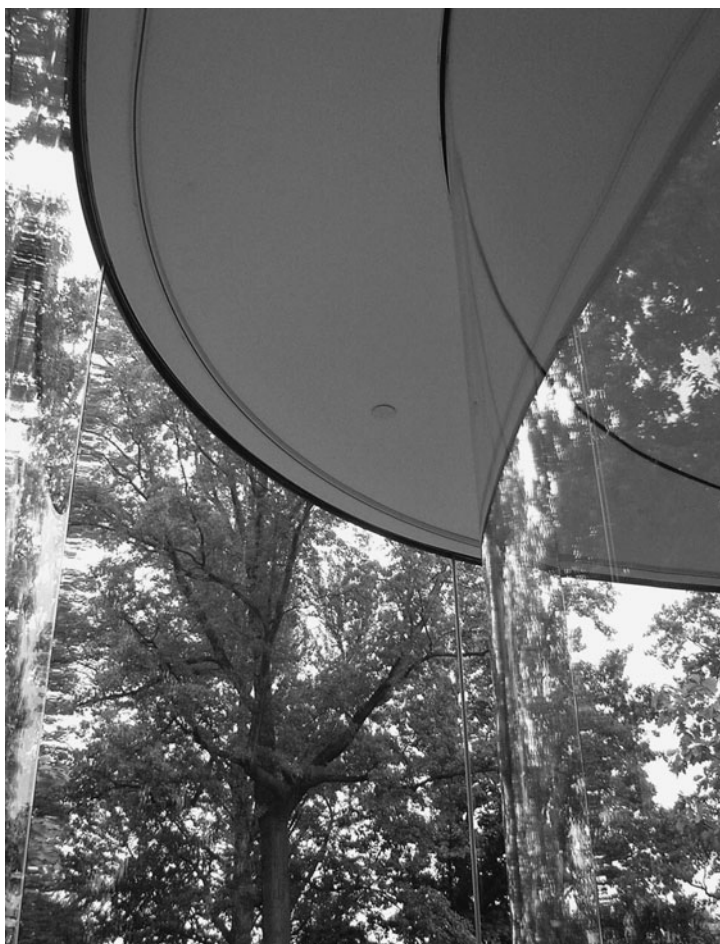
6.9 Detail. Note the high degree of precision in the detailing where the glass walls meet the roof. SANAA & Sasaki and Partners, Glass Pavilion at the Toledo Museum of Art, Toledo, Ohio, 2007.
