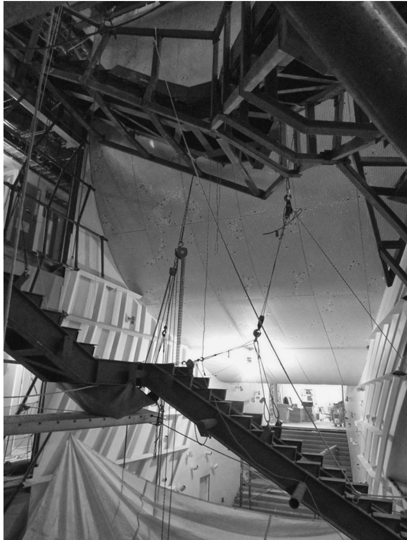
3.11 Interior being winched into place, note the perforated steel ceiling panels behind. Morphosis Architects, John A. Martin and IBE, 41 Cooper Square, New York, New York, 2009.
