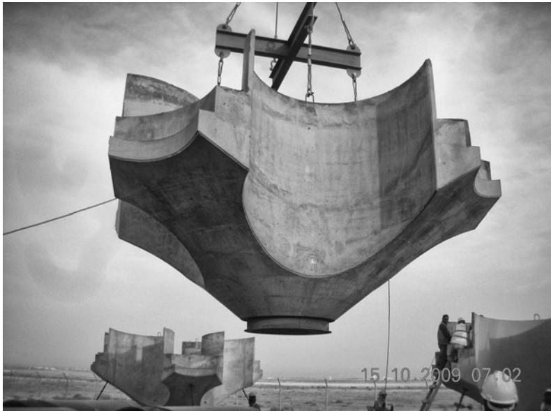
7.5a and b Precast components craned to the site. Foster + Partners, Buro Happold, Queen Alia International Airport, Amman, Jordan, 2013.
