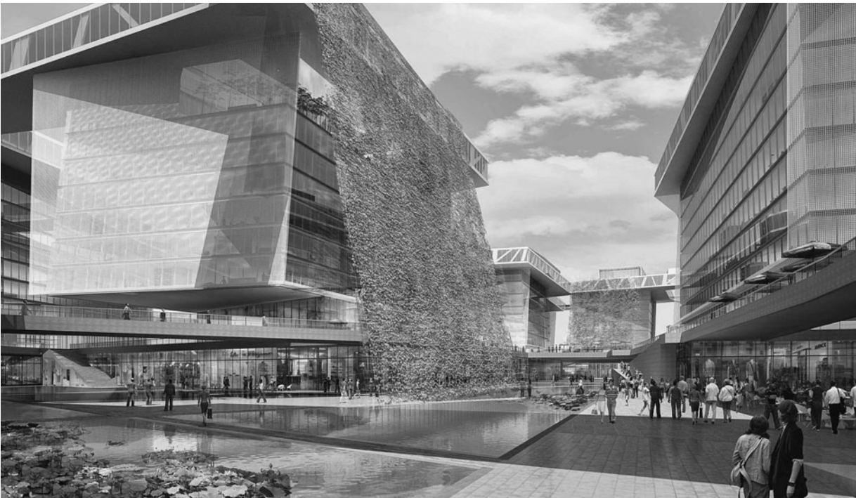
10.5 The bio-filtration veil: Hydroponic plants systems developed in collaboration with researchers at Rensselaer Polytechnic Institute to cleanse the air and the water. SPG Shanghai, SOM, Shanghai, China, 2010.
