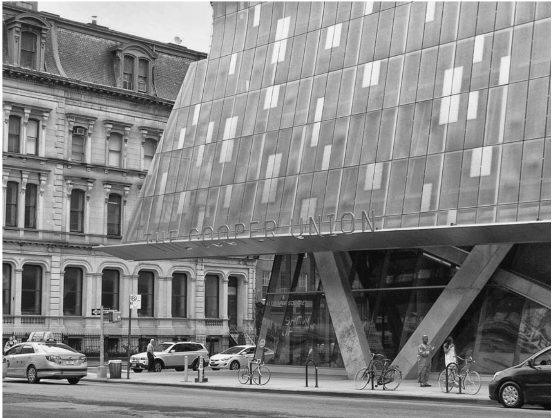
3.7 Note the column-free corner. Morphosis Architects, John A. Martin and IBE, 41 Cooper Square, New York, New York, 2009.
