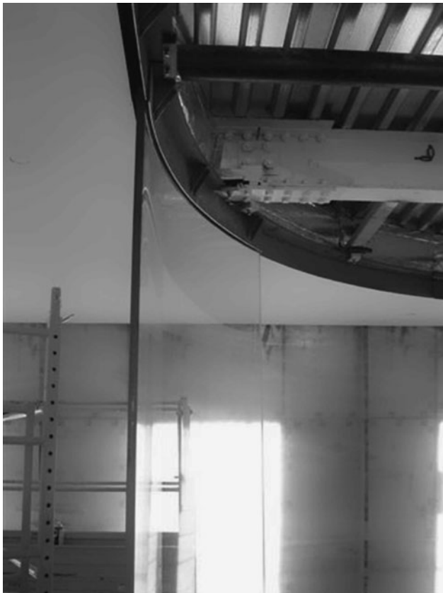
6.7 Glass installation. Note the very shallow available space between the underside of the roof deck and the underside of the ceiling where the mechanical systems had to be carefully inserted. SANAA & Sasaki and Partners, Glass Pavilion at the Toledo Museum of Art, Toledo, Ohio, 2007.
