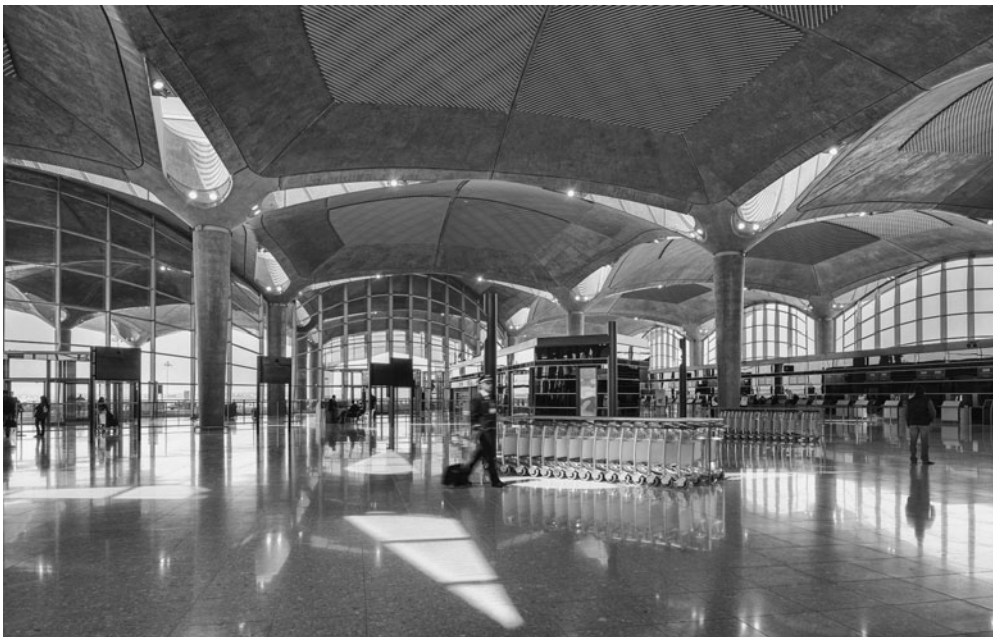
7.6 Interior view showing the openness afforded by the umbrella structures. Foster + Partners, Buro Happold, Queen Alia International Airport, Amman, Jordan, 2013.
