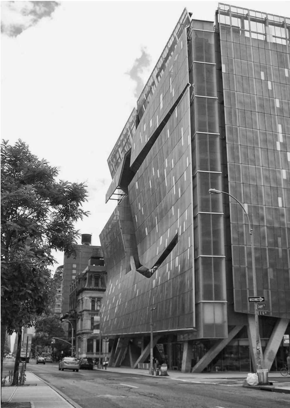
3.10 The translucent stair tower on the south west corner of the building. Morphosis Architects, John A. Martin and IBE, 41 Cooper Square, New York, New York, 2009.
