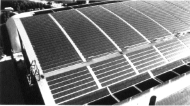
(Top) Figure I-2a. Rooftop photovoltaic panels will play a key role in on-site power generation. The natatorium of the Georgia Institute of Technology in Atlanta uses 32,750 square feet of solar panels. (Photo: Solar Design Associates)
