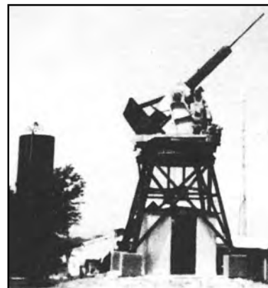
Fig 1—An aggressive approach to steering a giant EME antenna—a 5-inch gun turret from a destroyer.
