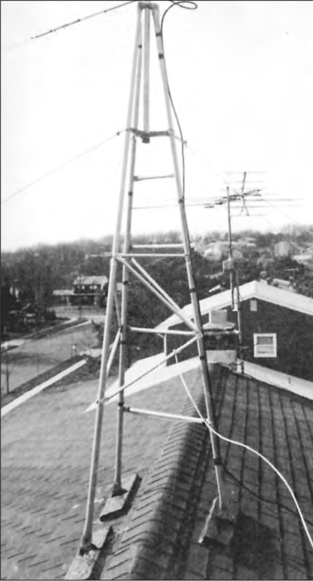
Fig 42 —This tripod tower supports a rotary beam antenna. In addition to saving yard space, a roof-mounted tower can be more economical than a ground-mounted tower. A ground lead fastened to the lower part of the frame is for lightning protection. The rotator control cable and the coaxial line are dressed along two of the legs. ( Photo courtesy of Jane Wolfert )
