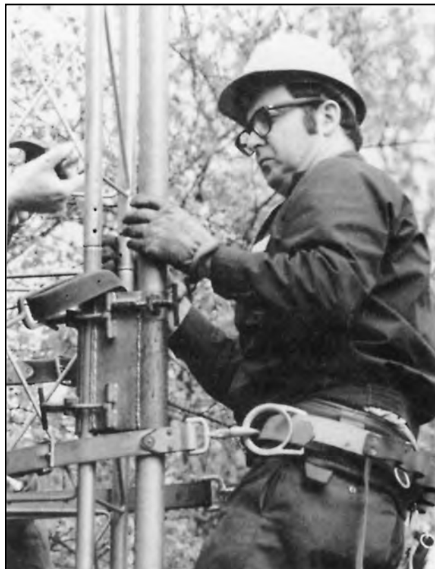
Fig 1 —Bill Lowry, W1VV, uses a good quality safety belt, a requirement for working on a tower. The belt should contain large steel loops for the strap snaps. Leather loops at the rear of the belt are handy for holding tools. (Photo by K1WA)
