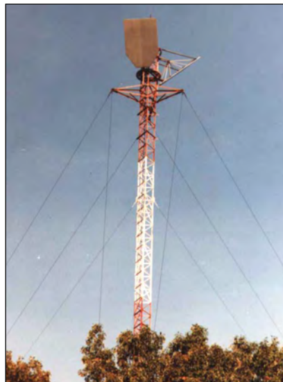
Fig 73— Commercial periscope antennas, such as this one, are often used for point-to-point communication.
