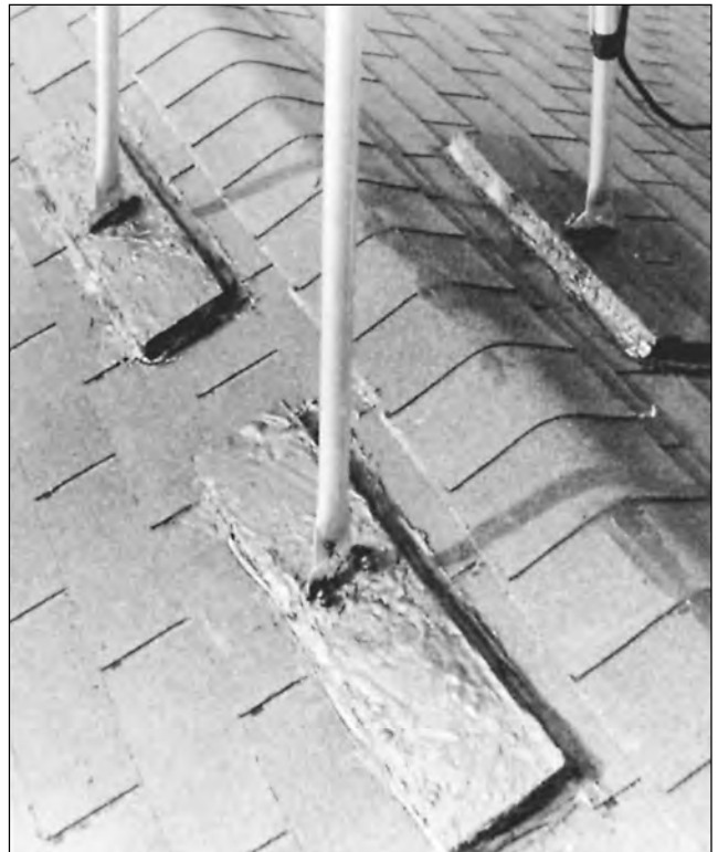
Fig 44 —Three lengths of 2 × 6 wood mounted on the outside of the roof and reinforced under the roof by three identical lengths provide a durable means for anchoring the tripod. A thick coat of roofing tar guards against weathering and leaks.
