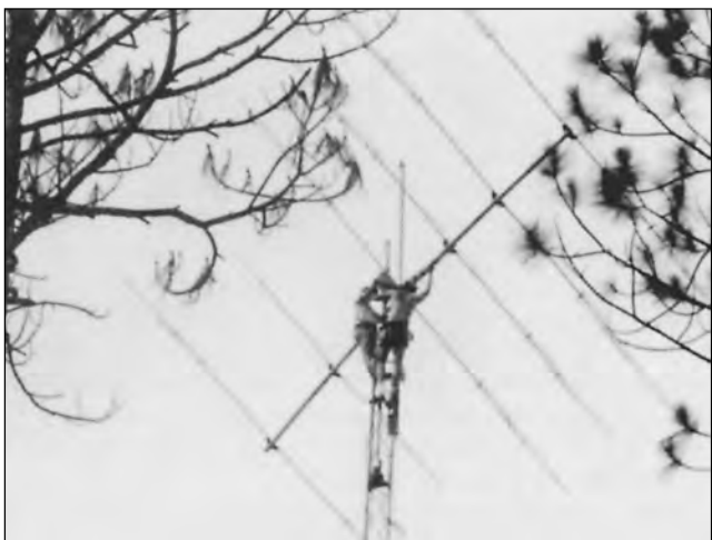
Fig 41—The U bolts securing the short pipe to the mast plate are loosened and the boom is turned to a horizontal position. This puts the elements in a vertical plane. Then the pipe U bolts are tightened and pinning bolts secured. The boom U bolts are then loosened and the boom turned axially 90°.
