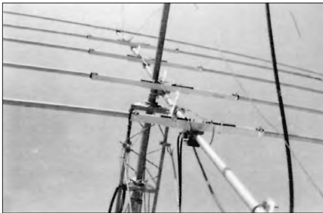
Fig 33 —The attachment of the elements to the boom.
