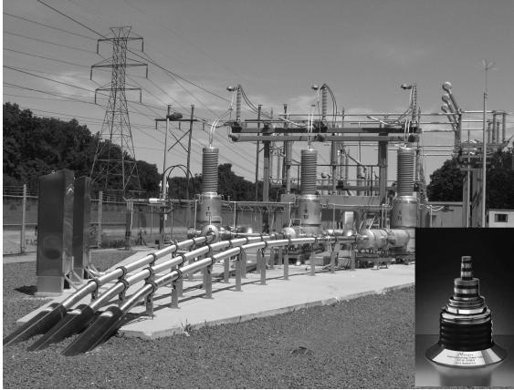
9.22 Terminations for the three phases of the LIPA cable produced by Nexans and AMSC. The installation is on Long Island in New York. The inset shows a cross-section of the cold dielectric cable.
