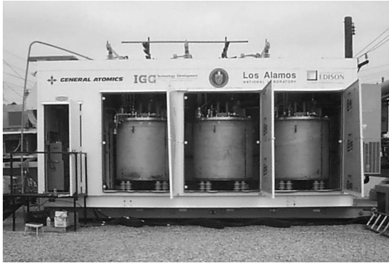
9.4 A transportable fault current controller at the substation in Los Alamos. The picture was taken during testing that occurred after repair of the damage caused by electrical arcing during the initial tests at SCE. (Source: Los Alamos National Laboratory.)
