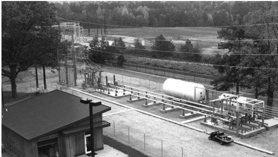
9.23 The first long term superconducting cable installation at the Southwire facility. Southwire is a producer of copper conductors for transformers, cables, etc. This three-phase cable installation delivered power to the plant for over 26 000 h.
