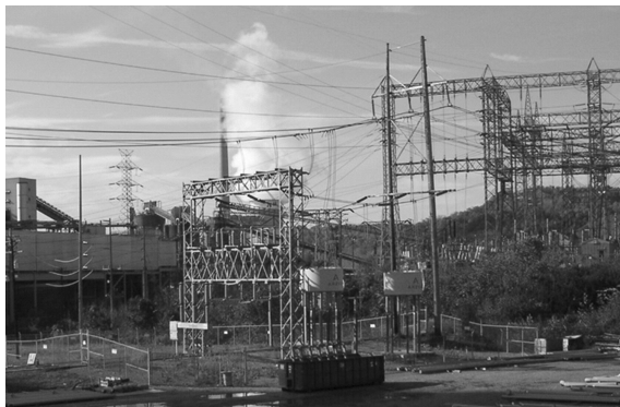
9.2 Three reactors in elevated tanks (one is hidden from view) at the TIDD substation on the AEP power grid. The tanks for these reactors are live, i.e., one terminal of the reactor is tied to the case or tank. The TIDD substation was chosen by AEP, Zenergy, and the US Department of Energy (DOE) for the demonstration of a high-voltage superconducting FCL
