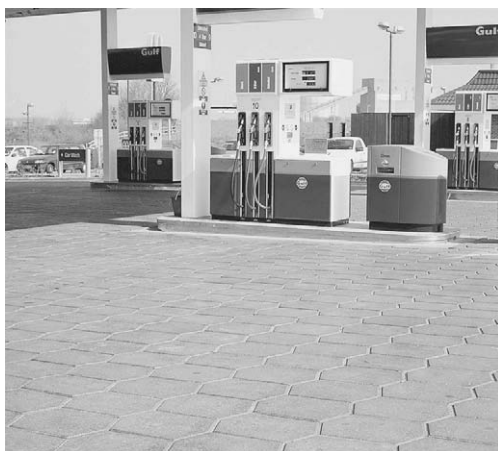
FIGURE 10.3 Segmental paving used to resist petroleum spillages.
