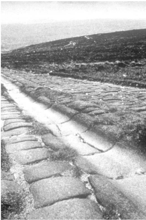
FIGURE 10.1 Roman segmental pavement in the United Kingdom.
