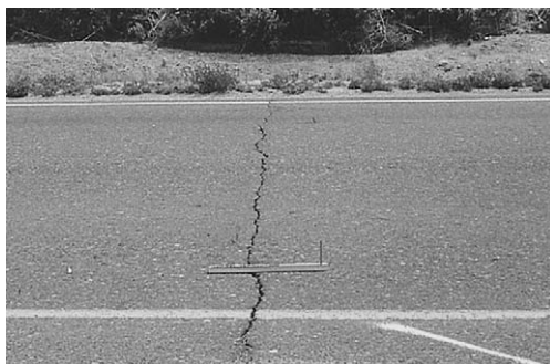
FIGURE 8.8 Thermal cracking.
