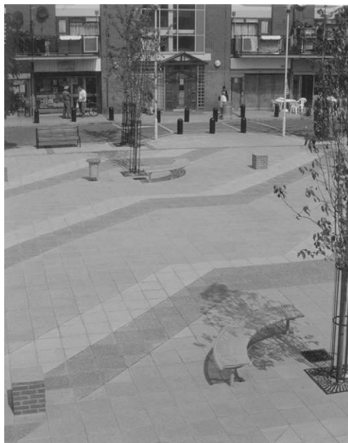
FIGURE 10.6 Lightly trafficked pedestrian area.
