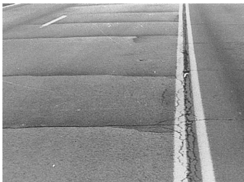
FIGURE 8.13 Reflection cracking.
