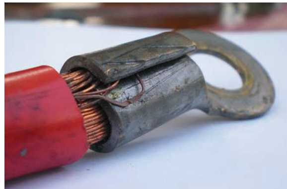
It is very important that the battery terminal lugs are perfectly crimped. I could pull Roobarb's old lugs right off.
