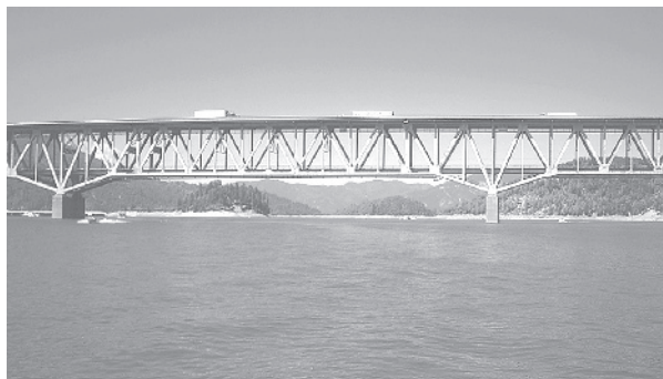
An example of a Warren truss (with verticals). See page 103.
