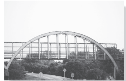
This three-hinged truss arch is used to support a pedestrian walkway. This bridge is referred to as a “through-arch bridge.”
