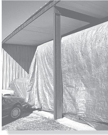
Wide-flange members are often used for columns. Here is an example of a beam column.
