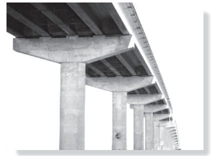
These hammerhead piers are tapered due to the greater shear and moment they must resist at their center.
