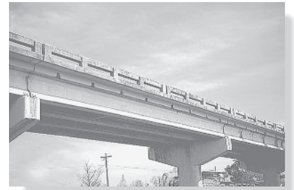
The prestressed concrete girders are simply supported on the piers and are used for this highway bridge.
