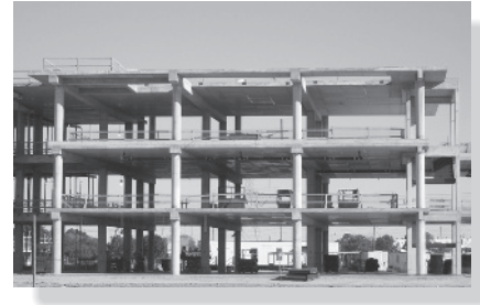
This statically indeterminate concrete building frame can be subjected to sidesway due to wind and earthquake loadings.
