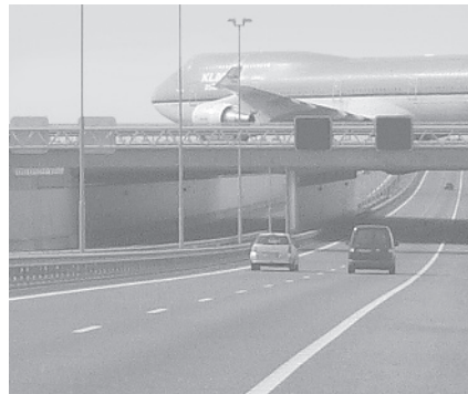
The girders of this bridge must resist the maximum moment caused by the weight of this jet plane as it passes over the bridge.
