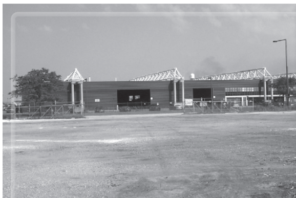
The roof of this building is supported by a series of space trusses.
