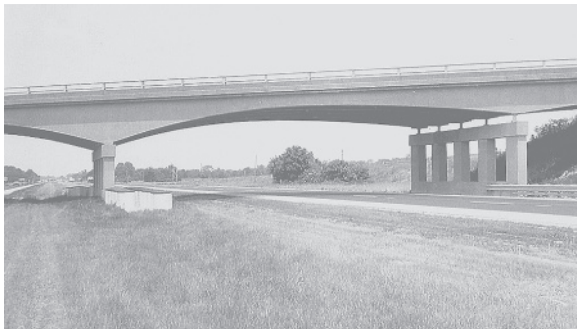
A continuous, reinforced-concrete highway bridge.
