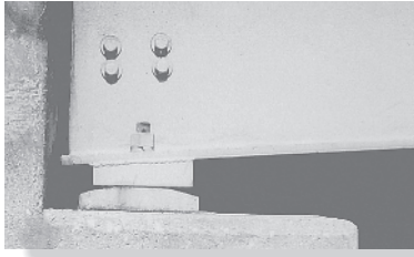
A typical rocker support used for a bridge girder.
