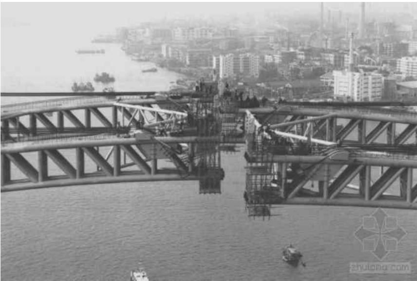
Figure 9.12 (Continued) Vertical and horizontal rotation of Yajisha Bridge. (Courtesy of Guizhou Bridge Construction Group Ltd.) (c) Half of the main arch is rotating horizontally to meet the bridge axis. (d) Before closure.
