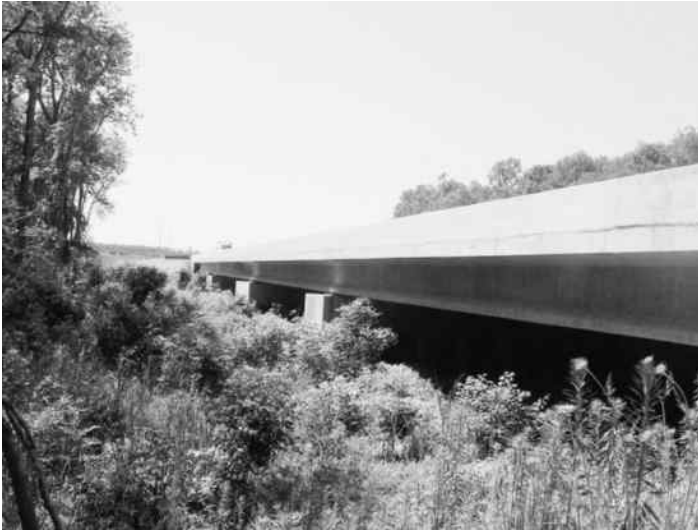
Figure 5.32 US23043 Bridge, Maryland.
