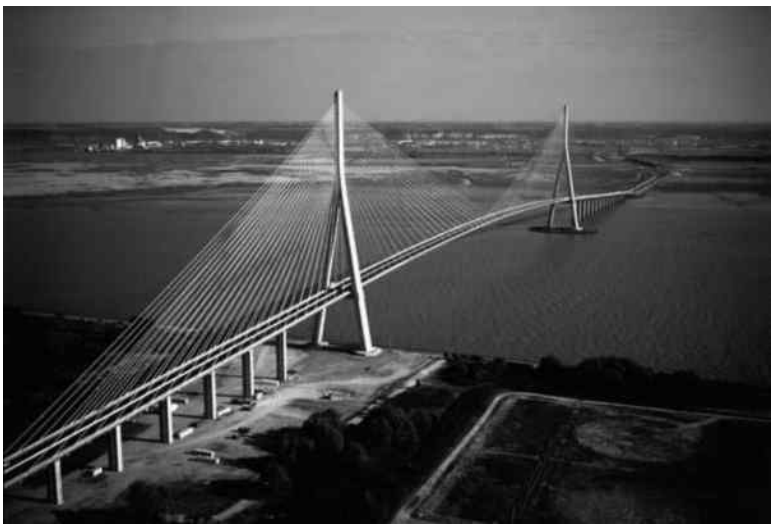
Figure 11.3 A cable-stayed bridge with auxiliary piers.
