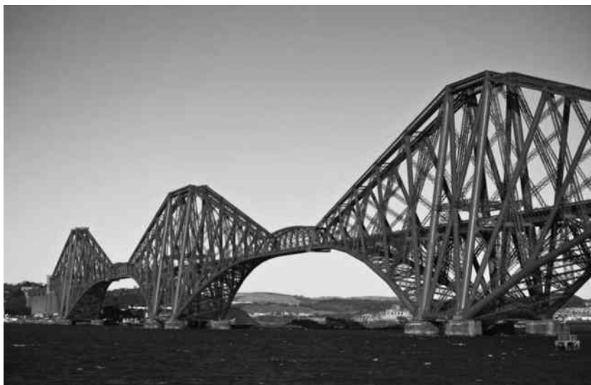
Figure 10.7 Forth Rail Bridge, Queensferry, Scotland.
