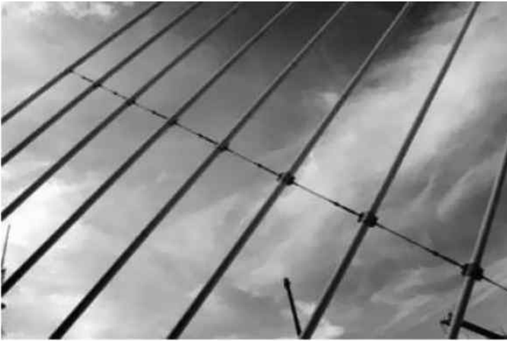
Figure 11.7 Crosstie of cables.
