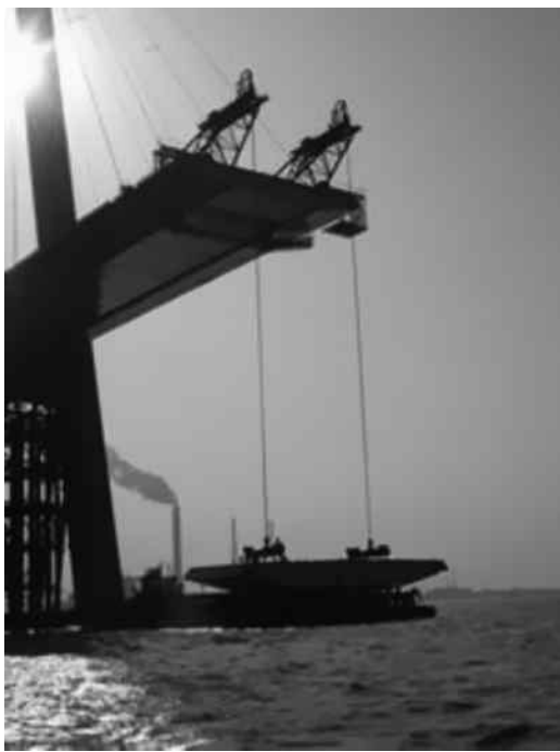
Figure 11.11 Lifting and erecting of one segment.
