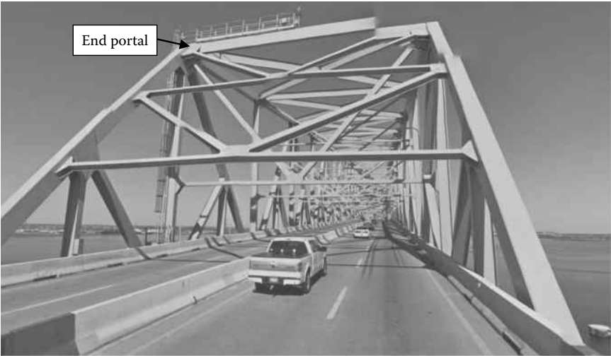
Figure 10.27 End portal of Francis Scott Key Bridge.
