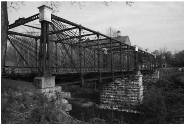
Figure 10.2 Bollman truss bridge.
