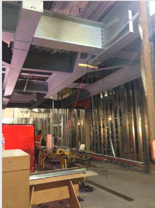
IMAGE COURTESY OF MCCARTHY BUILDING COMPANIES, INC.
