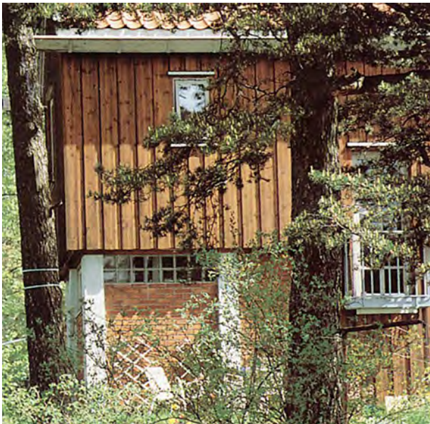
14.11 Exterior of bathroom shown in Figure 14.10. Both walls and floor consist of mineral materials only, to prevent moisture damage. Perlite is used as thermal insulation. Gaia Lista, 1996.
