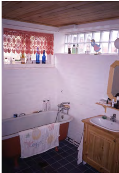
14.10 Porous brick with lime rendering balancing humidity in a bathroom. Hydraulic lime mortar is used to improve the potential for re-use of bricks. Gaia Lista, 1996.
