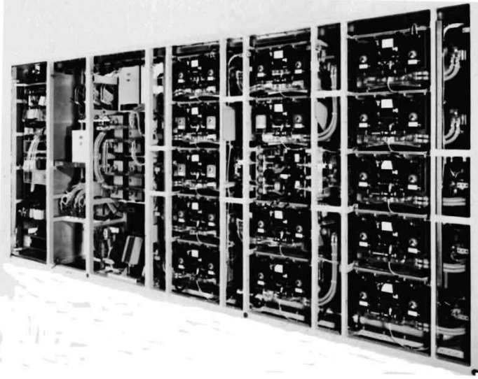
Fig. 6.38: GTO-thyristor converter scaffold for one bogie of “Euro-Sprinter” (Siemens AG, A&D)
