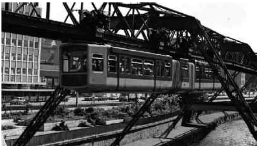
Fig. 12.6: Wuppertal suspension railway
