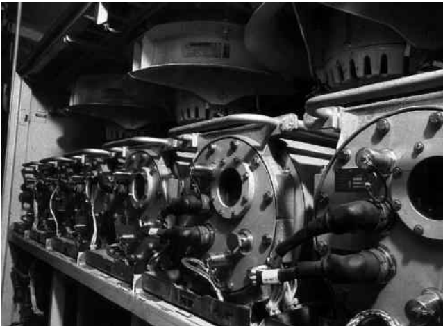
Fig. 7.10: Evaporative-cooled thyristor converters of TGV-A (Alstom Transports)
