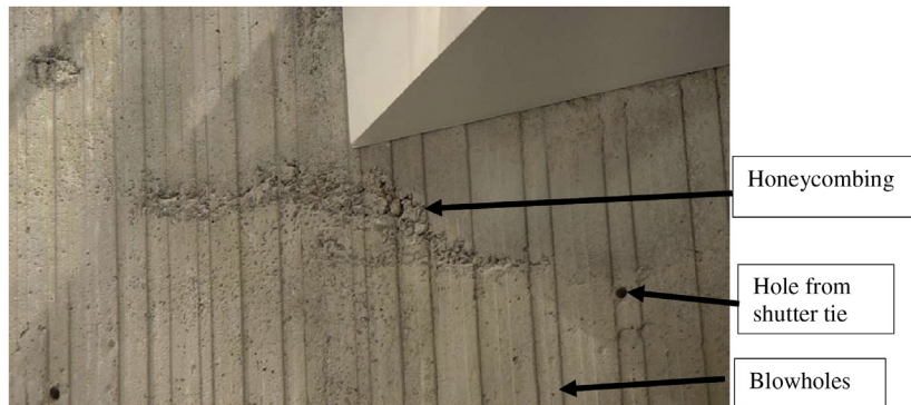
FIGURE 26.4 Defects in Concrete Surface
