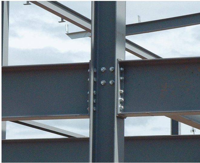
FIGURE 30.11 A Typical Bolted Joint in a Steel Frame
