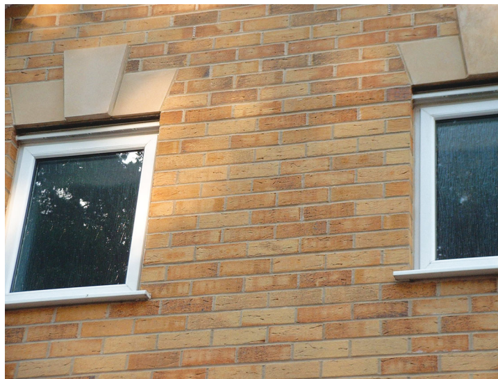
FIGURE 34.8 Well Planned Brickwork
