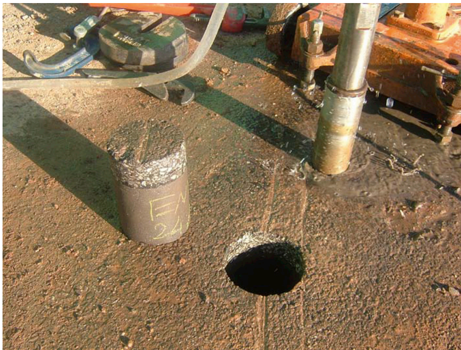
FIGURE 27.7 Core Recovered From Road Slab
