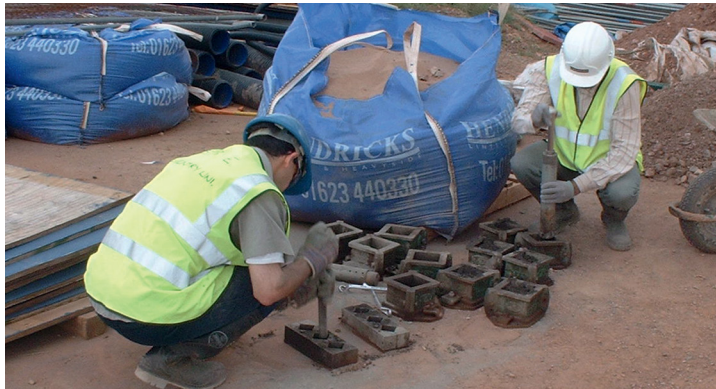
FIGURE 22.11 Compacting Test Cubes on Site
