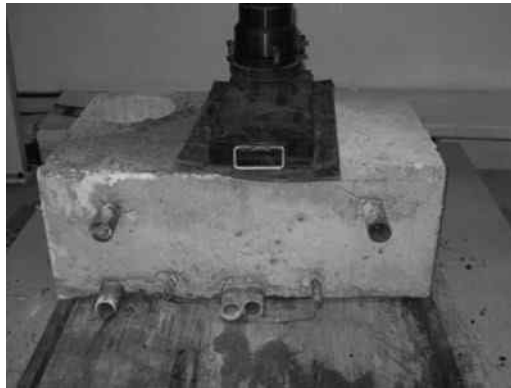
Figure 10.17 The W-type power supply rail of the 3G OLEV being tested. © 2015 IEEE. Reprinted with permission from Choi et al. (2015c)
