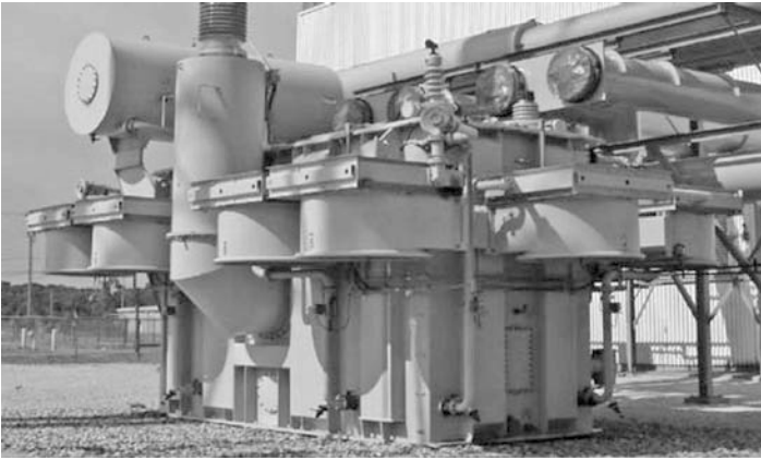
FIGURE 5.9 Generator step-up transformer
