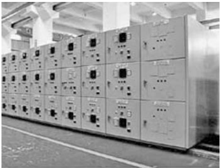
FIGURE 7.1 Medium-voltage switchgear
