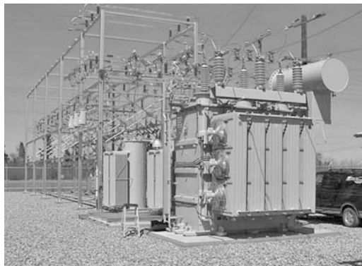
FIGURE 5.7 Conservator tank design
