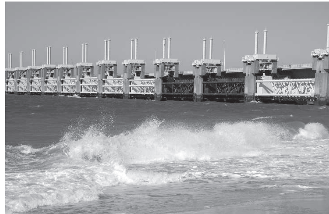
Storm Surge Gates in Holland Dam.
