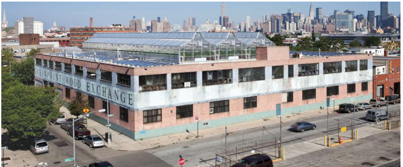
Figure 6.36 The rooftop site demonstrates a new use for what is usually nonproductive areas while taking advantage of sun exposure.
