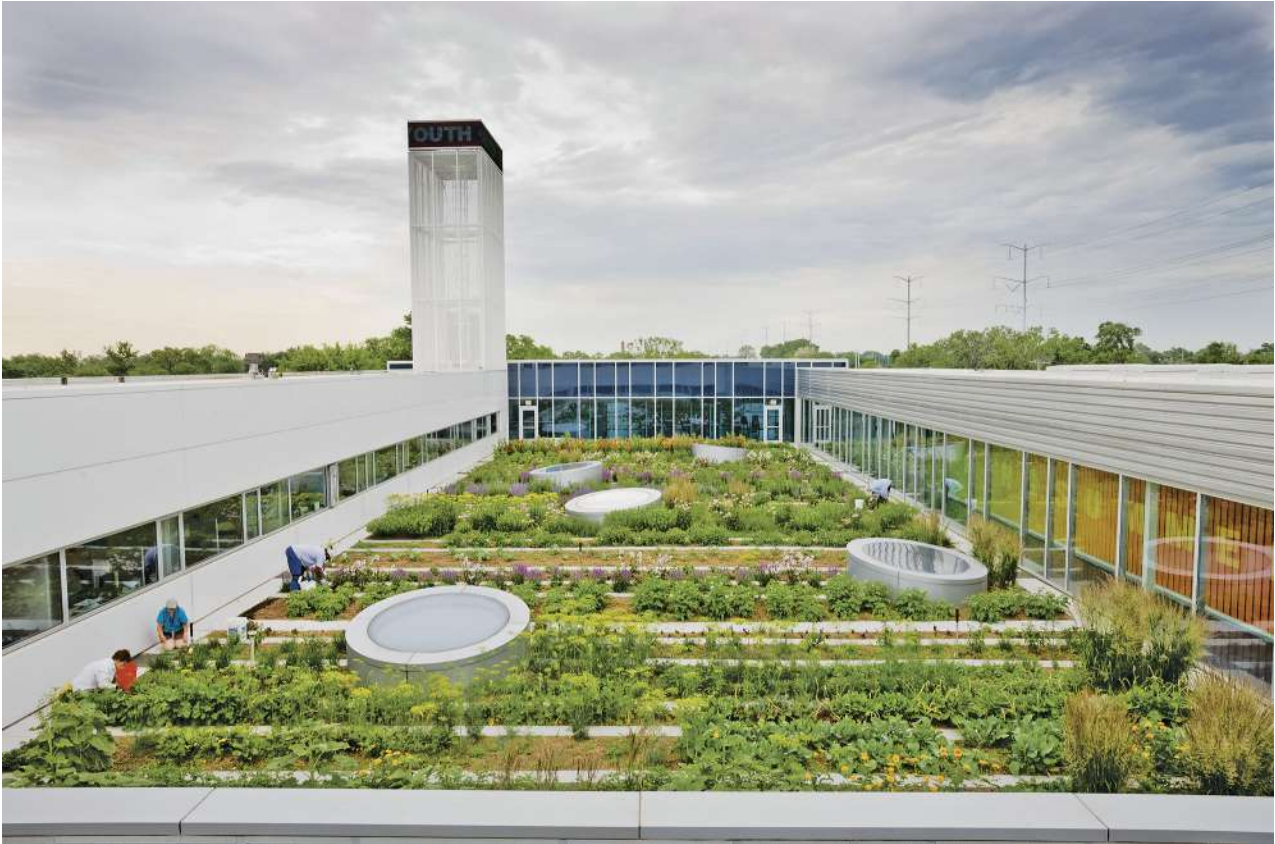
Figure 3.24 The rooftop garden at the Gary Comer Youth Center, Chicago, Illinois.
