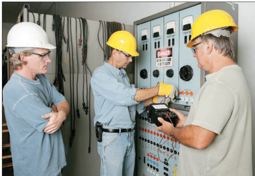
FIGURE 1-5 Electricians making a measurement.
