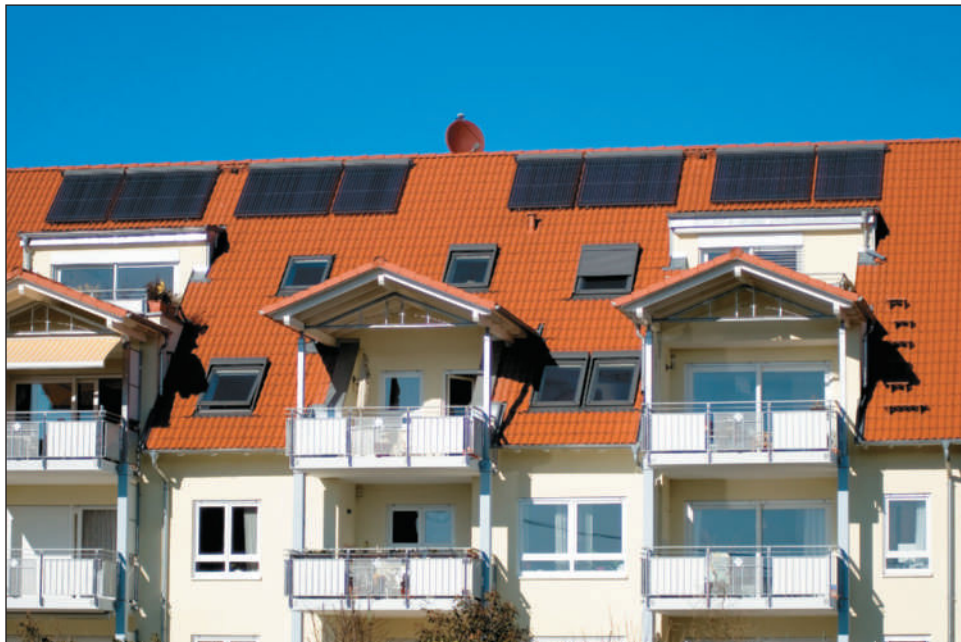
FIGURE 15-4 PV arrays mounted on a house.
