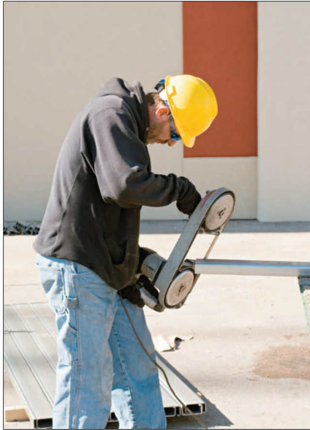
FIGURE 9-25 A portable bandsaw being used at a jobsite.
