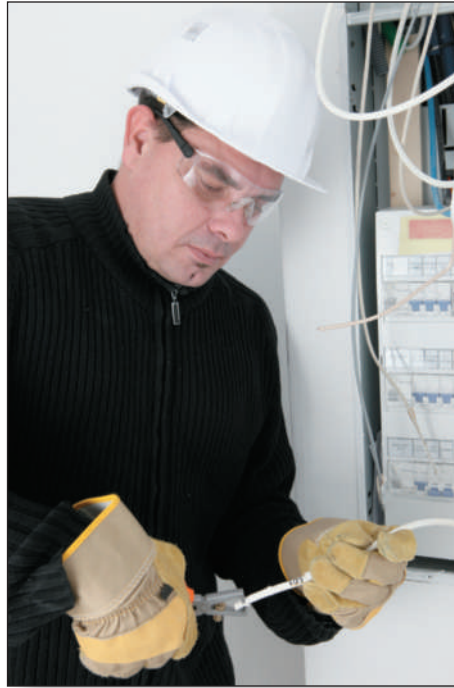
FIGURE 1-4 An electrician at work.
