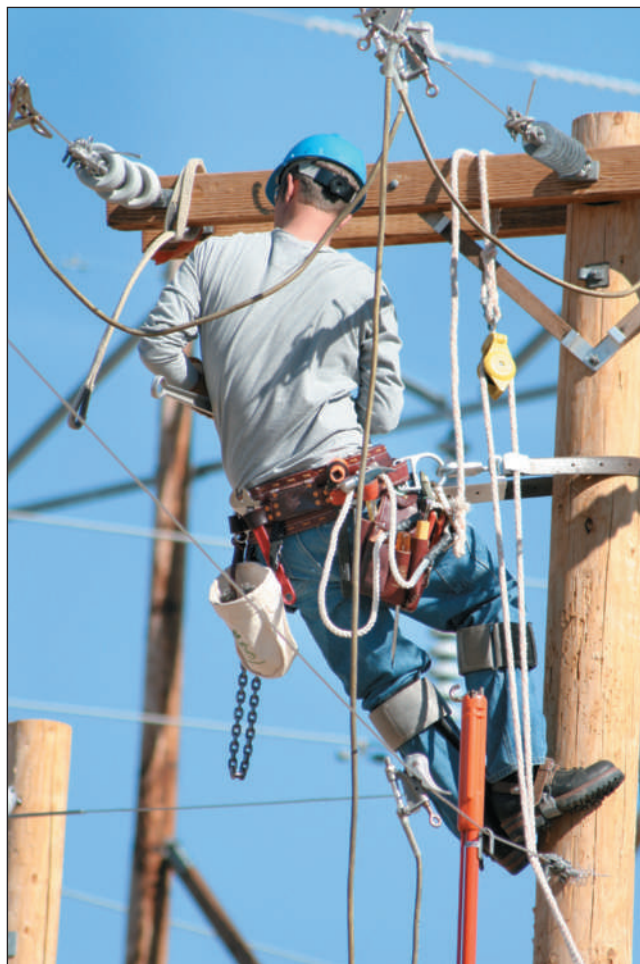
FIGURE 1-13 Lineman working on power lines.
