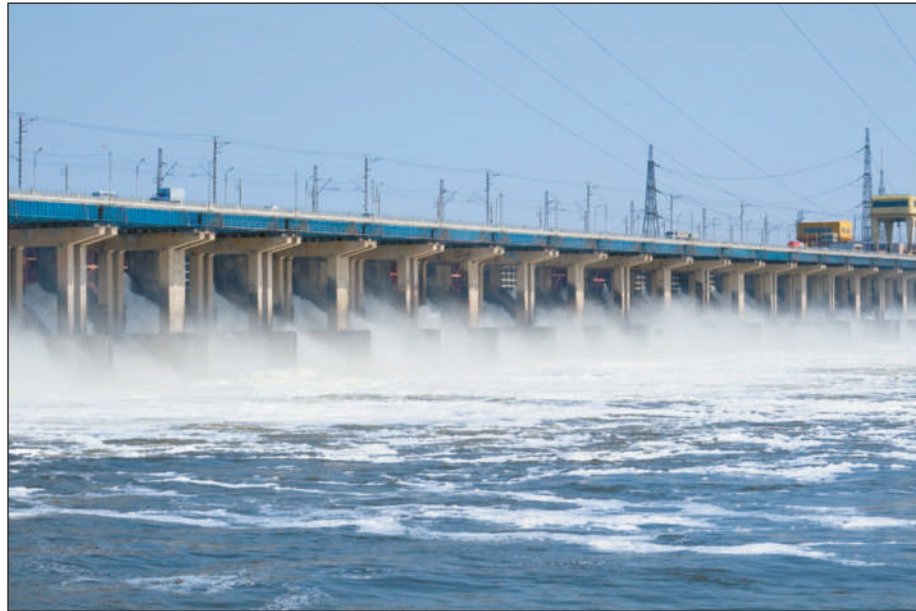
FIGURE 15-12 A hydroelectric power station on a river.
