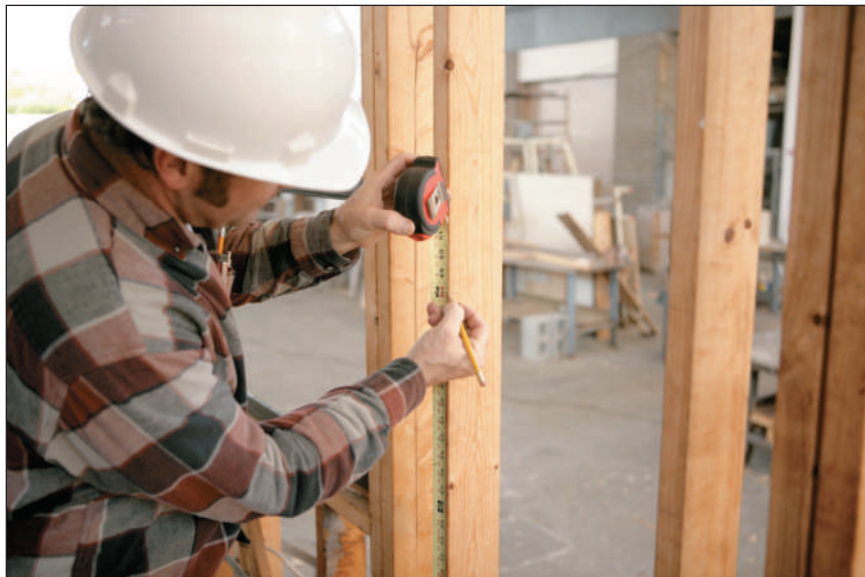
FIGURE 1-10 A construction electrician measuring to install a switch box.
