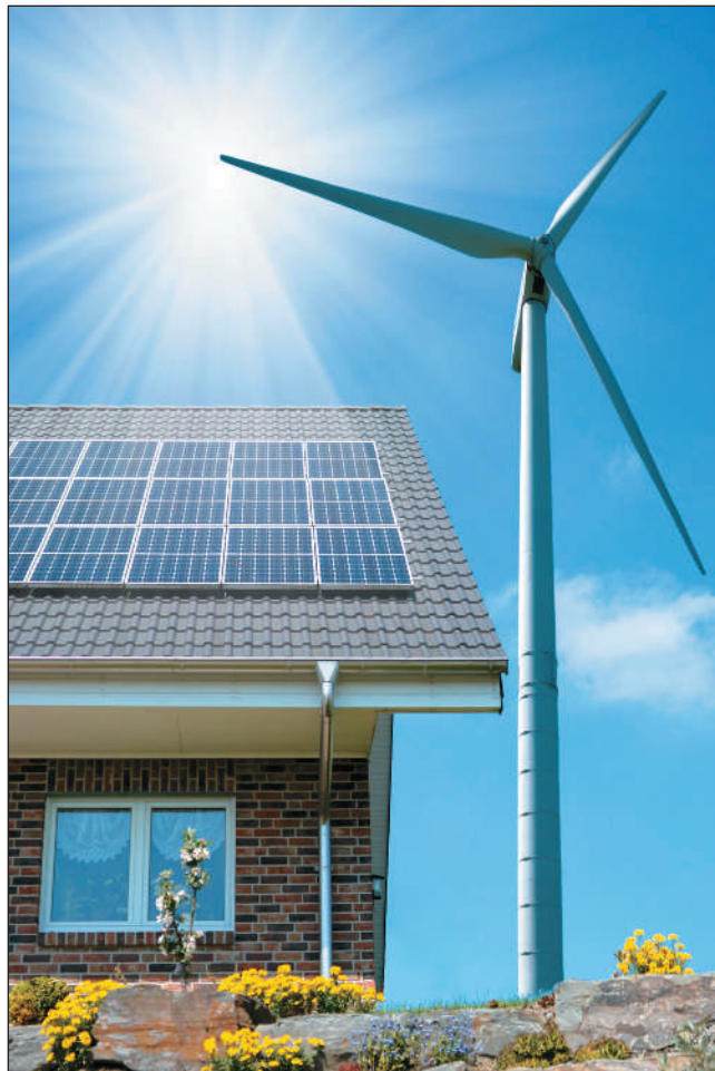
FIGURE 15-8 A roof with solar panels, and a wind turbine next to the dwelling.
