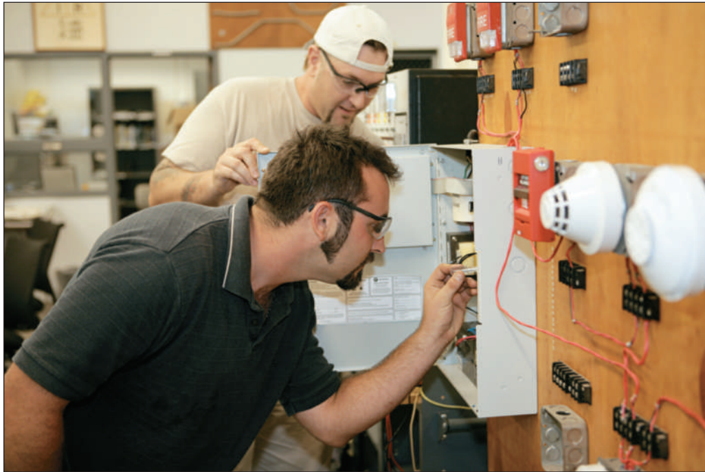
FIGURE 2-1 A journeyman and an apprentice electrician.
