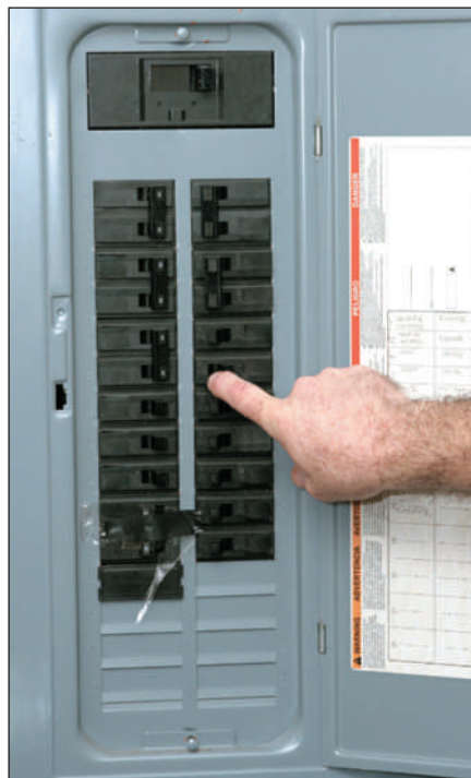
FIGURE 1-9 Circuit-breaker panel.
