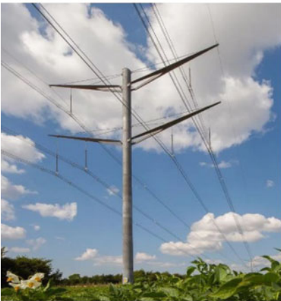
Fig. 1.3 Examples of aesthetical transmission pylon concepts, a Eagle pylon configuration proposed by Bystrup company, b Flower pylon configuration proposed by Gustafson Porter with Atelier One and Pfisterer
