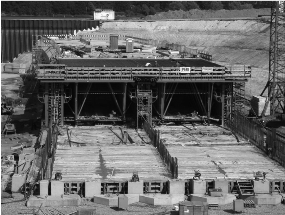
Figure 2.26 Assembly of tunnel segments
