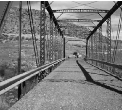
FIGURE 8.10 San Miguel Bridge deck. The deck, believed to have been installed in 1964, consists of gravel roadbase on semi-circular corrugated metal pipe segments, which bear on the bottom flanges of steel stringers. It now has a roadway of gravel on an unusual system of semi-circular lengths of corrugated metal pipe set between steel stringers. A steel vehicular rail has replaced the original railing. It served the mining industry in western Colorado until the 1980's. Abandoned since 1990, it remains the oldest bridge originally built in Colorado. (With permission from ASCE.)
