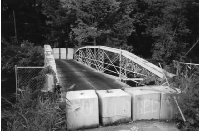
FIGURE 11.5 Berlin Iron Bridge Co. lenticular pony truss bridge.
