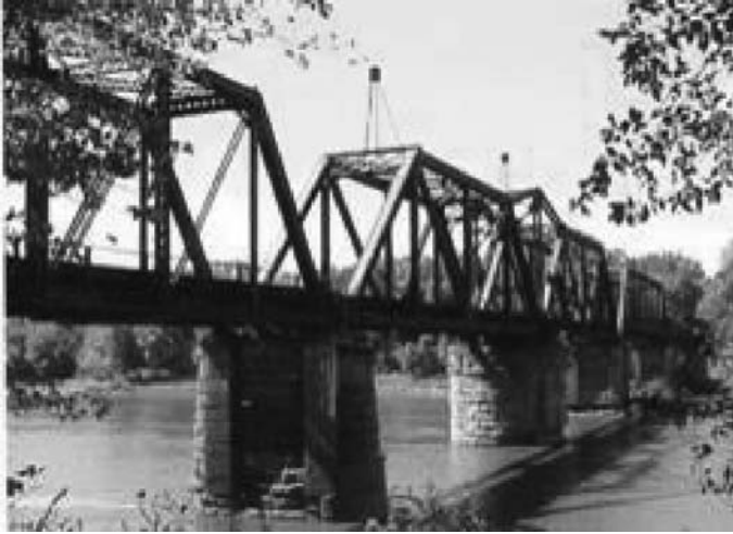
FIGURE 10.14 The Wabash Cannonball Bridge today. (P. Kennedy.)
