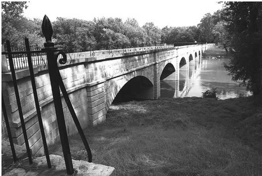
FIGURE 12.4 Completed stabilization of the Monocacy Aqueduct.
