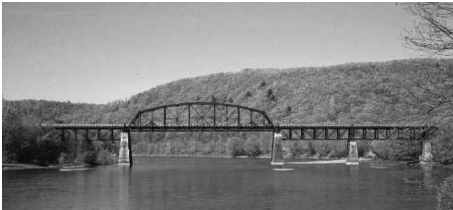
FIGURE 10.12 The Belmar Bridge across the Allegheny River. (Source: D. Alward—Venangoil website.)
