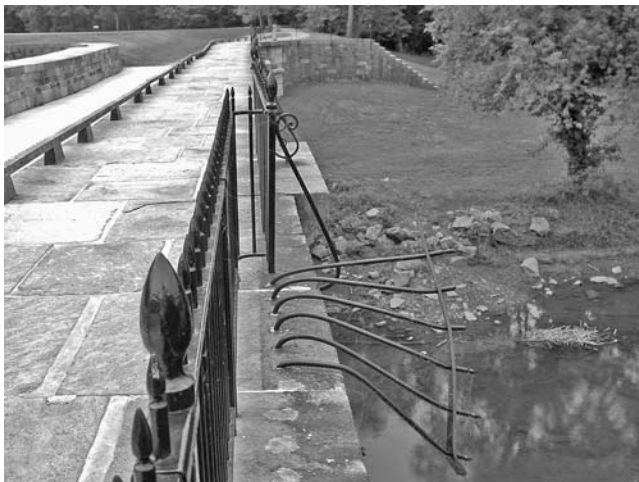
FIGURE 12.23 New and existing railing at the Monocacy Aqueduct.
