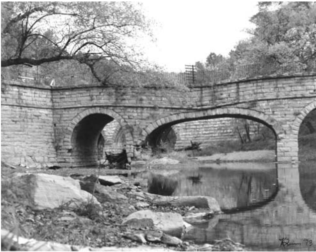
FIGURE 12.15 Hinge formations at the Catoctin Aqueduct.
