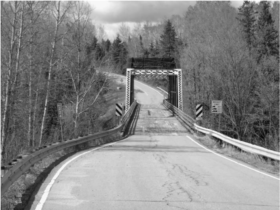
FIGURES 5.6 AND 5.7 Bridge 5721. Top: Elevation View. Bottom: View from South Approach.
