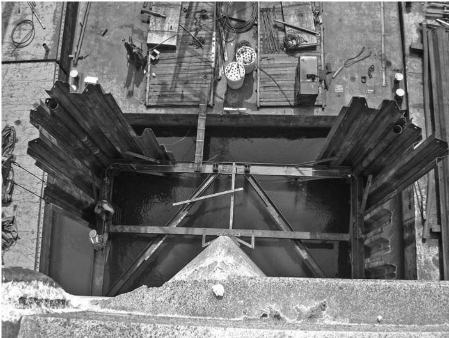
FIGURE 14.15 Pier 2, Cofferdam, 2006. (Source: Ian Engstrom, Parsons Transportation Group Inc.)
