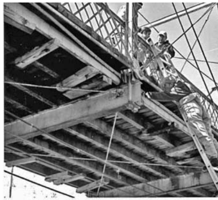
FIGURE 8.4 Blue River Bridge deck. The deck consists of longitudinal “running boards” on transverse timbers on steel stringers. The orthogonal criss-crossing of running boards and deck timbers creates a much more continuous deck than that at Fruita Bridge. The steel stringers bear on and are mechanically attached to the steel floor beams.
