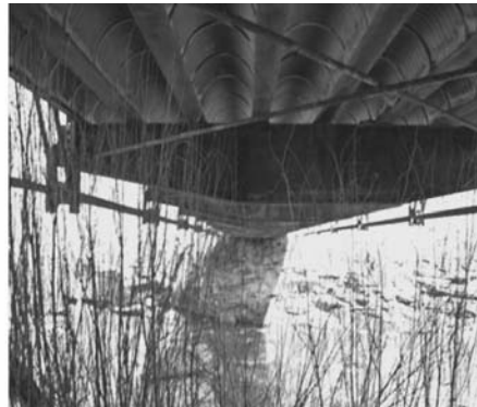
FIGURE 8.10 San Miguel Bridge deck. The deck, believed to have been installed in 1964, consists of gravel roadbase on semi-circular corrugated metal pipe segments, which bear on the bottom flanges of steel stringers. It now has a roadway of gravel on an unusual system of semi-circular lengths of corrugated metal pipe set between steel stringers. A steel vehicular rail has replaced the original railing. It served the mining industry in western Colorado until the 1980's. Abandoned since 1990, it remains the oldest bridge originally built in Colorado. (With permission from ASCE.)
