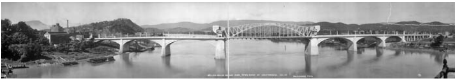
FIGURE 14.3 Million Dollar Bridge over Tennessee River at Chattanooga, August, 1917. (Courtesy of the Library of Congress, LC-USZ62-123508.)
