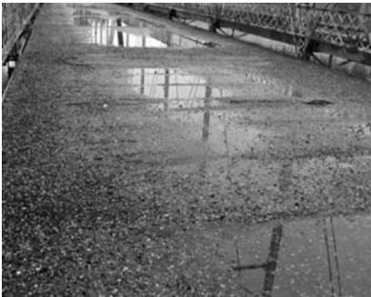
FIGURE 8.8 Rifle Bridge deck. The deck of (weathered) asphalt pavement on corrugated bridge deck on a combination of steel and timber stringers is similar to that of the Prowers Bridge.
