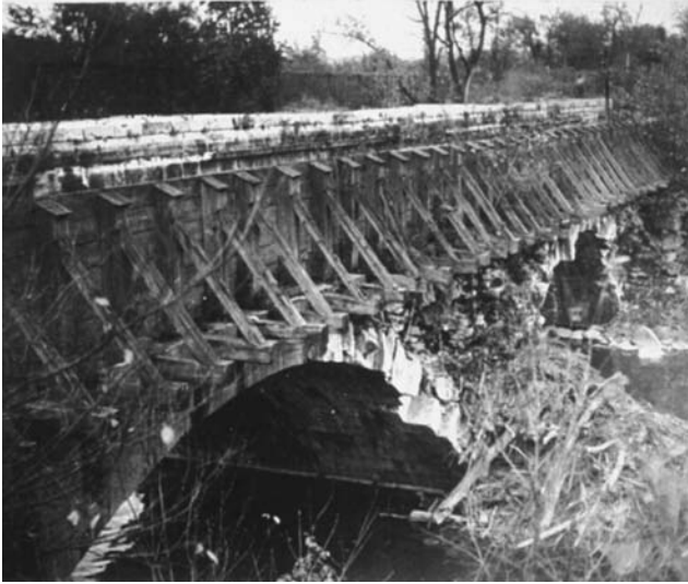
FIGURE 12.7 Wooden Wall Repairs at the Conococheague Aqueduct.
