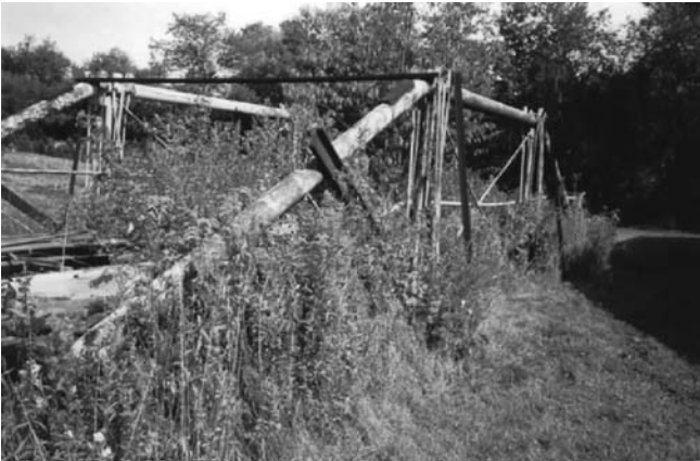
FIGURE 11.4 Ball pipe bridge as originally found.
