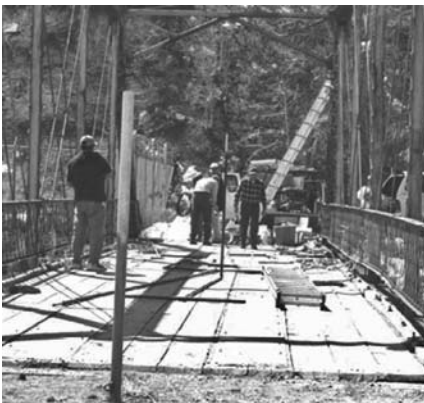
FIGURE 8.4 Blue River Bridge deck. The deck consists of longitudinal “running boards” on transverse timbers on steel stringers. The orthogonal criss-crossing of running boards and deck timbers creates a much more continuous deck than that at Fruita Bridge. The steel stringers bear on and are mechanically attached to the steel floor beams.
