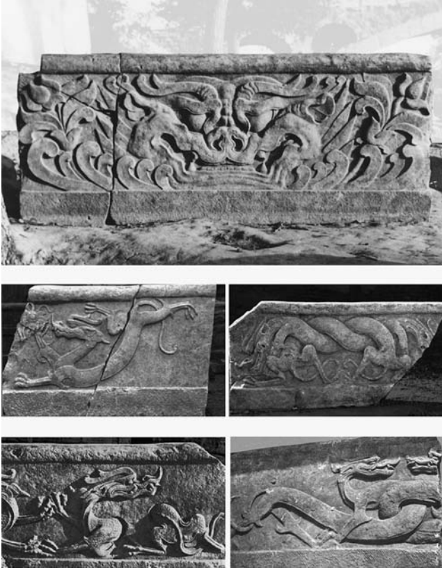
FIGURE 3.9 Original railing panels of the An Ji Bridge photographed almost immediately after they were recovered from the river bottom. Presumably, there would have been two panels like the top panel located at the center of each railing and four of each of the other panels located symmetrical with respect to the center of the bridge.
