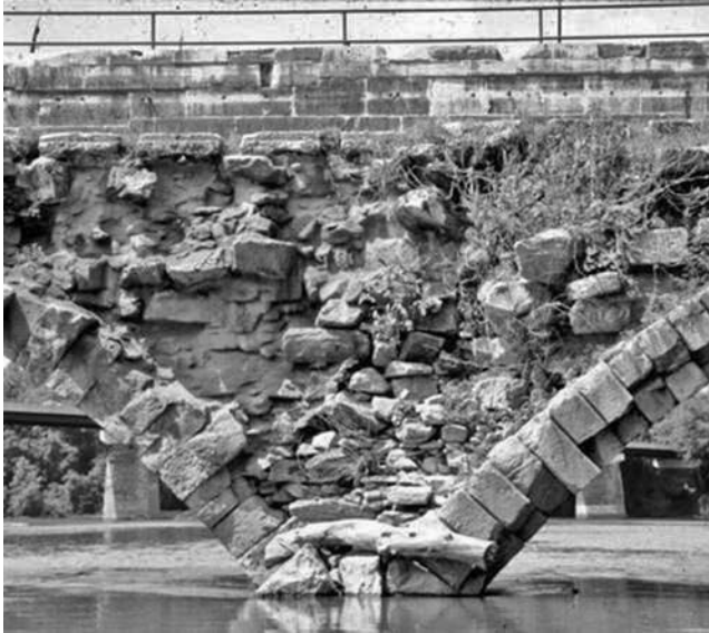
FIGURE 12.11 Interior mortared stone fill at the Conococheague Aqueduct.
