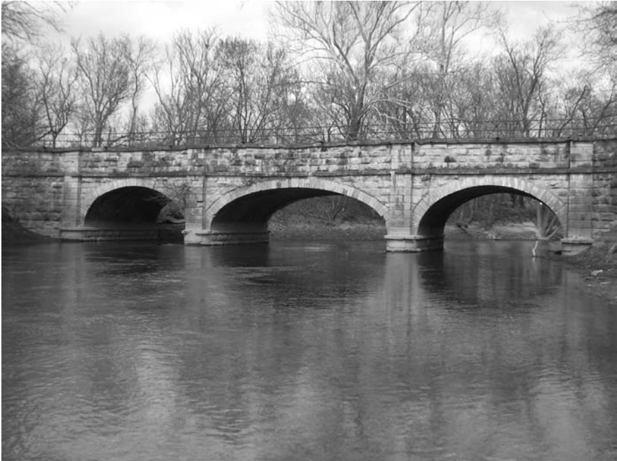
FIGURE 12.6 The Antietam Aqueduct.
