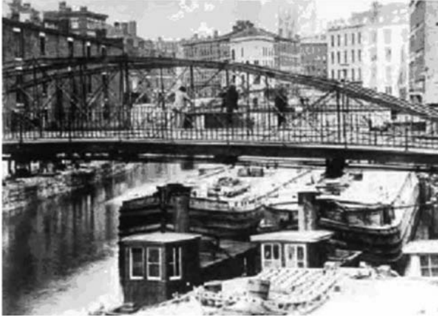
FIGURE 15.1 Circa 1870 Commercial Slip Bridge photo.
