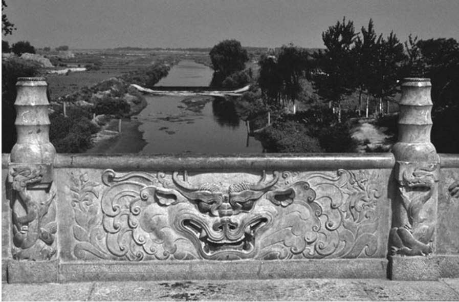
FIGURE 3.10 A fair simulation of the An Ji Bridge's original central railing panels.
