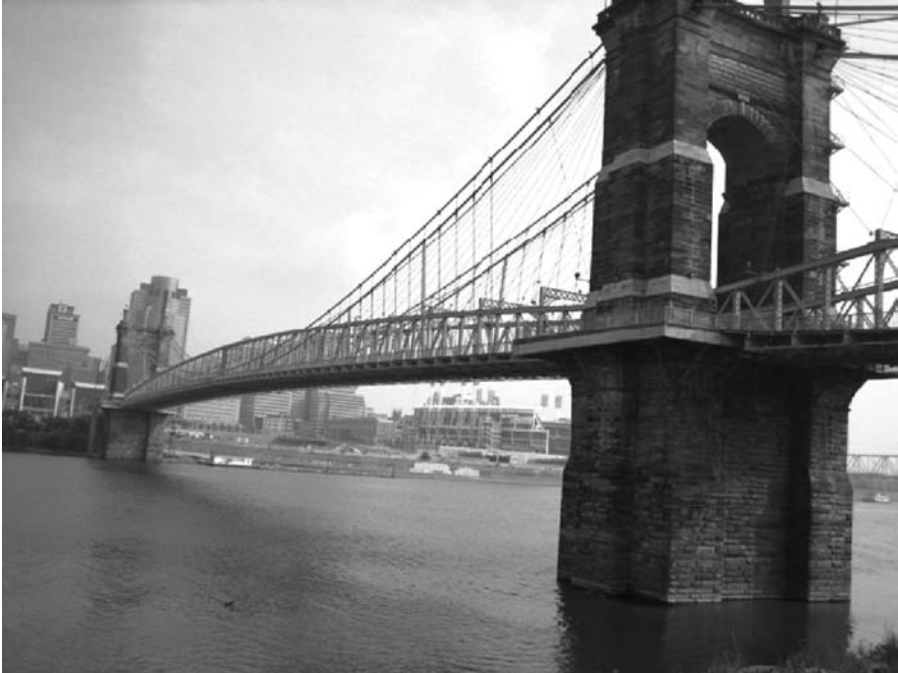
FIGURE 6.1 The John A. Roebling Bridge carries KY 17 over the Ohio River between Covington, KY, and Cincinnati, OH.
