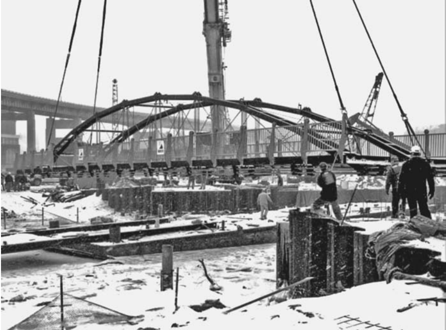
FIGURE 15.9 Lifting the bridge into its final position.
