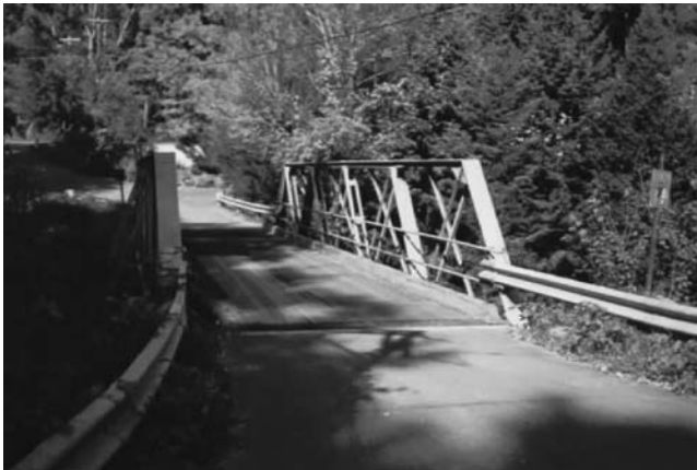
FIGURE 11.6 Bridge No. 5 while still in service.
