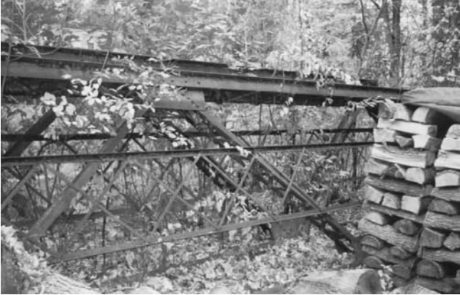
FIGURE 11.3 Trusses of Bridge No. 2 as originally found.
