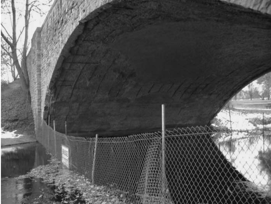
FIGURE 5.12 Phalen Park bridge (L-8560) arch soffit.
