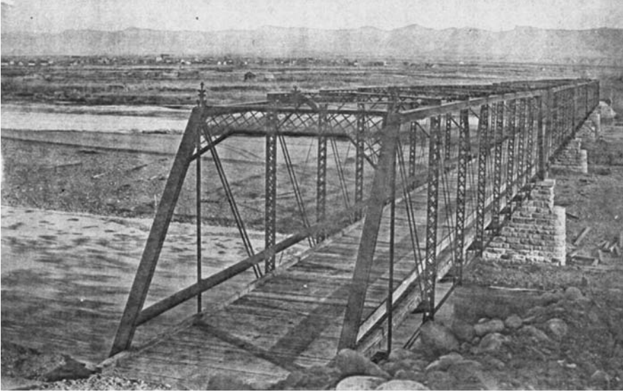
FIGURE 8.9 Fifth Street Bridge over Grand River, Grand Junction, CO. Built in 1886, one span of this five-span, wrought iron Pratt truss was relocated to the San Miguel location in the 1930's. The original timber deck and very simple, single board railing can be seen. (Photo courtesy of Museum of Western Colorado.)
