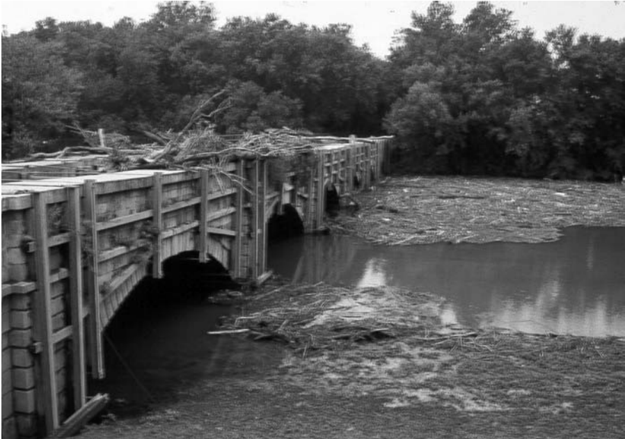
FIGURE 12.3 The Monocacy Aqueduct with steel bracing and flood debris.
