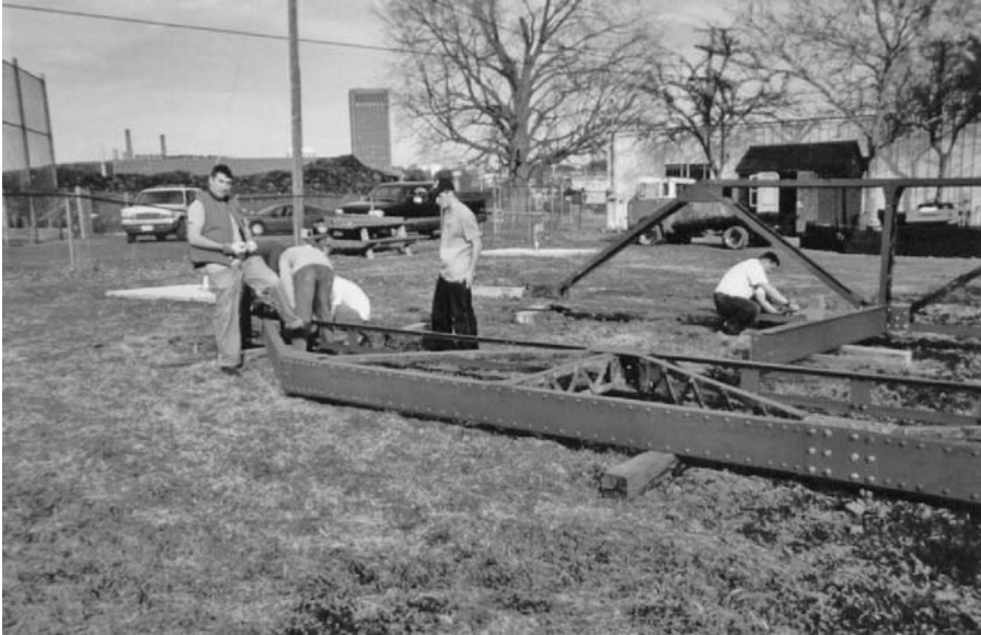
FIGURE 11.12 Students performing trial assembly of trusses and beams.
