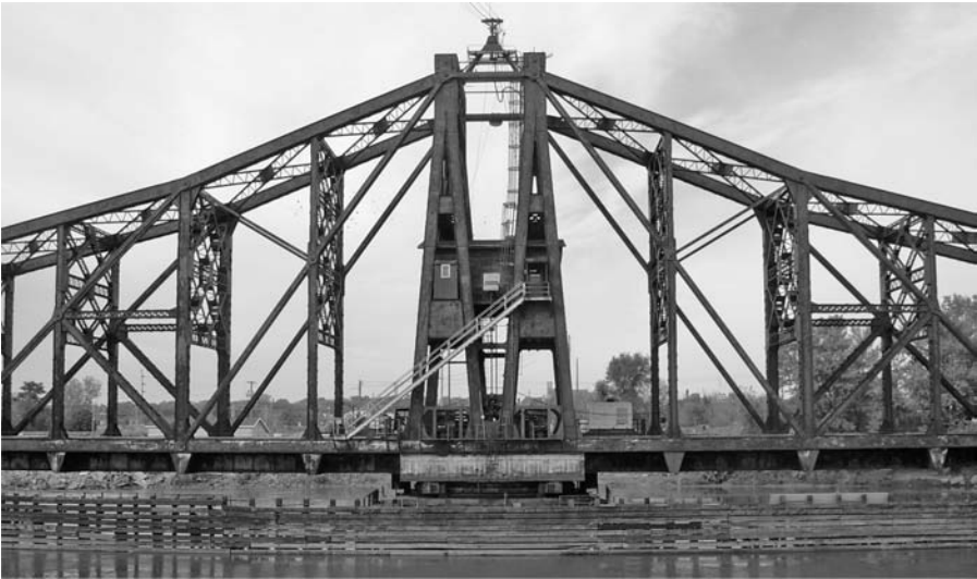
FIGURE 2.14 Third swing span in fully-open position.
