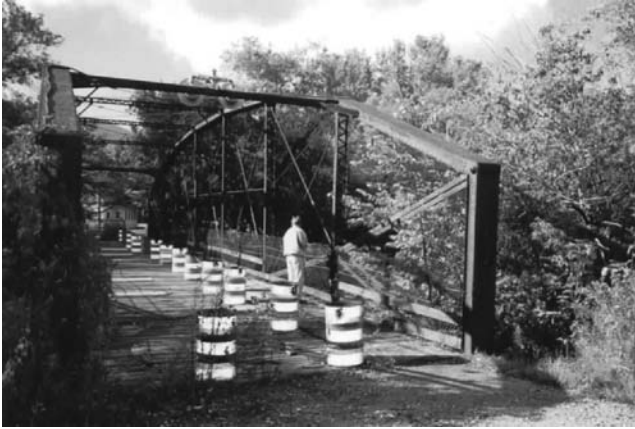
FIGURE 11.7 Berlin Iron Bridge Co. through truss bridge.
