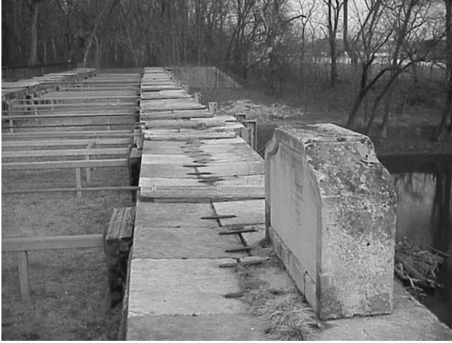
FIGURE 12.14 Iron cramps between coping stones at the Monocacy Aqueduct.
