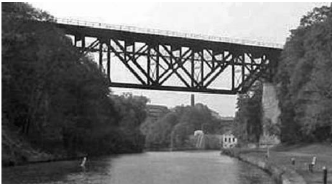
FIGURE 10.15 The Deck Truss at Lockport. (Source: A.K. Sloan.)
