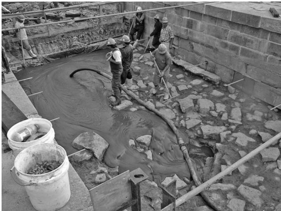
FIGURE 12.22 Flow grouting the prism floor at the Monocacy Aqueduct.
