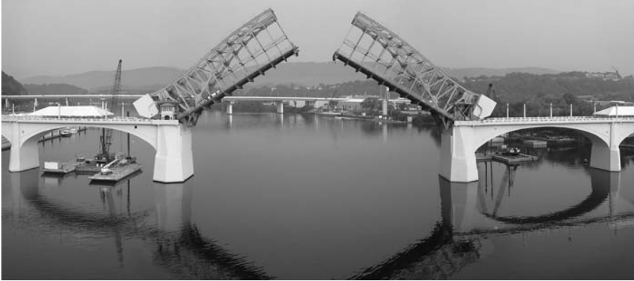
FIGURE 14.16 Market Street Bridge, Bascule Span, August, 2007. (Source: Ian Engstrom, Parsons Transportation Group Inc.)
