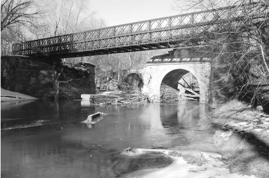
FIGURE 12.5 The Catoclin Aqueduct.
