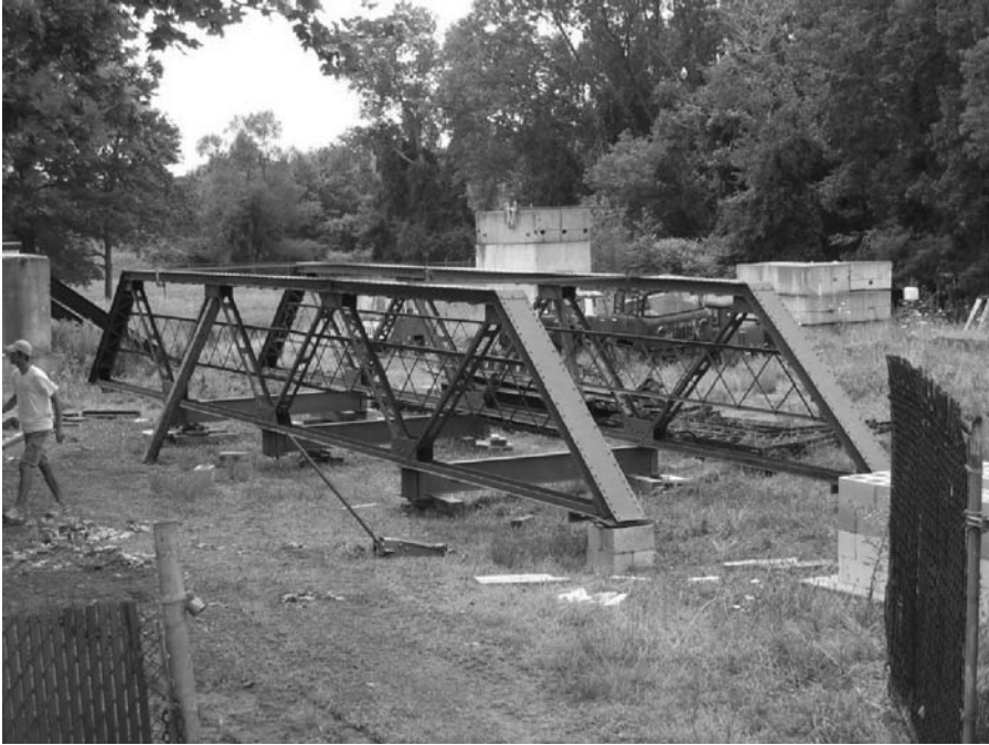
FIGURE 11.15 Trial assembly of Bridge No. 2.
