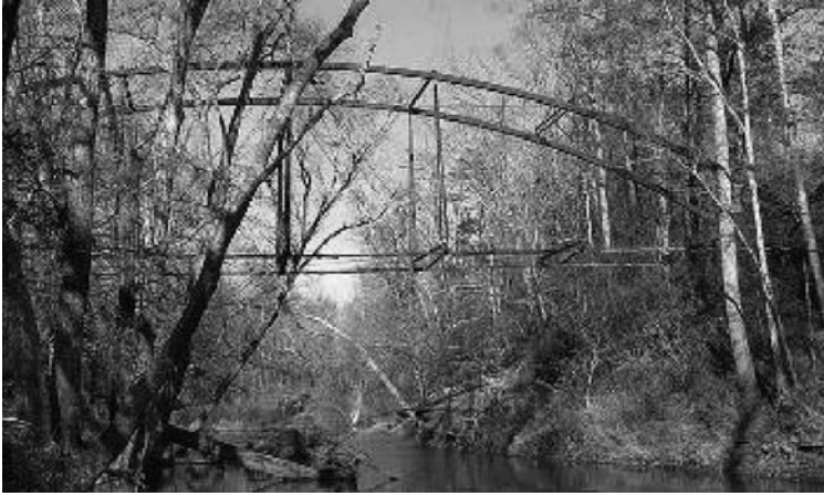
FIGURE 10.11 The Black Warrior Bridge awaiting relocation. (Source: K. Willis.)
