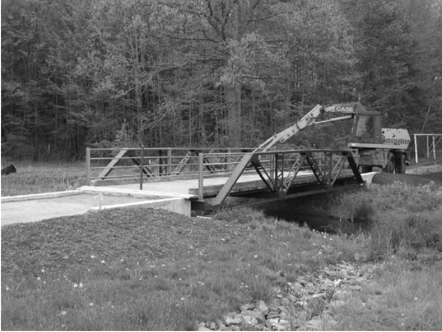
FIGURE 11.14 Bridge No. 1 at final location.
