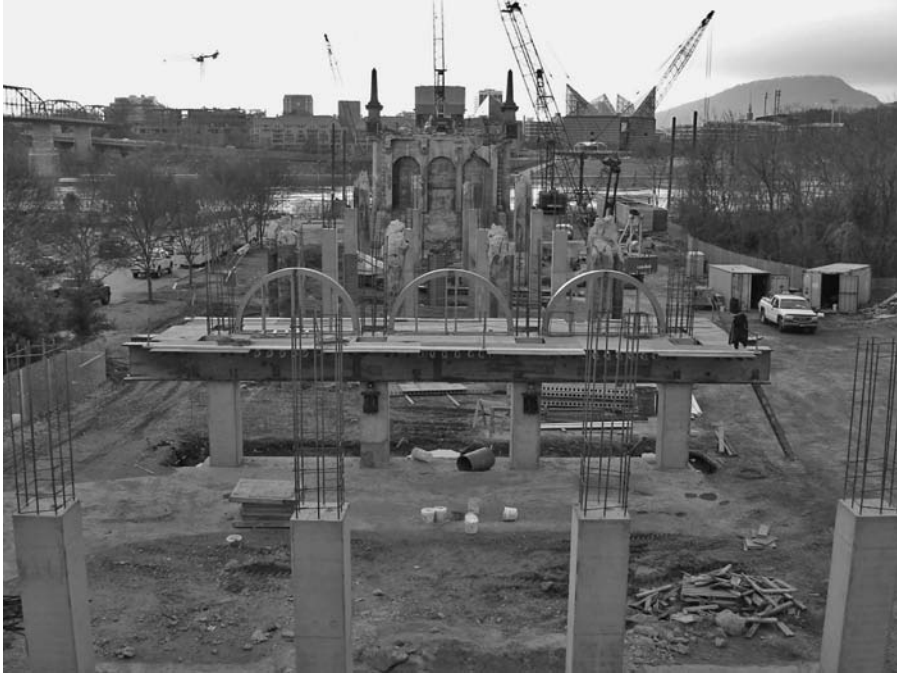
FIGURE 14.11 North Approach Spans, Reconstruction, 2005. (Source: Ian Engstrom, Parsons Transportation Group Inc.)
