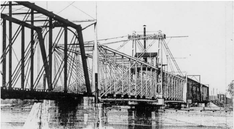
FIGURE 2.5 First swing span in closed position. (Courtesy of Clinton County Historical Society.)
