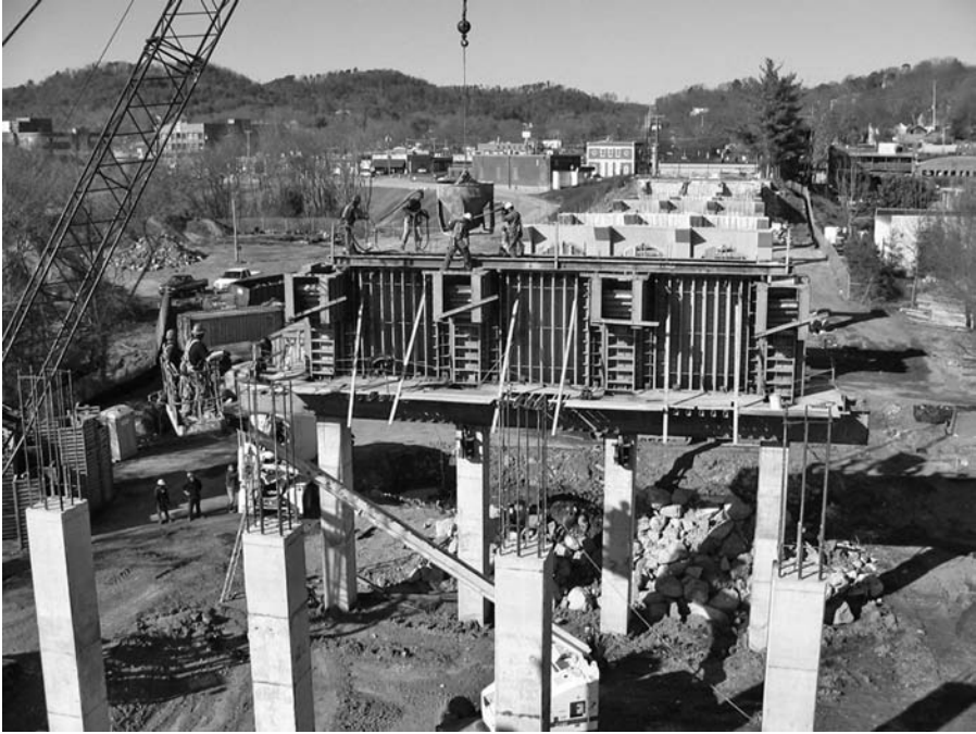
FIGURE 14.12 North Approach Spans, Reconstruction, 2005. (Source: Ian Engstrom, Parsons Transportation Group Inc.)
