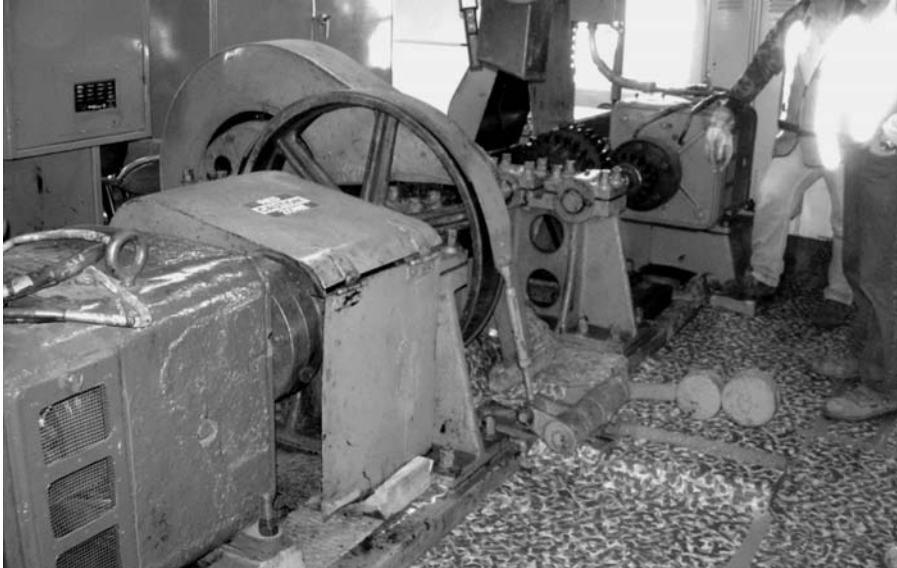
FIGURE 2.18 Primary span drive in Operator's House.
