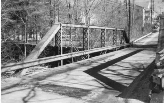
FIGURE 11.8 Bridge No. 7 while still in service.
