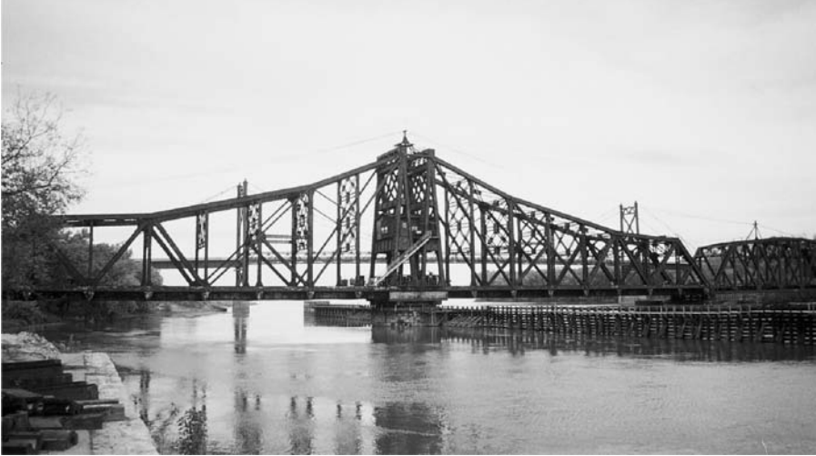
FIGURE 2.13 Third swing span in closed position.
