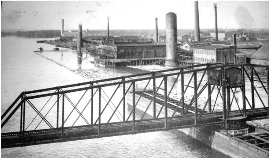
FIGURE 2.8 Second swing span in closed position. (Courtesy of Clinton County Historical Society.)
