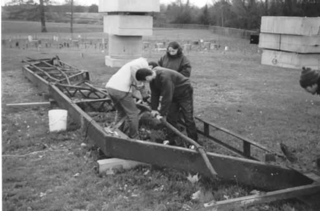
FIGURE 11.1 Students working to remove old handrail from Bridge No. 1.
