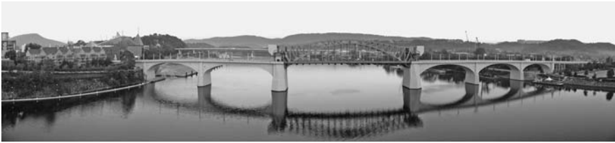
FIGURE 14.17 Market Street Bridge, September, 2007. (Source: Ian Engstrom, Parsons Transportation Group Inc.)
