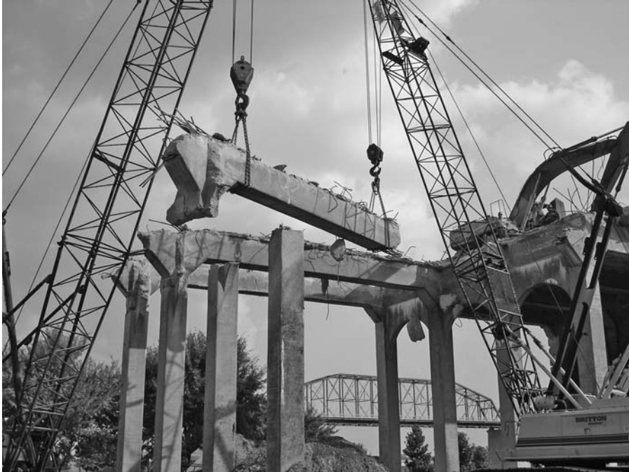
FIGURE 14.10 North Approach Spans, Demolition, 2005. (Source: Ian Engstrom, Parsons Transportation Group Inc.)
