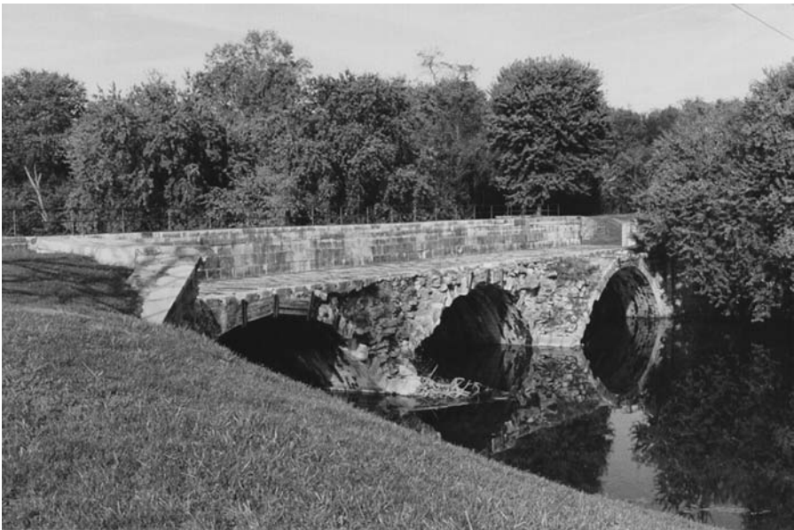
FIGURE 12.8 The Conococheague Aqueduct.
