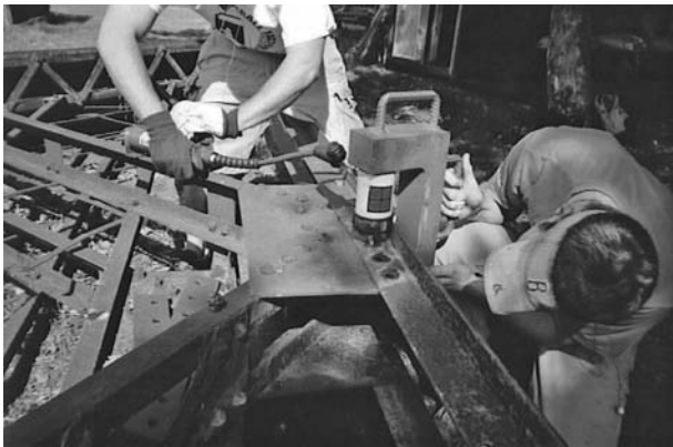
FIGURE 11.13 Students using portable hydraulic rivet press to remove rivets.
