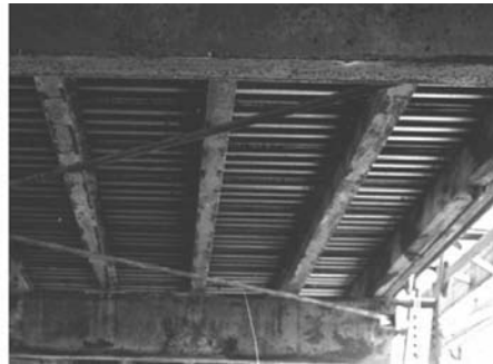
FIGURE 8.8 Rifle Bridge deck. The deck of (weathered) asphalt pavement on corrugated bridge deck on a combination of steel and timber stringers is similar to that of the Prowers Bridge.
