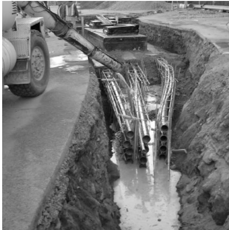
FIGURE 14-89 Duct bank being backfilled.
