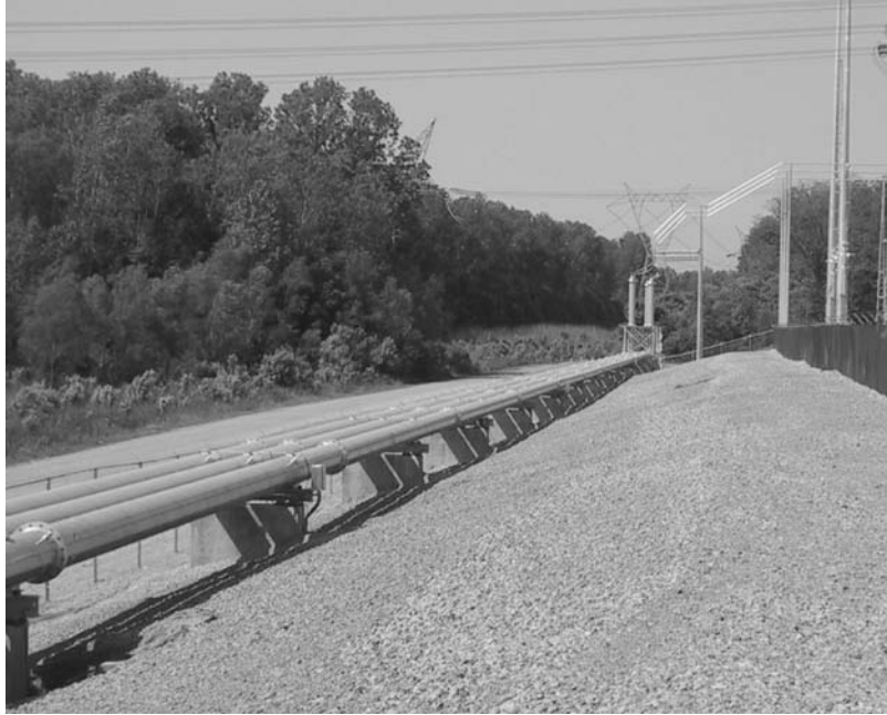
FIGURE 14-93 GIL installation. (Courtesy of CGIT/AZZ.)
