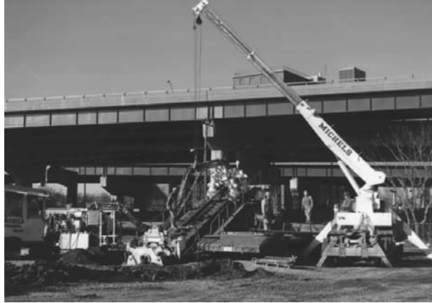
FIGURE 14-95 Guided boring equipment for a river crossing.
