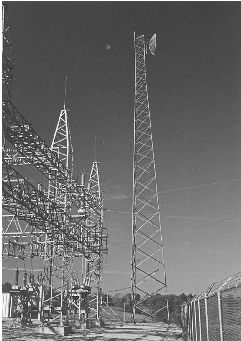
FIGURE 16-16 Microwave systems require large towers for line-of-sight paths between stations.
