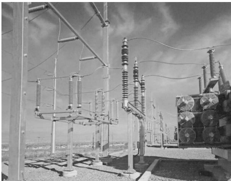
FIGURE 10-132 Substation transformer protective device. ( S&C Electric Company. )
