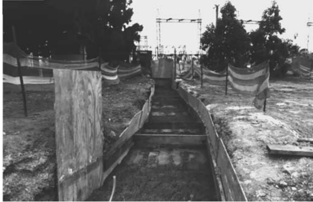
FIGURE 14-90 Cable trench with final FTB layer installed.
