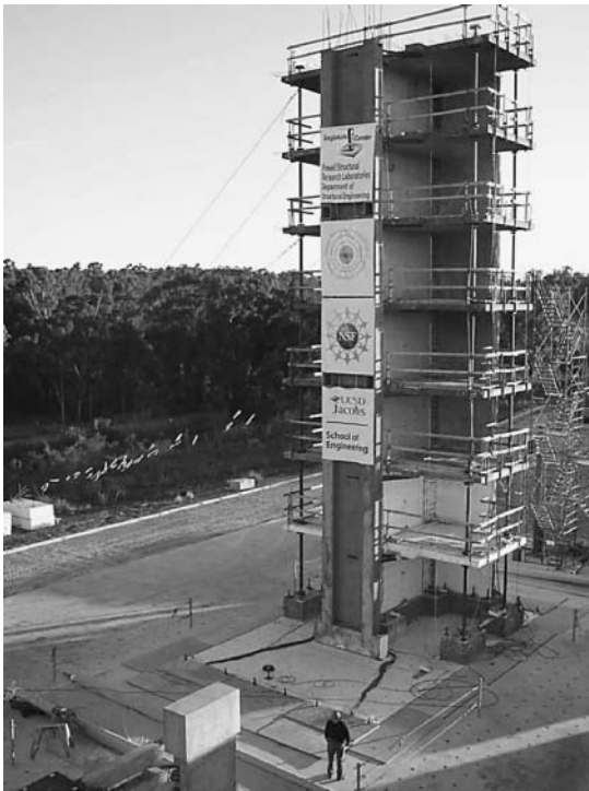
Figure 10.25 A seven-story wall building tested at UCSD ( http://nees.ucsd.edu/7Story.html )
