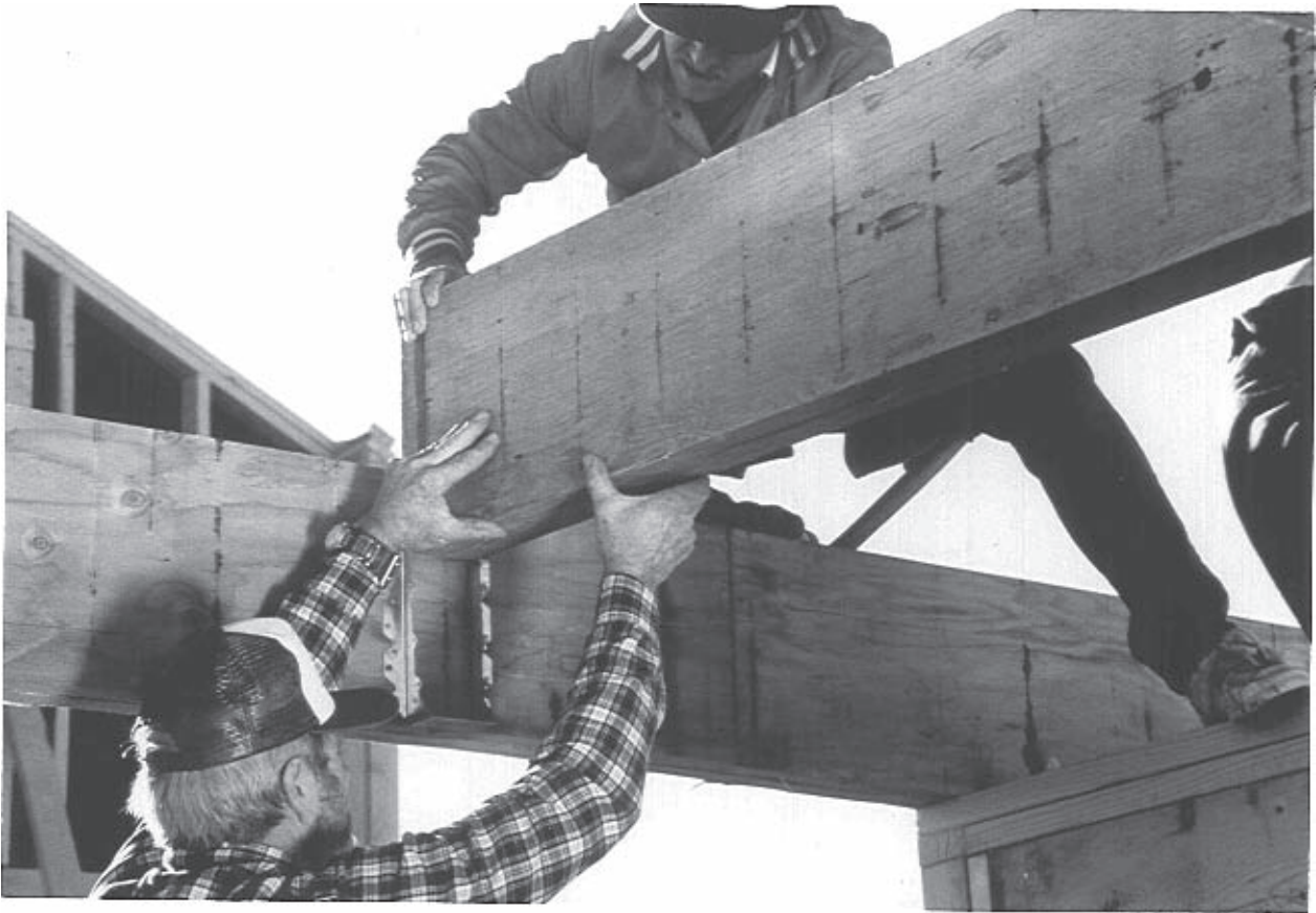
Figure 16-4. LVL (laminated veneer lumber) beams are popular, because they are strong and can be manufactured in any length and depth. Courtesy of Trus Joist Macmillan, A limited Partnership, Boise, ID.
