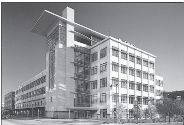
Figure 1-1(B). Commercial construction.
