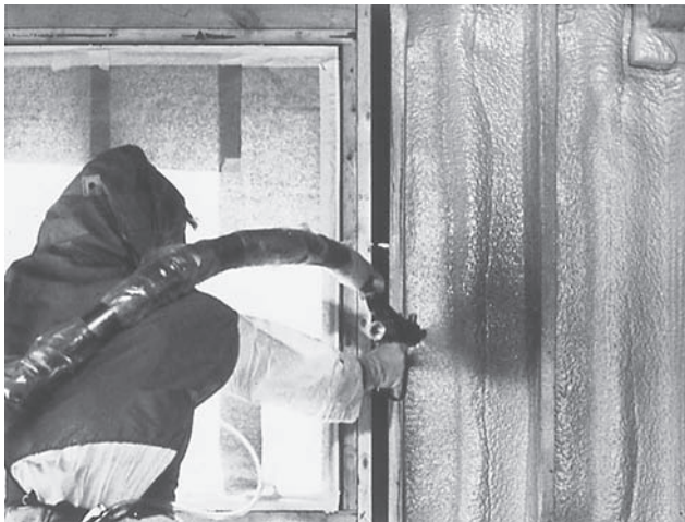
Figure 31–2. Foamed-in-place insulation. Courtesy of the Upjohn Company.
