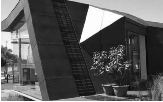
Figure 5.26 Built in 2005, this house in Australia uses the DSC-based Living Building Panel from Dyesol. (Photo courtesy: Dyesol).
