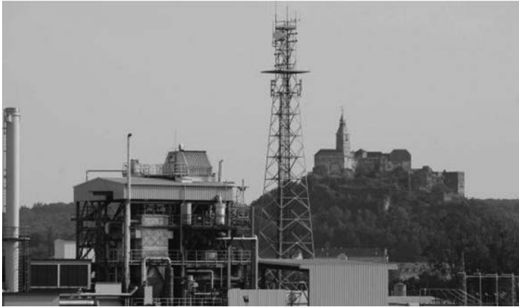
Figure 7.9 This plant in the Austrian town of Güssing makes fuel from wood. It uses steam to separate carbon and hydrogen from scrap lumber, then recombines the molecules to make a form of natural gas. (Photo courtesy: International Herald Tribune/Bianca Otero).
