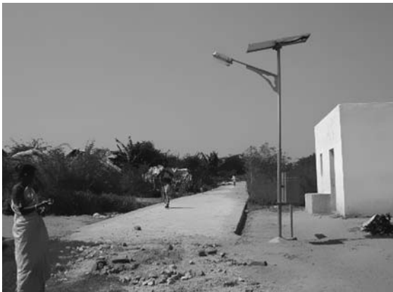
Figure 2.21 Street lighting installed in 2006 in the roads of Maharashtra, India, uses PV to power LED lamps at night. (Photo courtesy of Grameen Surya Bijlee Foundation, www.suryabijlee.com ).
