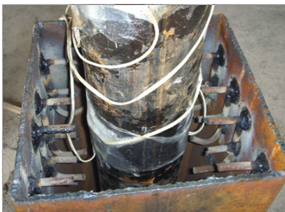
Fig. 5.4 Shear studs inside outer tube
