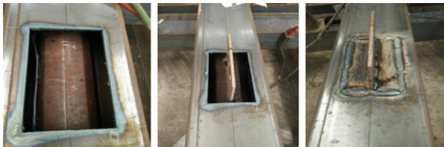
Fig. 7.2 Assembling process of the anchorage web
