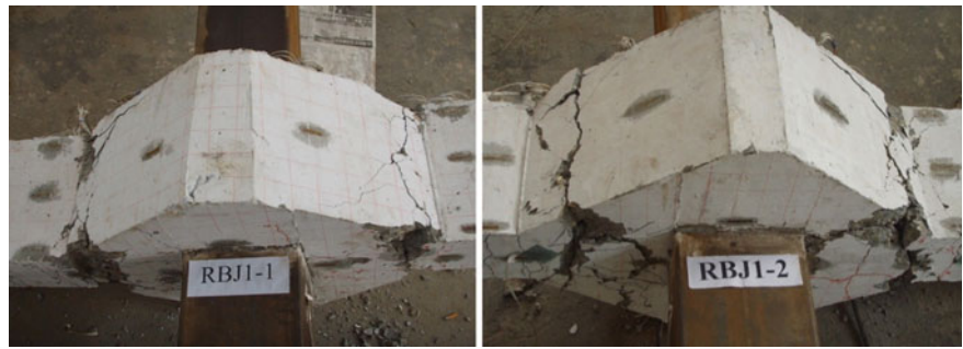
Fig. 5.6 Damage at failure
