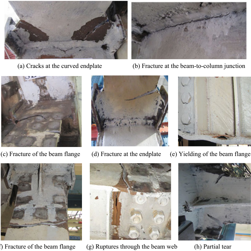
Fig. 6.9 Typical failure patterns of the specimens
