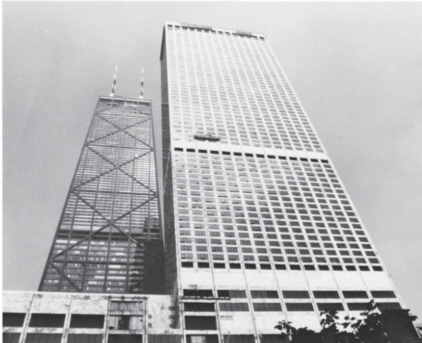
Water Tower Place, Chicago, Illinois, tallest reinforced concrete building in the United States (74 stories, 859 ft).
