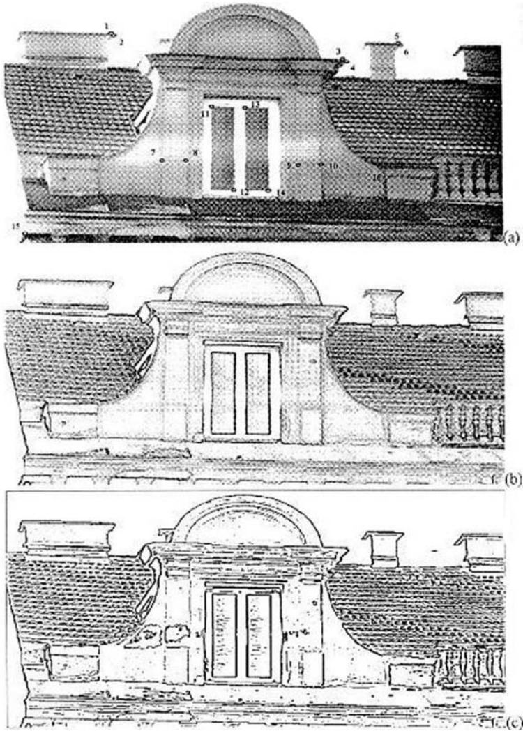
FIGURE 17.6. (a) Facade original; (b) after applying histogram equalization and Sobel-operator; (c) after applying thresholding.
