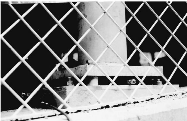
Figure 1.11 Flat jacks fitted under each new column.
