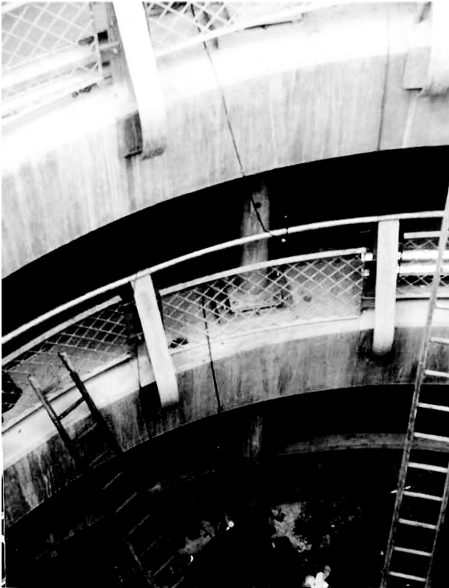
Figure 1.10 Additional steel columns.
