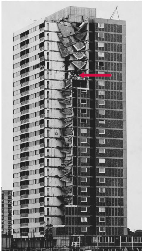
Figure 6.10 Progressive collapse showing point of explosion. (Ronan Point building collapse, May 16, 1968, London. Courtesy of Building Research Establishment.)
