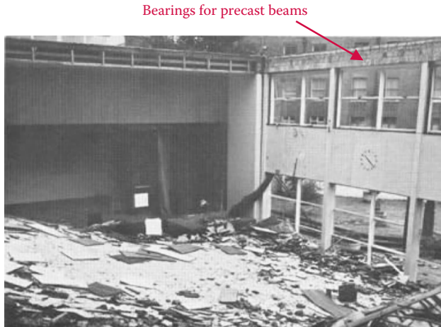
Figure 6.5 Assembly hall showing edge beam that supported the precast beams. (From Scott, G.A., Building Disasters and Failures , Construction Press Ltd., Lancaster, 1976. With permission.)
