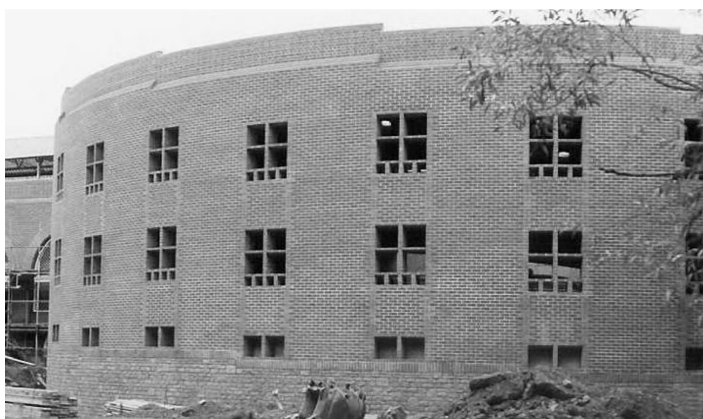
Figure 1.9 Car park with circular ramps.
