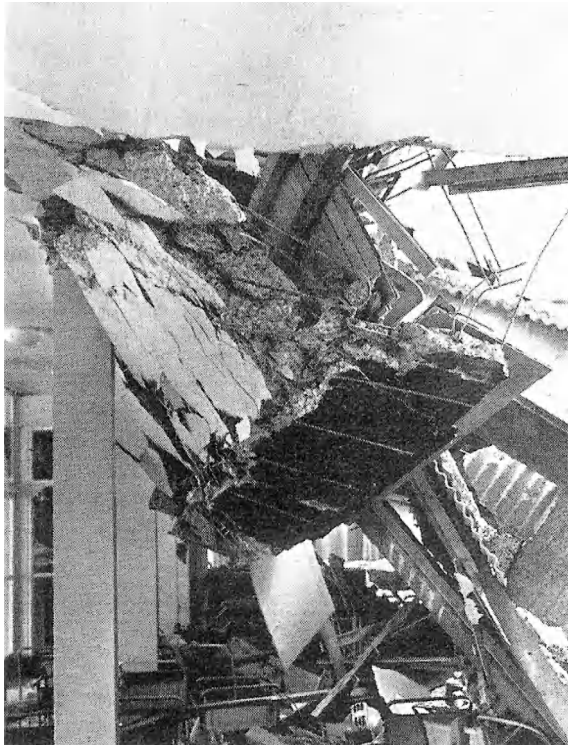
Figure 6.6 Part of roof that collapsed on chairs below. (From Scott, G.A., Building Disasters and Failures , Construction Press Ltd., Lancaster, 1976. With permission.)
