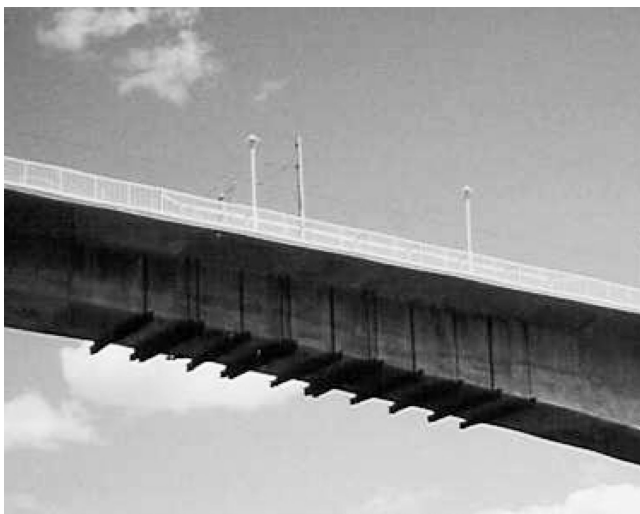
Figure 3.5 Temporary repair work on bridge.
